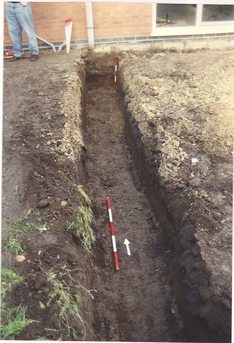
PI. 3 Western wall footing at the southern side of the building, facing north.
