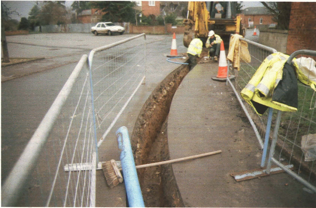
Plate 1 - General view of the pipeline trench along Church Street
