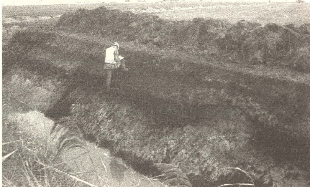
Plate 2 : Looking northeast, along the route of the Bourne-Morton Canal towards Morton Fen. The sequence of deposits continues either side of the recorded section.
