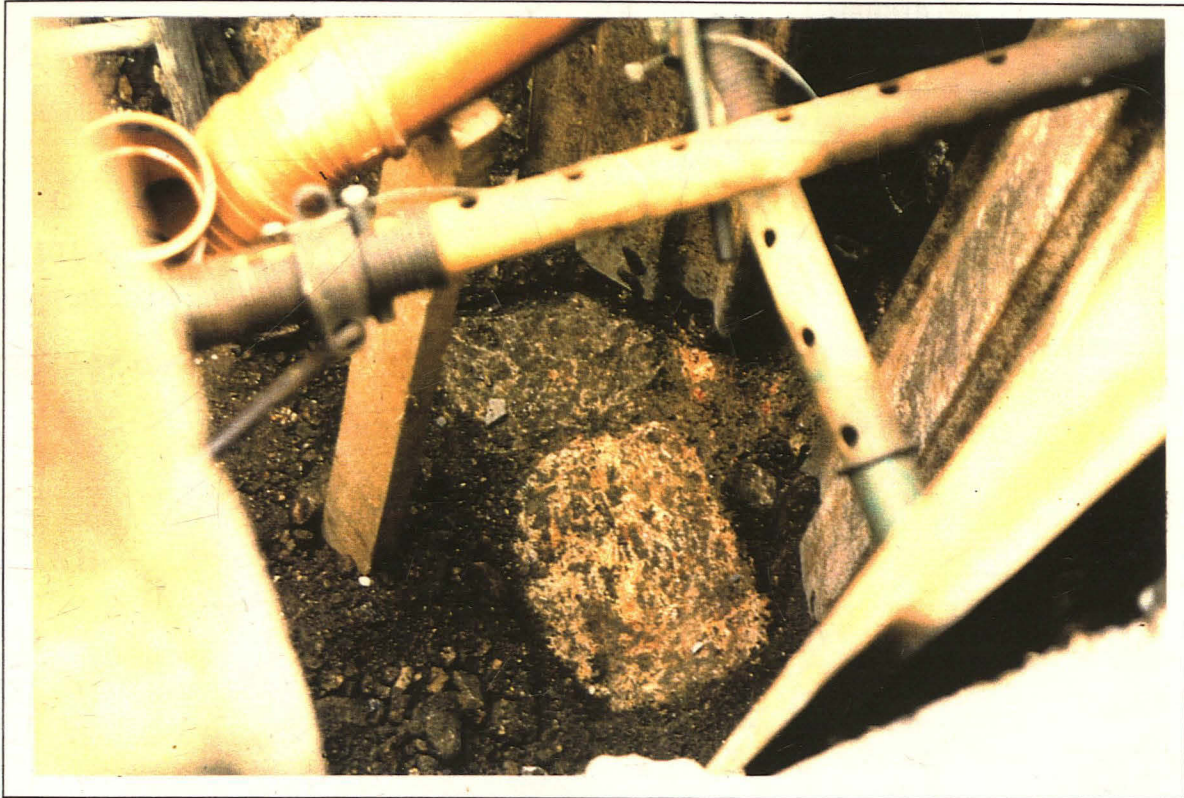
Plate 1: Overhead view of paving slabs in base of trench
