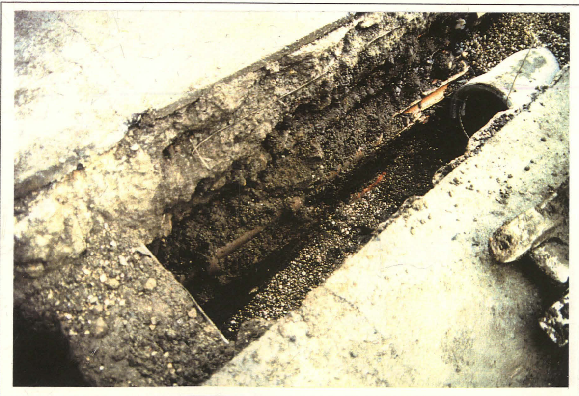
Plate 2: Extent of modern disturbance, St. Marks Street sewer connection (UCLA95)
