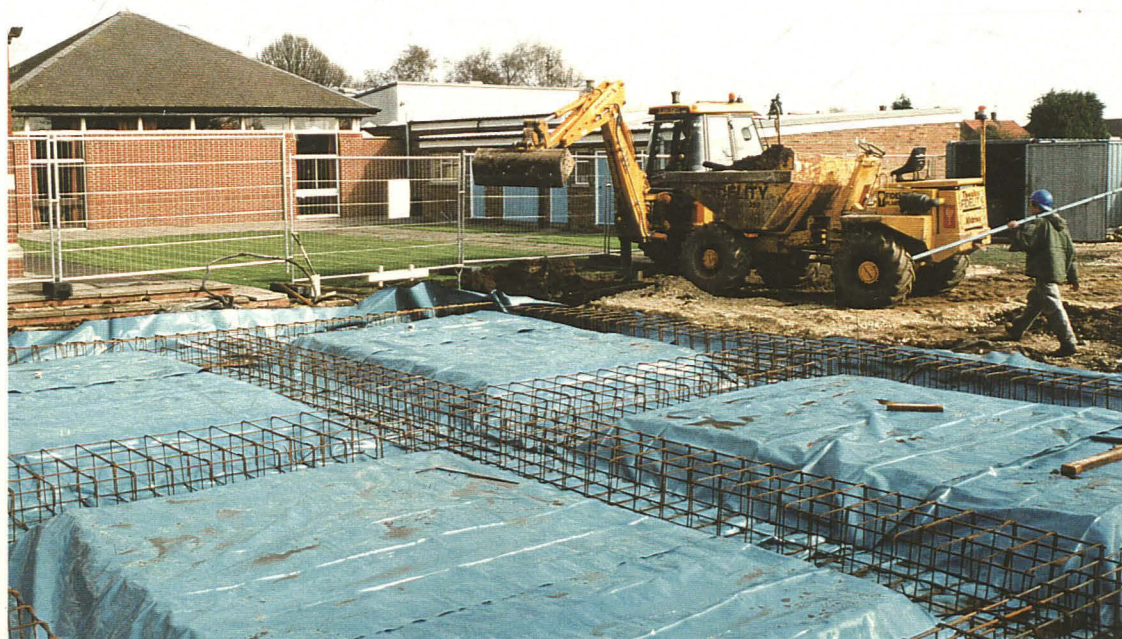
P2. General view looking north-west, during construction of foundation raft
