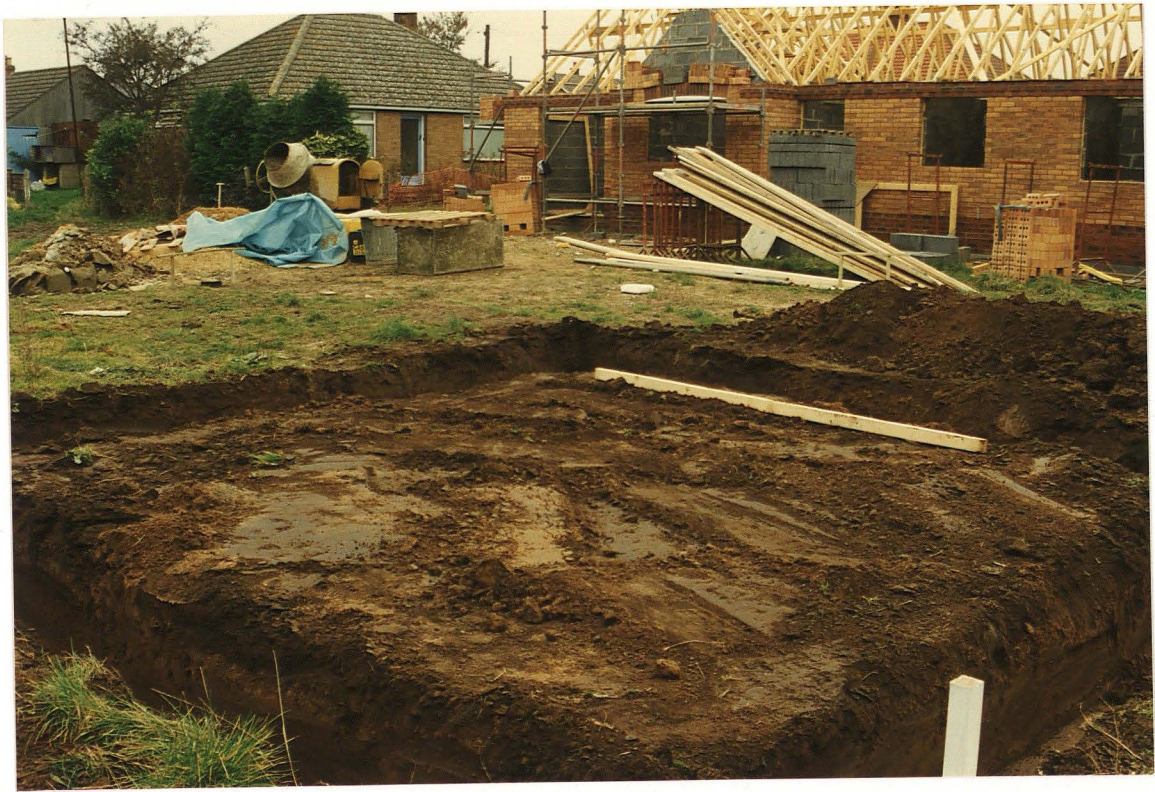
Pl. 3 Location of the garage to west of Plot 10 (looking NE).
