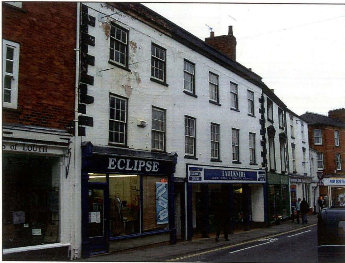
Plate 1 (left): general view of the frontage of 91, 93 and 95 Eastgate, Louth.
