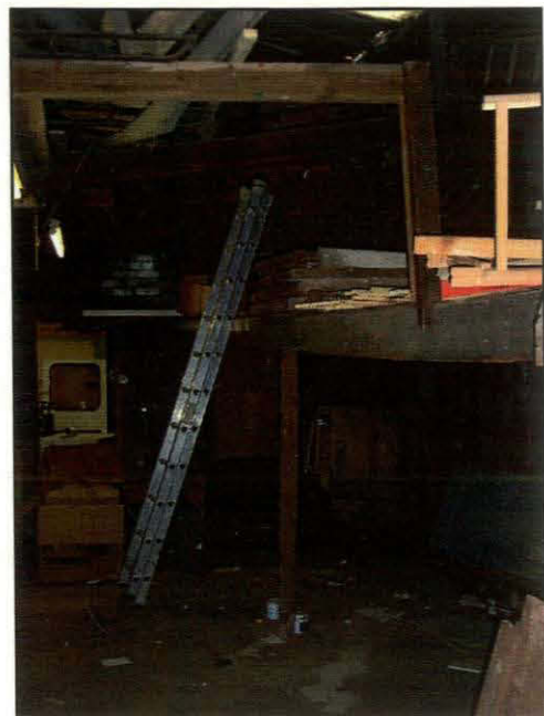
Plate 13 (above): Interior view of building 2, looking north.
