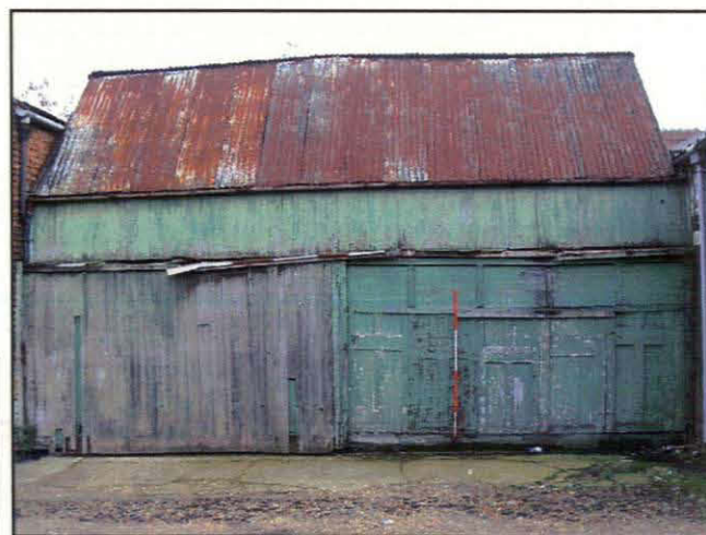
Plate 7 (right): West facing elevation of building 2, looking east.
