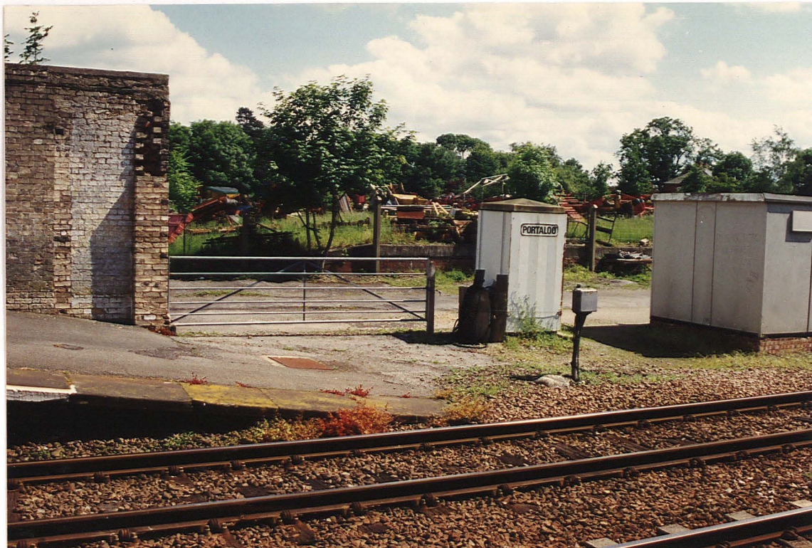
Pl. 8 Railway sidings and former coal yard used for equipment storage to south of goods shed (looking east).
