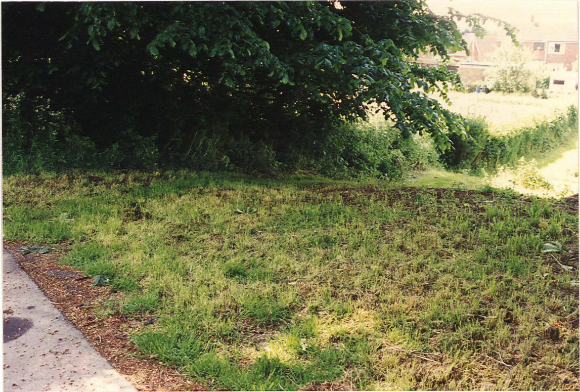
Pl. 4 Earth embankment raising the station from the former ground level to the west (looking SW from station access, outside the application site).
