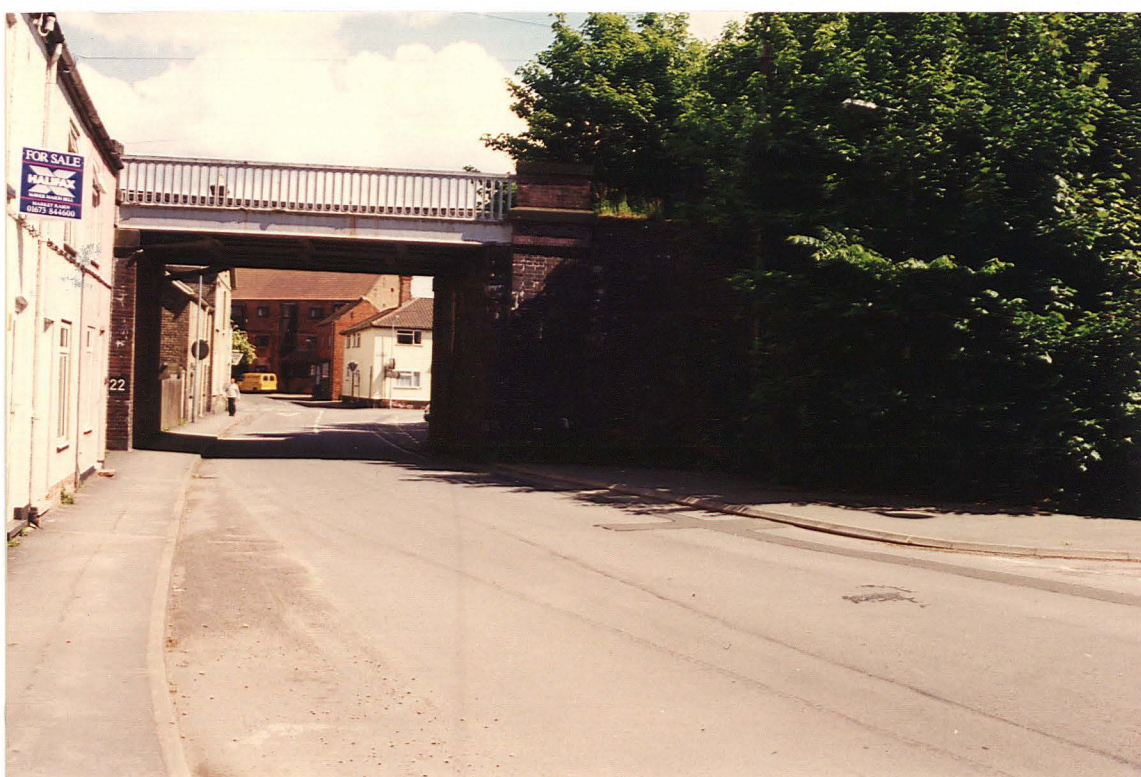
Pl. 9 Railway bridge over Chapel Street showing the height of the track compared with adjacent properties (looking east across Linwood Road to Serpentine Street).
