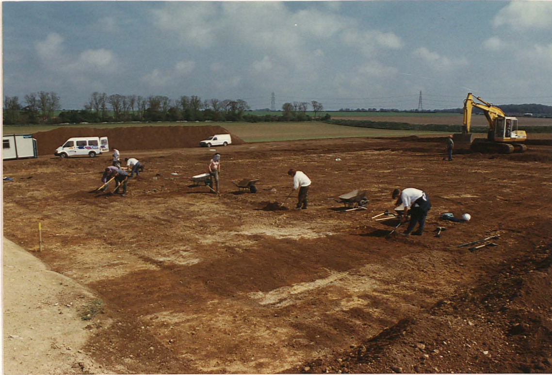
Plate 1: Removing the modern ploughsoil; looking NE
