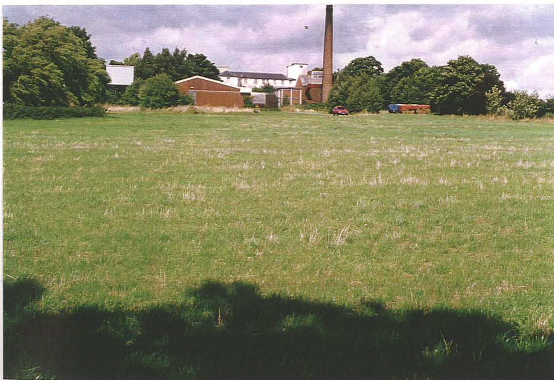
PI. 7 The eastern side of the hospital site, looking north from the rear field, with boiler house and infirmary beyond.
