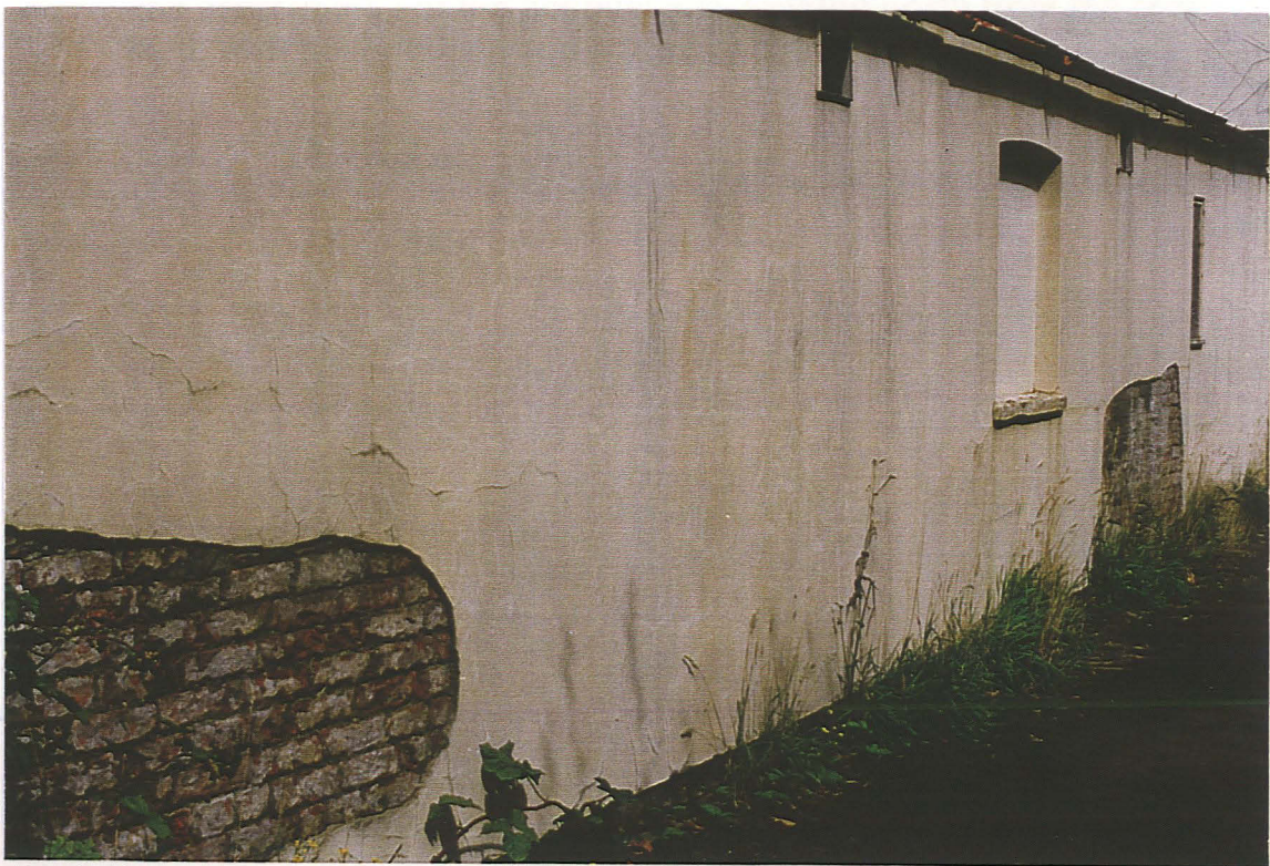
Pl. 5 Exposed brickwork at the rear of the House of Industry block.
