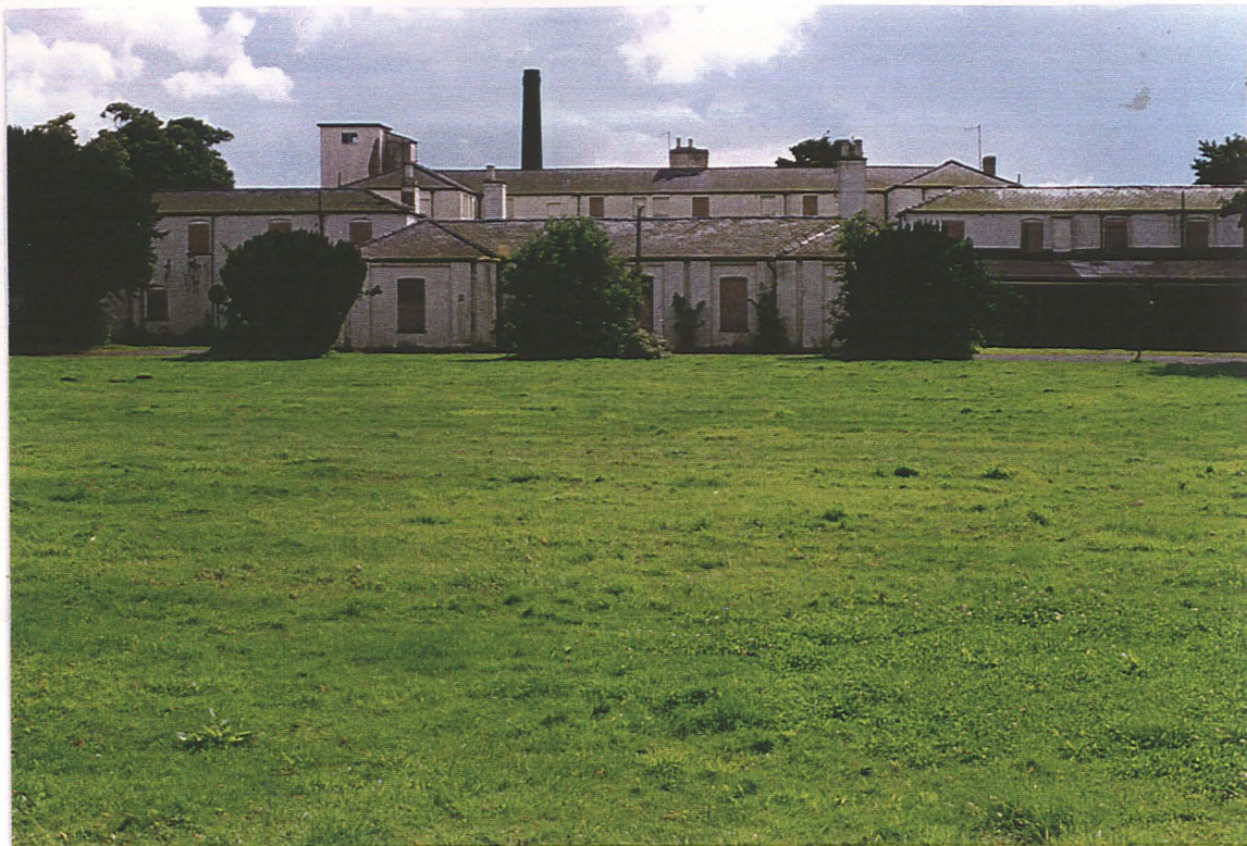
Pl. 2 Buildings at the front of the hospital site (looking south across the lawn area).
