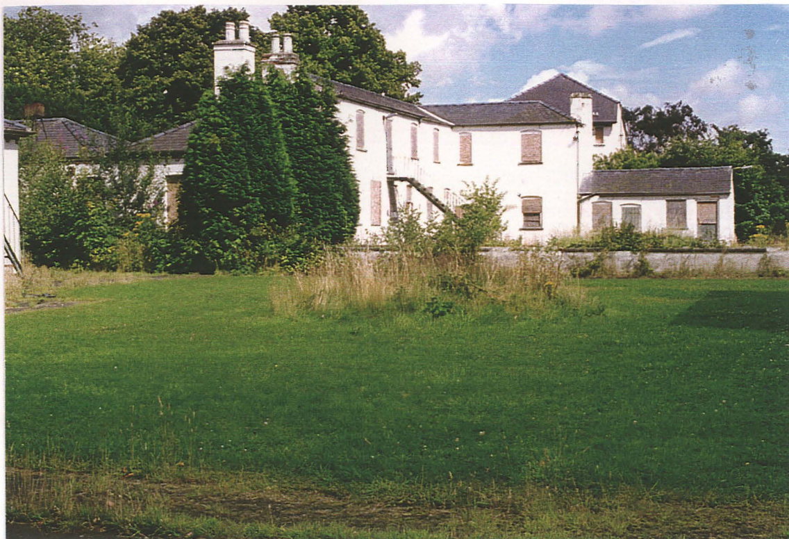
PI. 6 Rear elevation of the Caistor Union Workhouse buildings at the front of the site (looking NE across the courtyard).
