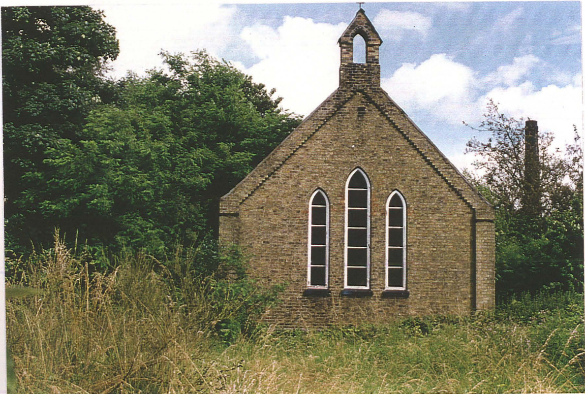
Pl. 9 Rear elevation of St. Lawrence's chapel and overgrown burial ground (looking east).
