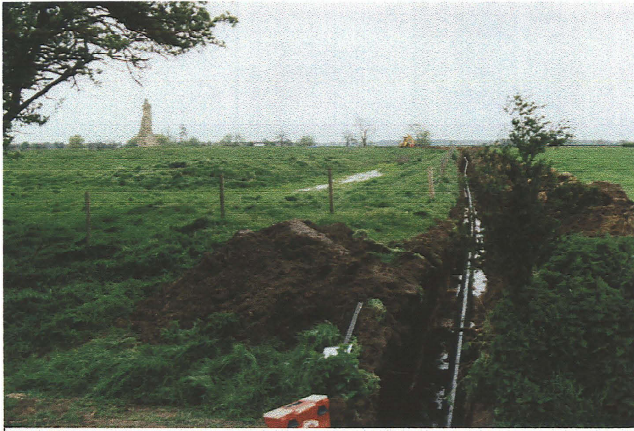
Plate 1 : General view of site looking northeast, showing pipe trench.
