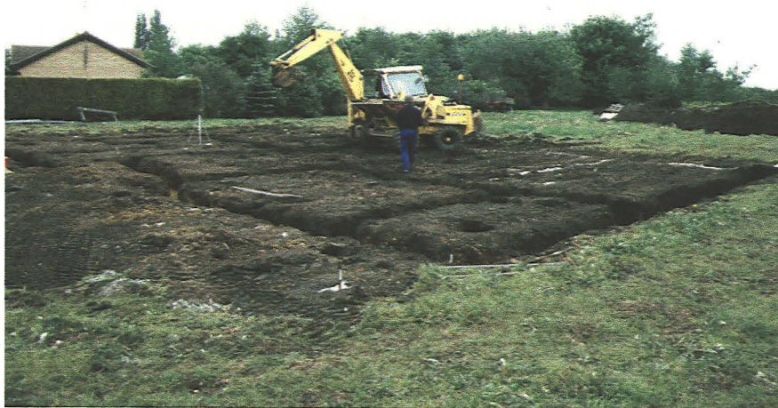
Plate 1: General site view.
