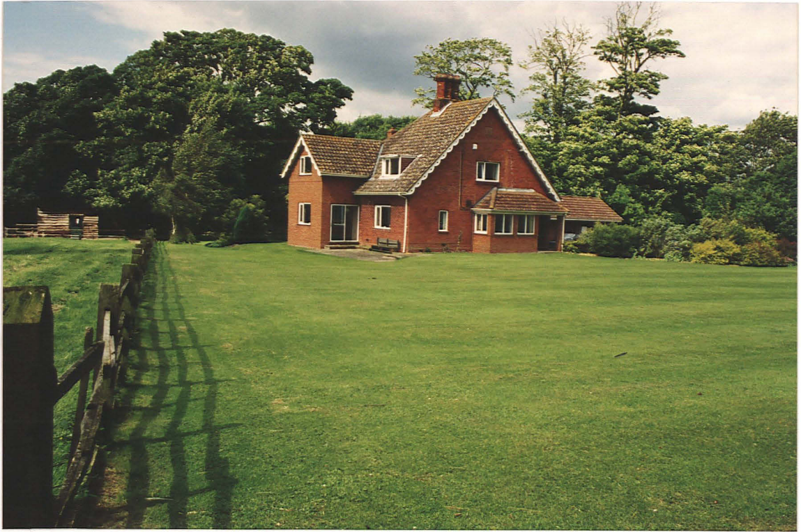
Pl. 5 Former gamekeeper's cottage (New Farm Crops offices) to east of survey area with landscaped lawns.
