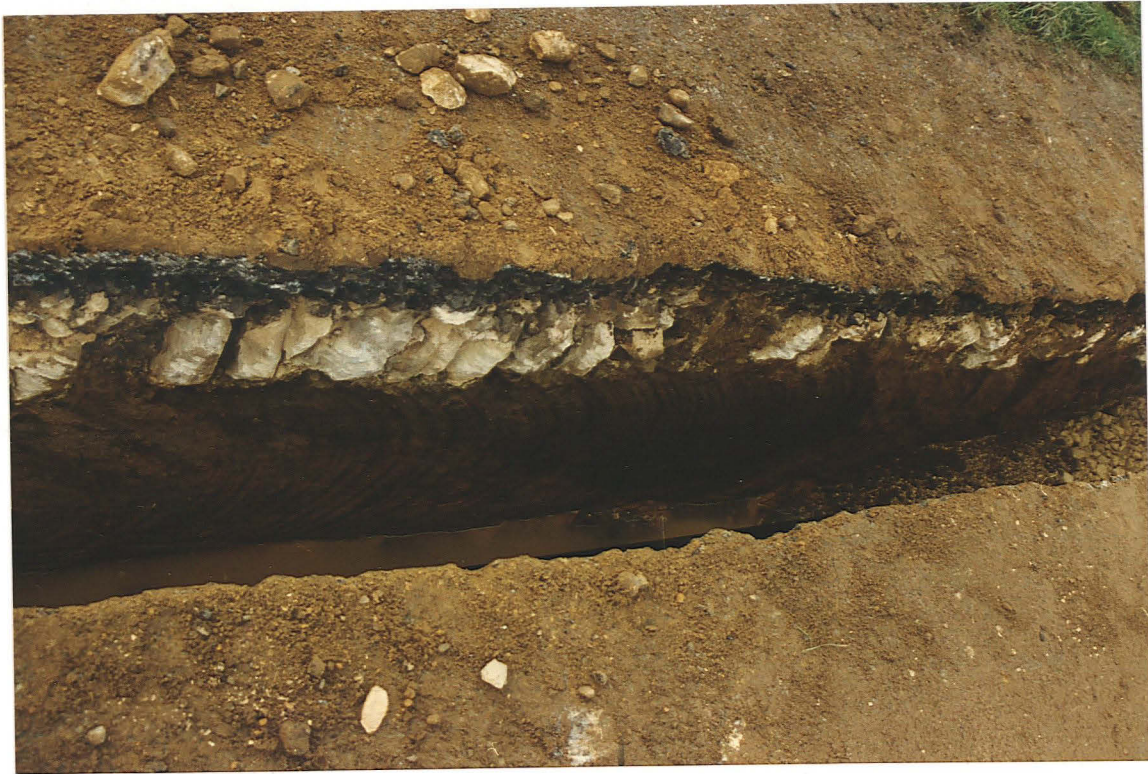
PI. 16 Pitched limestone rubble used for road edge consolidation, 7F.
