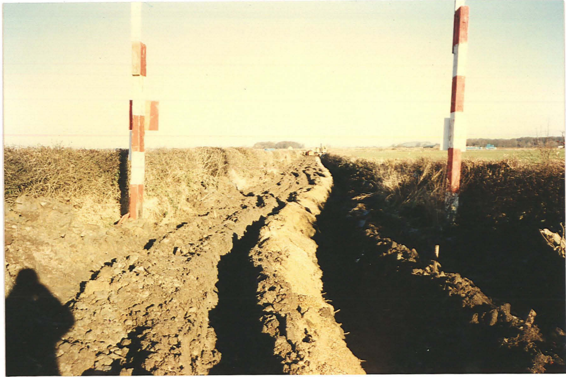
Pl. 10 Green lane to south of Cliff Lane (looking north). The pipe trench was excavated through modern rubble at the eastern side of the track.
