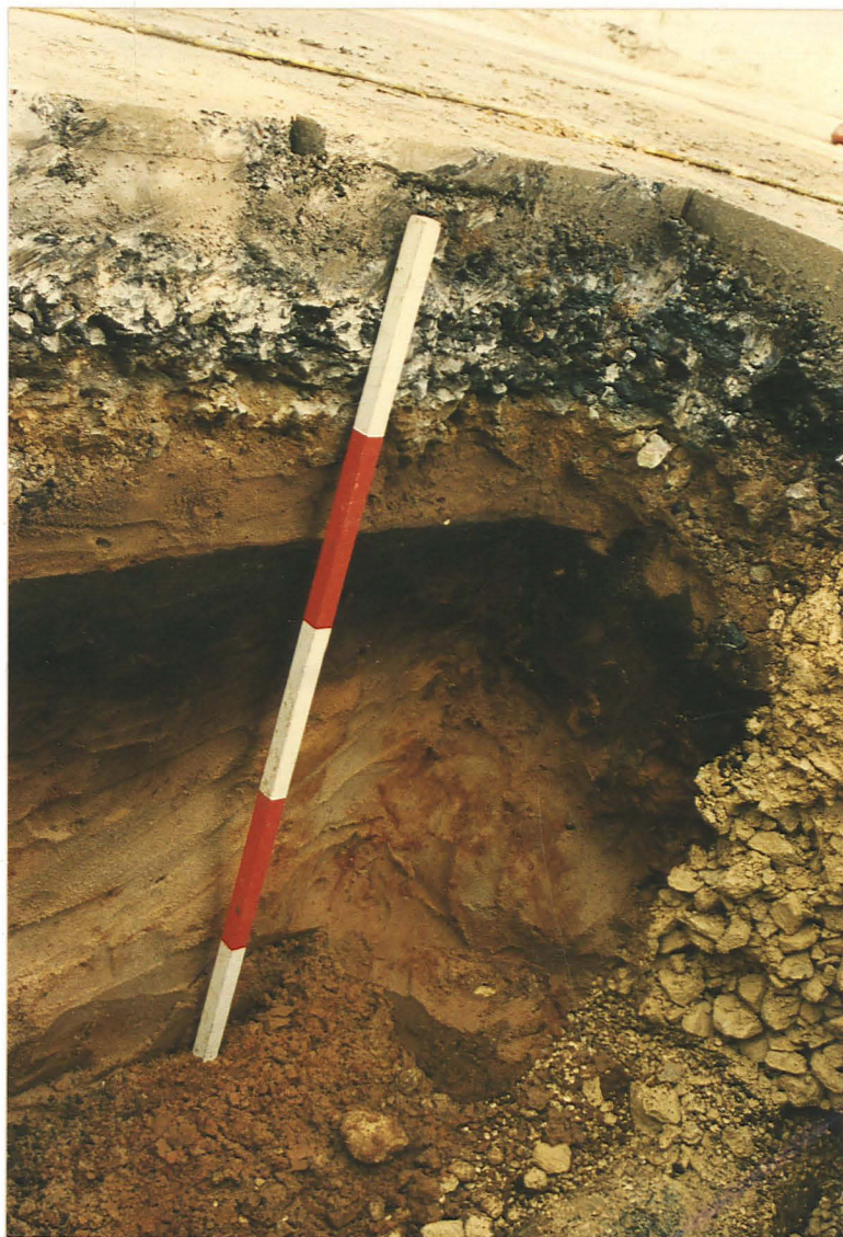
Pl. 12 Pipe trench section at Sand Lane/Barkston Road junction (7A), showing sand bedding for the road sealing black sand from a buried ground surface or ditch fill (scale divisions 0.2m).
