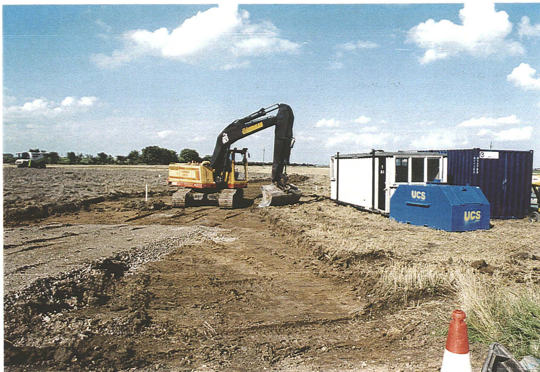
P1. General view of site showing topsoil stripping, looking north
