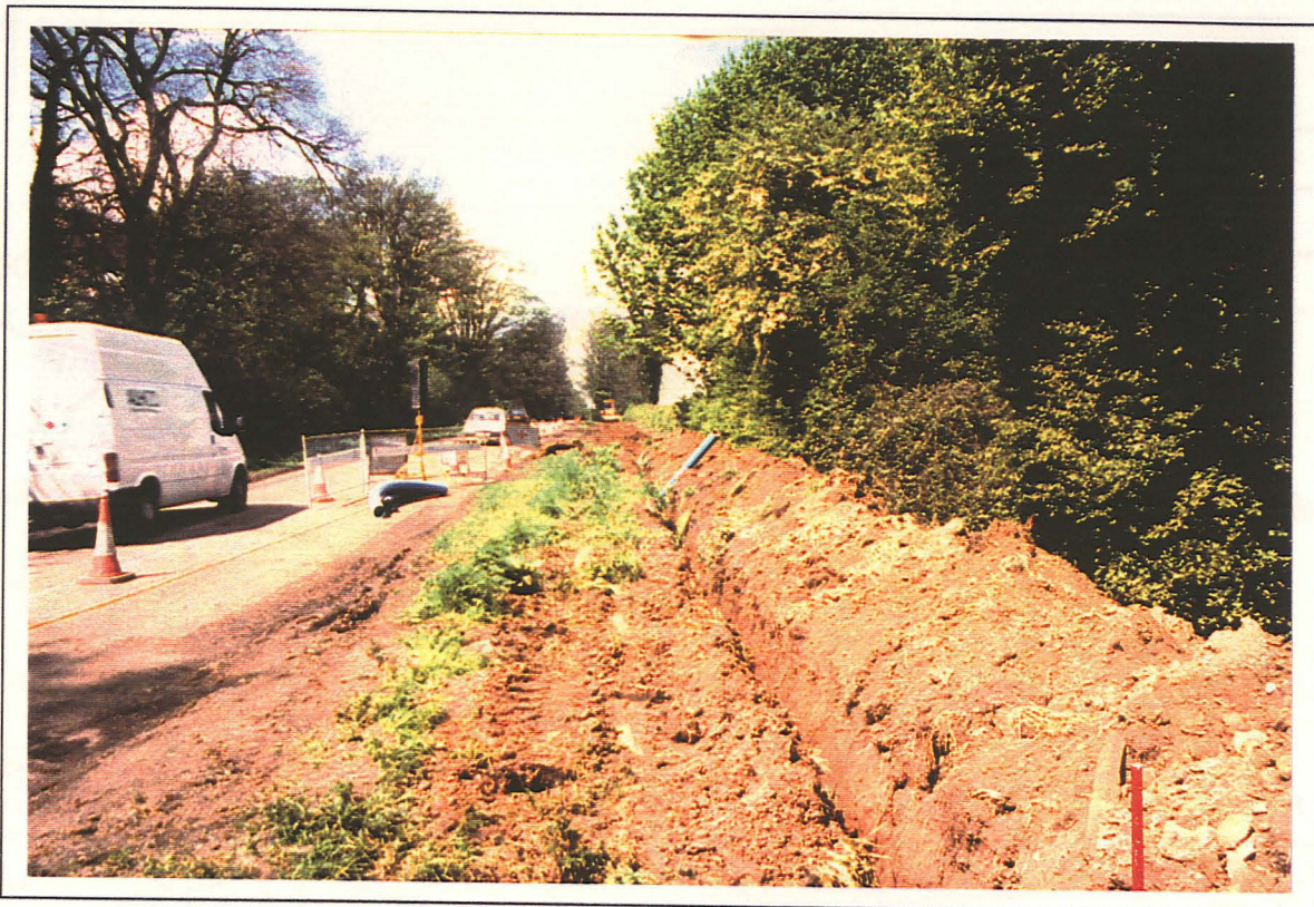
Plate 1: General view of trench - looking north-west
