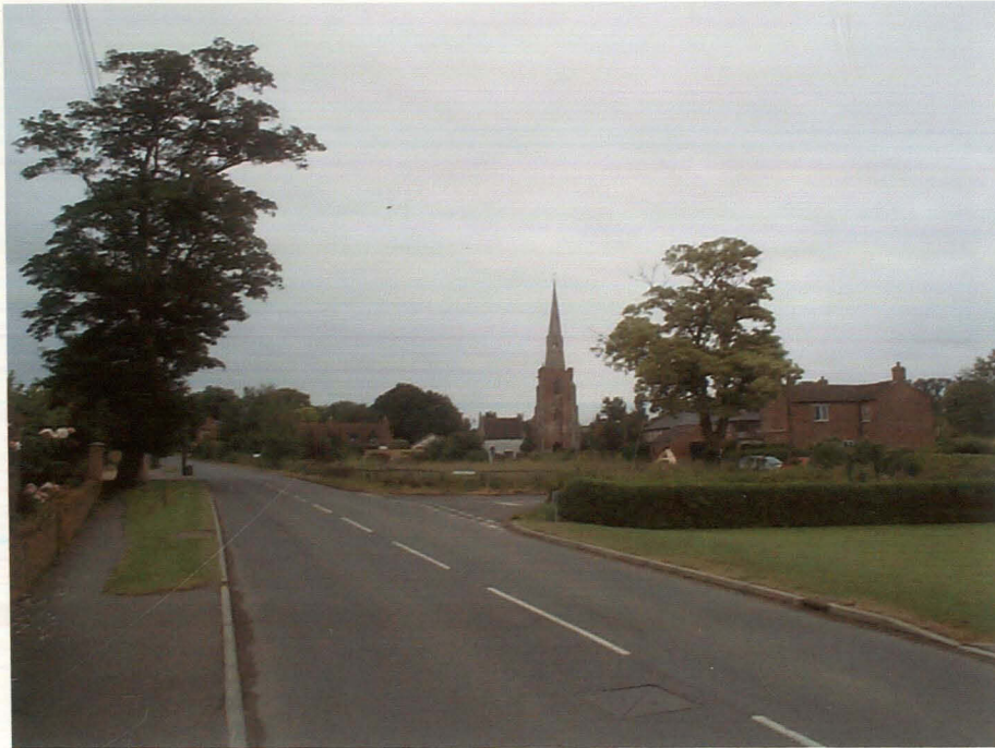
Plate 1 General view of Tydd St. Mary conservation area, looking east along Common Way
