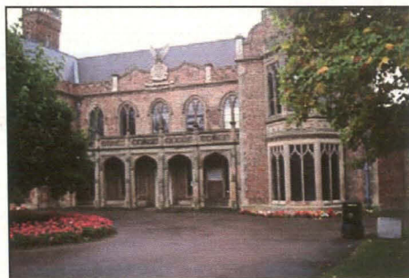
Plate 15. The western façade.
