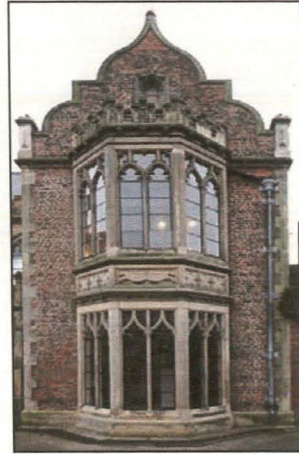
Plate 8. Oriel window on the western façade
