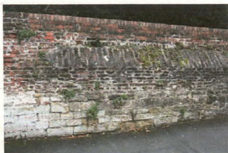
Plate 6. Part of the perimeter wall.
