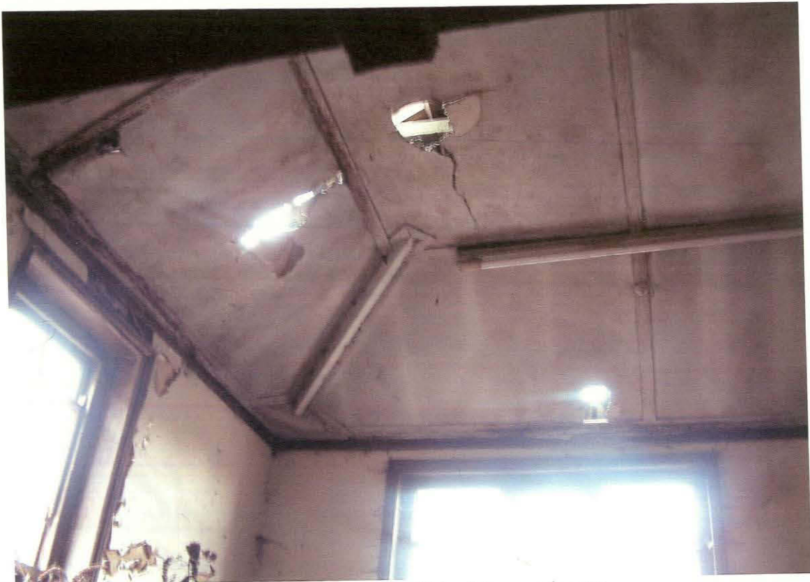
Plate 15. Showing ceiling in First floor room D looking south east
