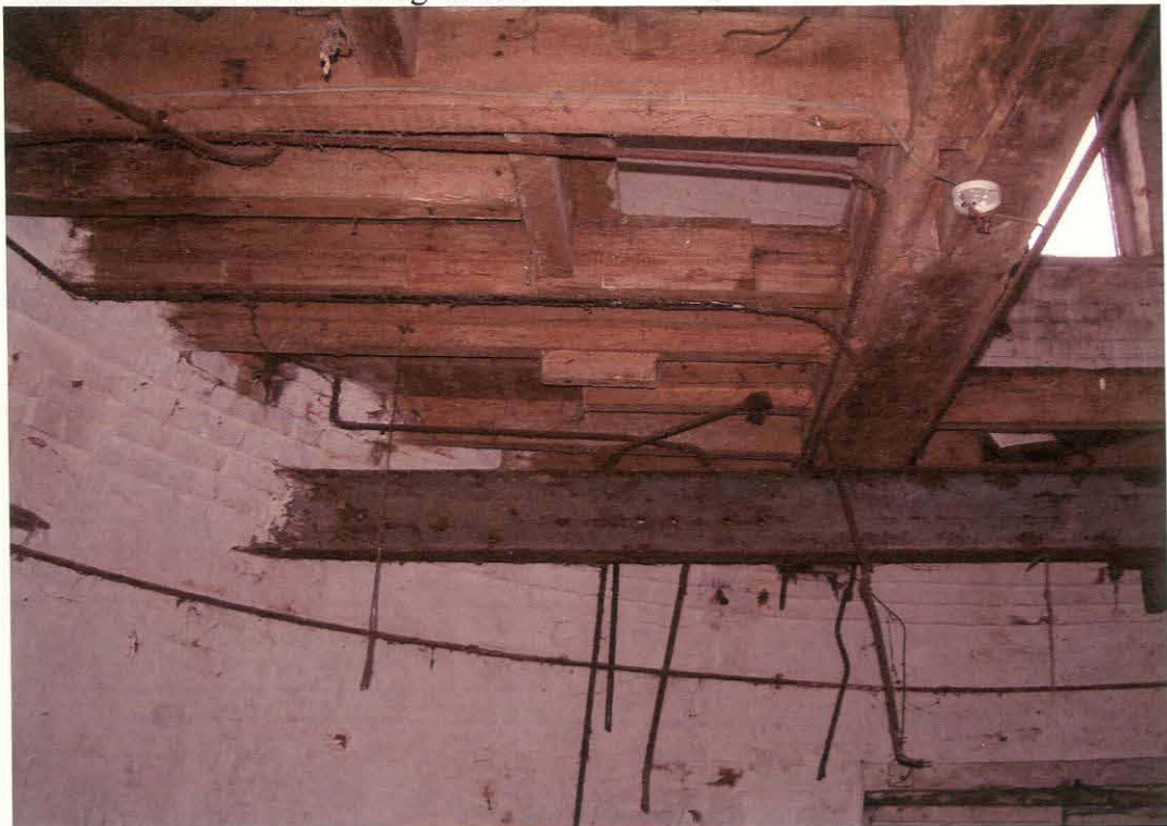
Plate 24. Ground floor South showing ceiling timbers & R.S.J.
