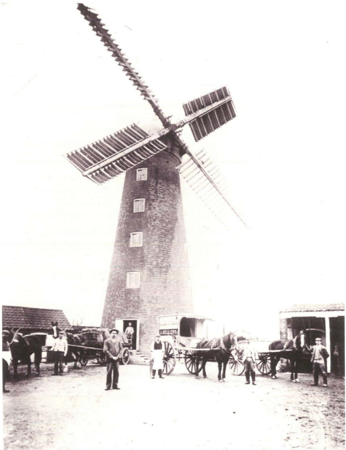
Plate 31. Mill in original state (Undated, probably around late 19 th c- early 20 th Century).
