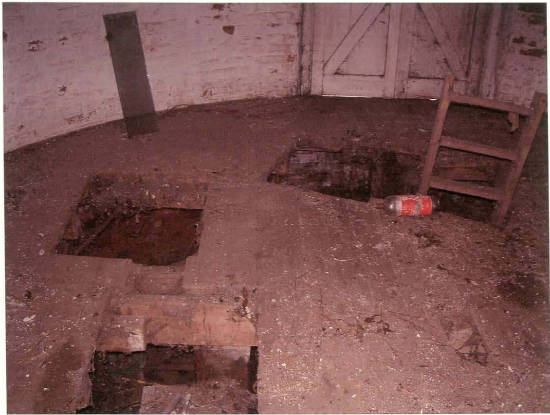
Plate 23. Ground floor looking south.
