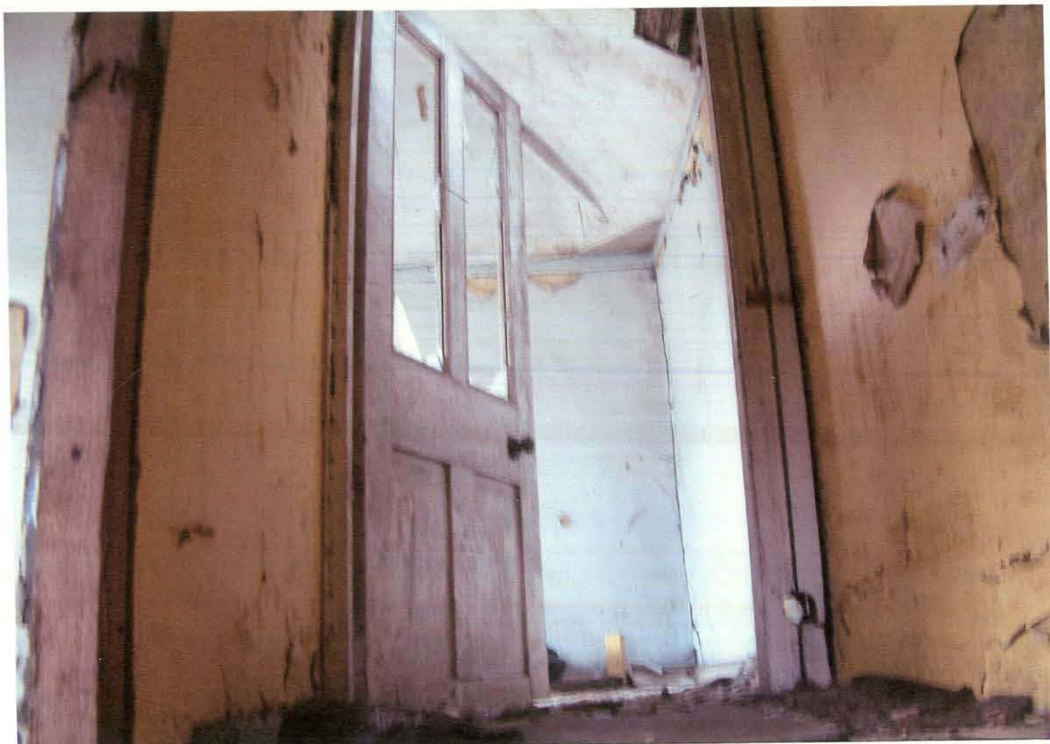
Plate 13. Staircase into first floor room C
