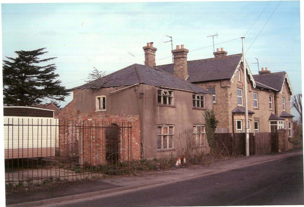
Plate 1. Millers Cottage north east view.
