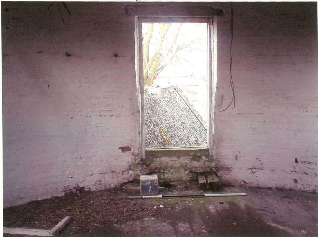
Plate 26. North view first floor showing access doorway.
