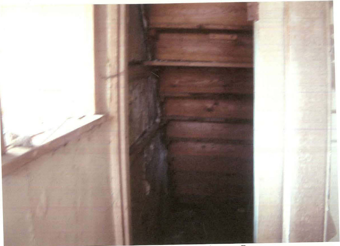
Plate 11. Ground floor Showing underside of staircase in room B.
