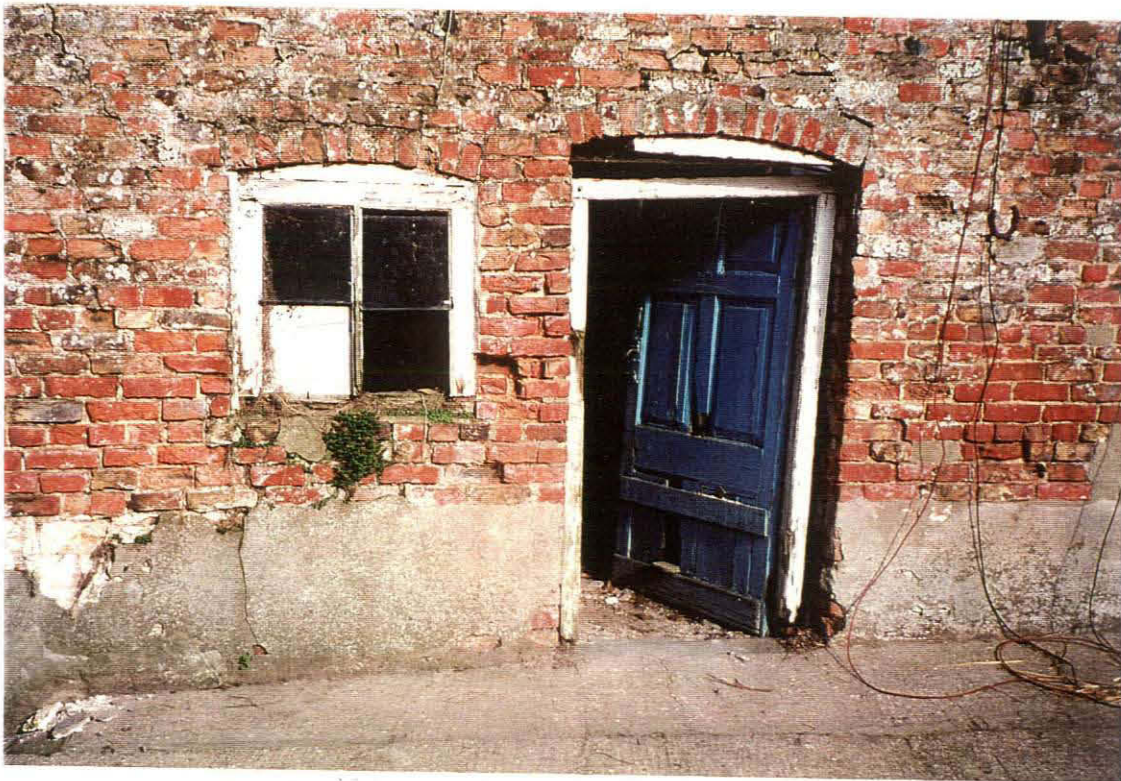
P. 6 Construction of utility, looking N.
