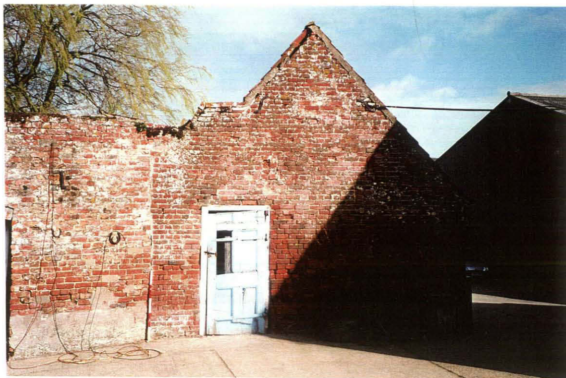
P.1 South wall of garage outbuilding, looking N.
