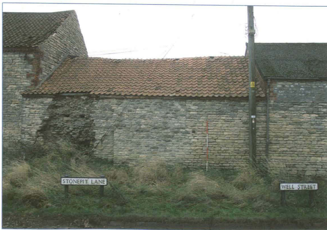
Plate 4: North elevation of Building 2, showing exposed rubble core and blocked doorway. Looking south.
