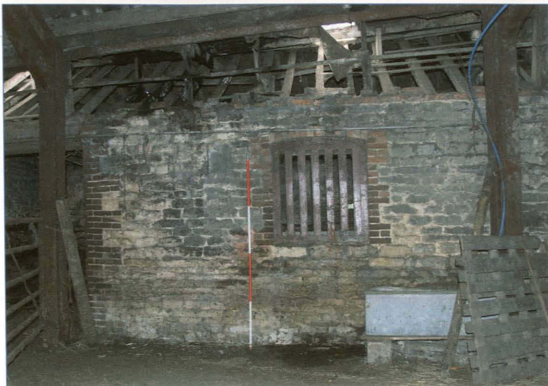
Plate 5: South elevation of Building 2, showing the window and part of the entrance to the west. The saw tooth brickwork is likely to be an original feature.
