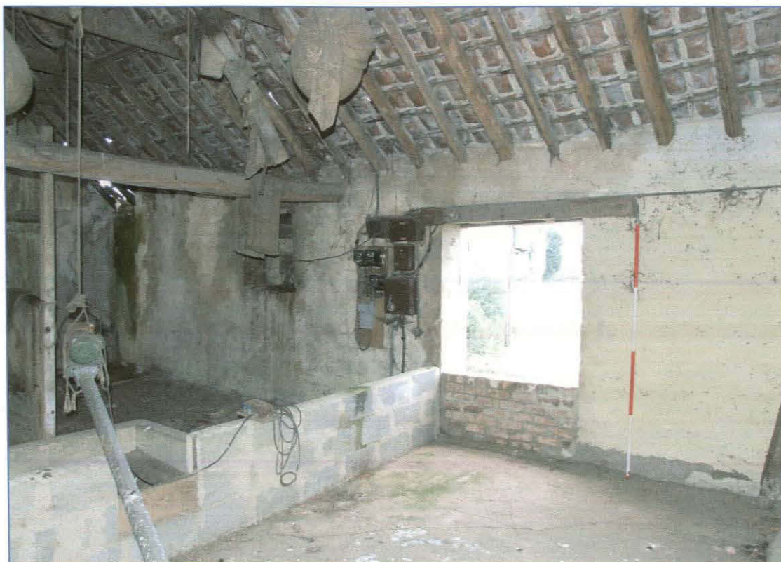
Plate 11: Loading hatch in north wall of Building 3, and breeze block storage bay. The chute in the middle of the breeze block wall allows grain to poured into sacks on the ground floor. Looking north-west.
