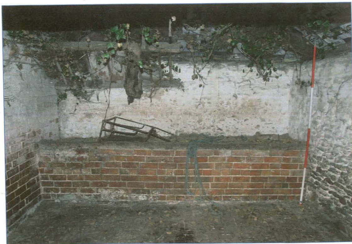
Plate 16: Brick feeding trough in stable block 4b, looking north.
