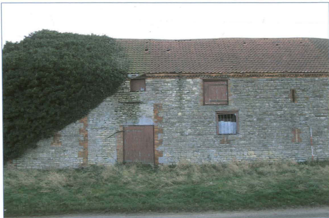
Plate 10: North elevation of Building 3, east end. Note the blocked doorway defined by the saw tooth brickwork with smaller door inserted. The window to the west truncates a ventilation slit. Looking south.
