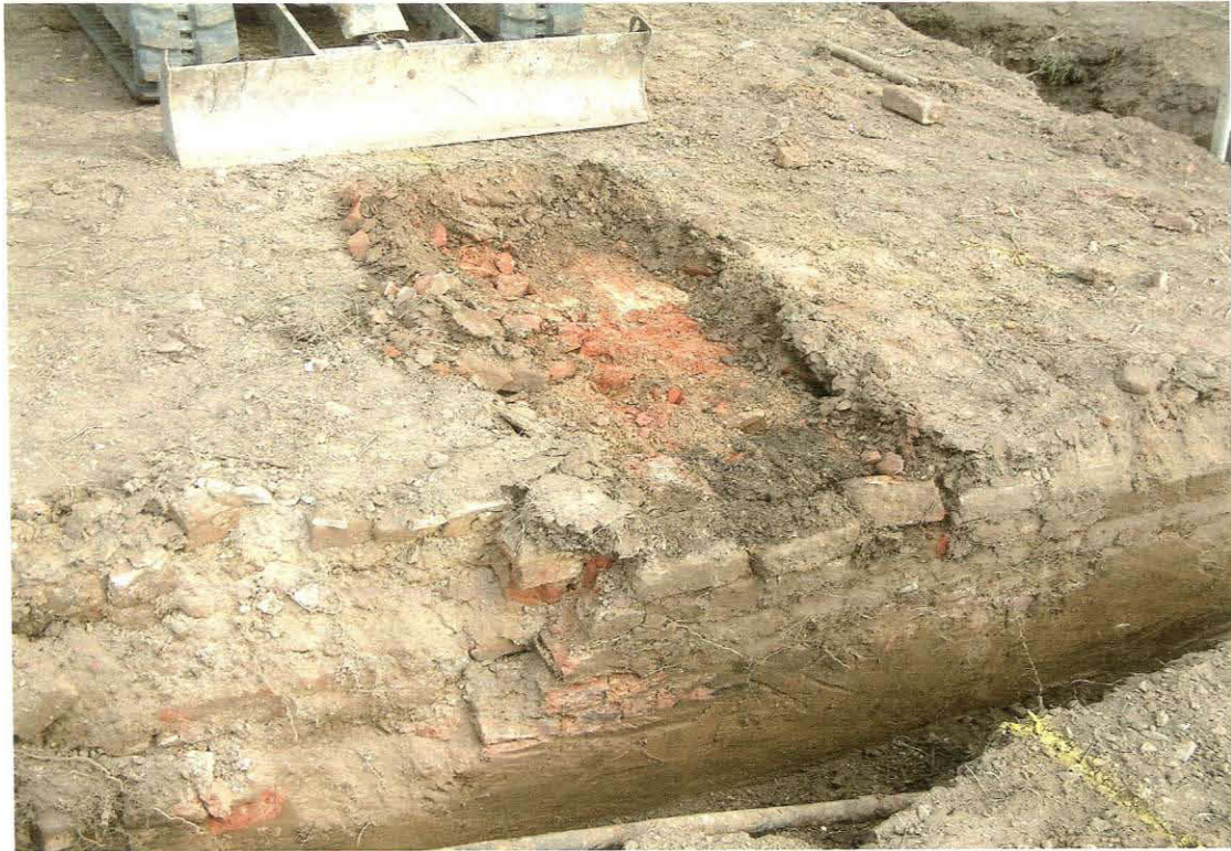
Plate 21. Showing old footings of demolished building left in situ.
