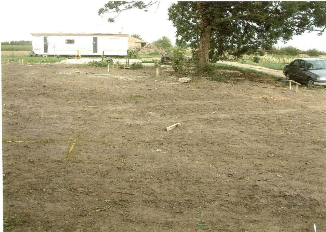
Plate 19. Site after demolition.
