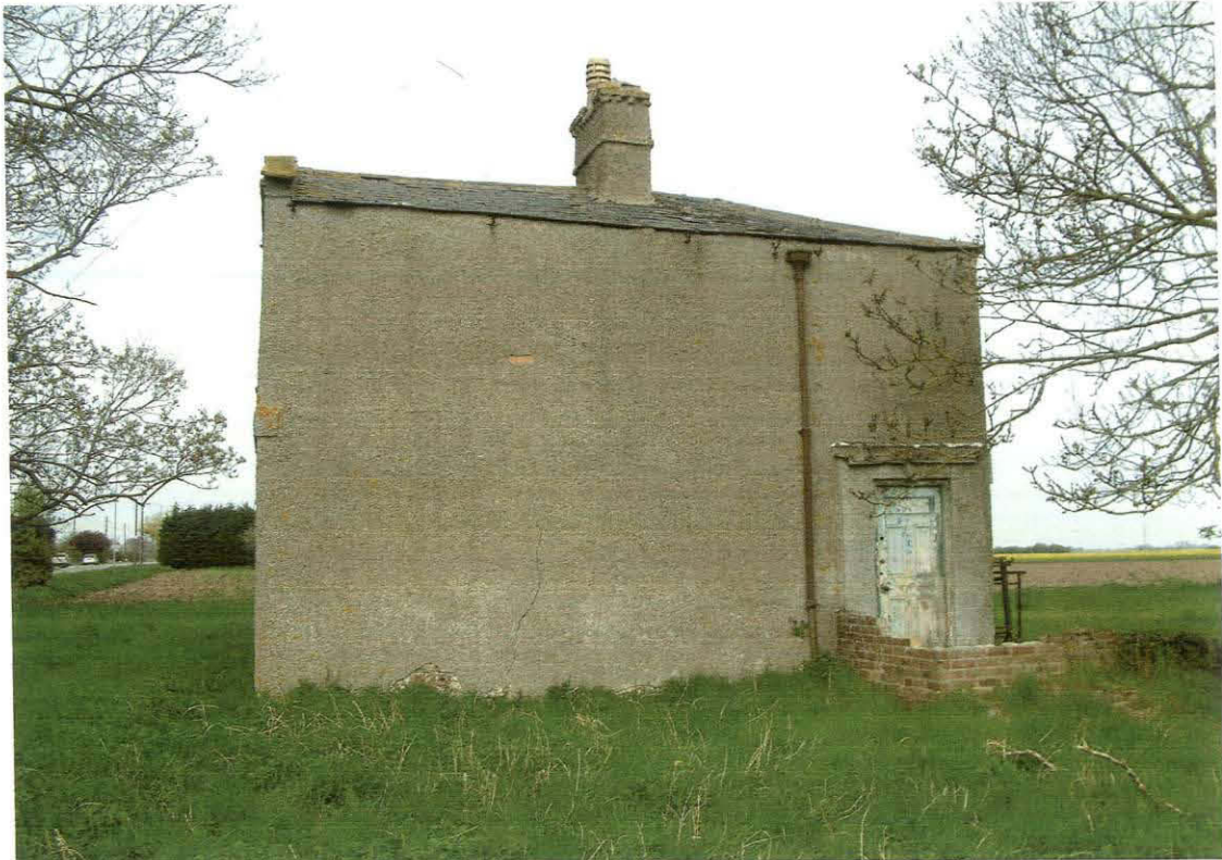
Plate 1. Eastern elevation of Moulton Farm House looking west.
