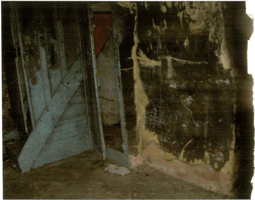
Plate 13. Showing bricked fireplace, staircase and cupboard understairs.
