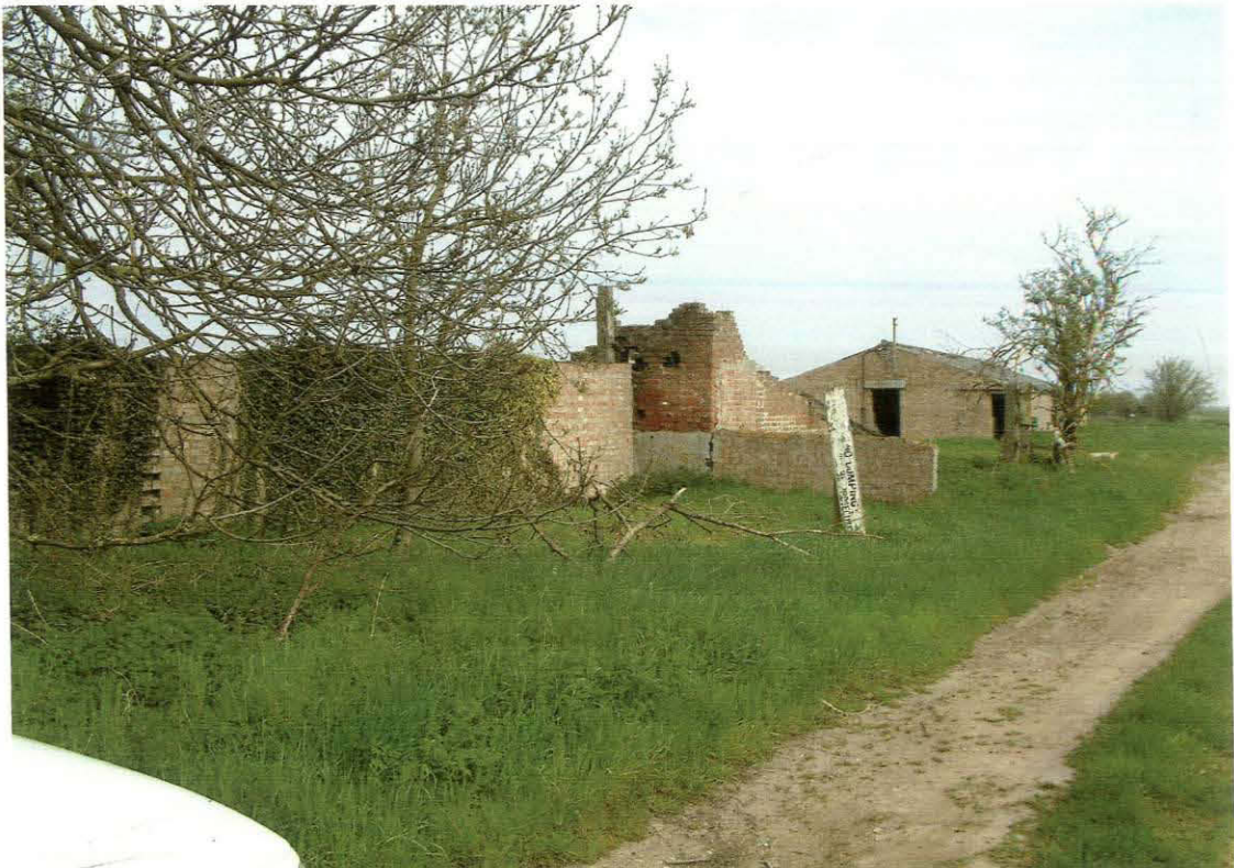
Plate 17. Out buildings to north of property, buildings in foreground to be demolished.
