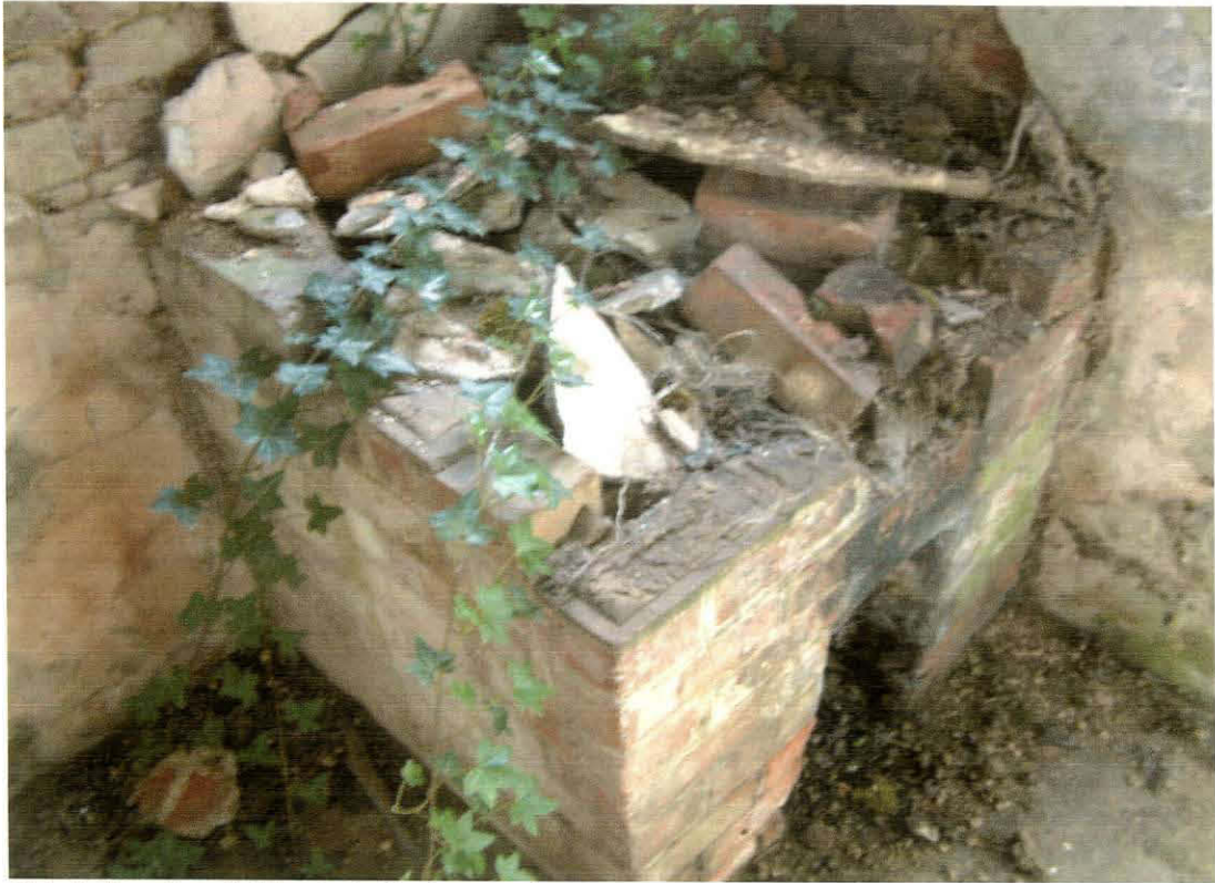
Plate 5. Remains of old water boiler in extension
