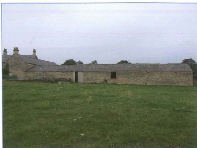
Plate 9: West elevation of Buildings A and B, looking north-east.
