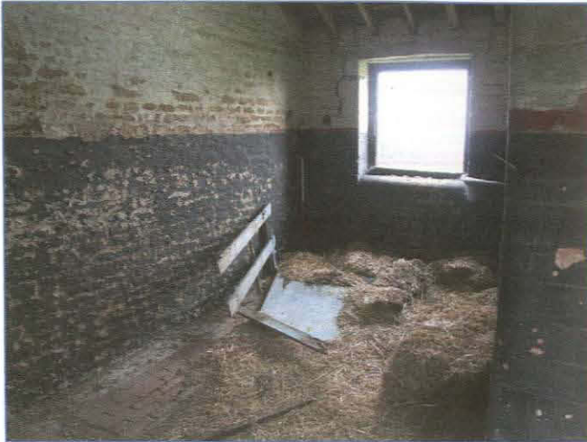
Plate 7: Possible storage room in Building B. Looking south-west.
