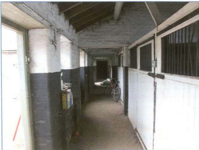
Plate 6: View along the corridor running the length of Building B. Looking south-south-east.
