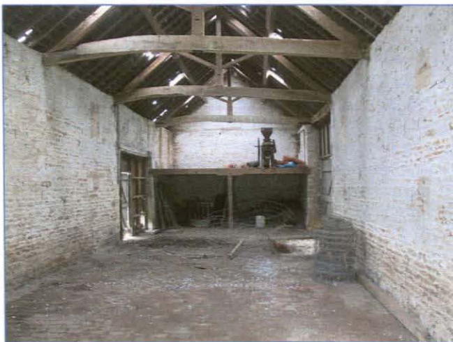
Plate 18: Interior of threshing barn Building E. Looking north-north-west.
