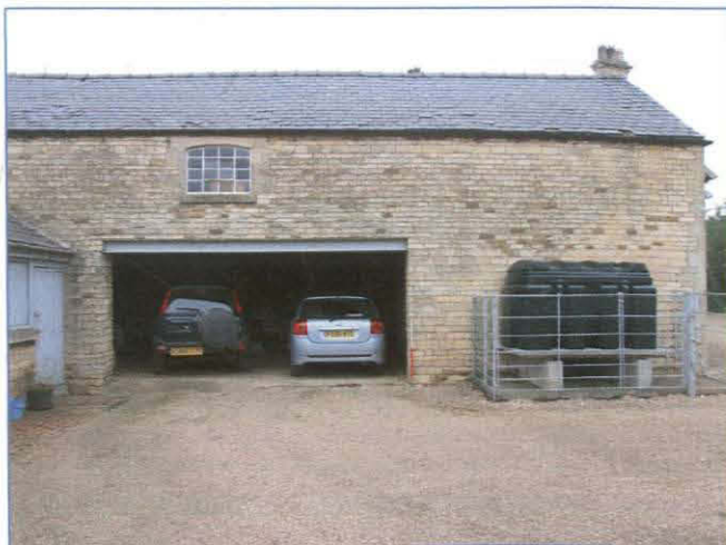
Plate 3: South elevation of the granary/cart shed Building A, looking north-north-west.
