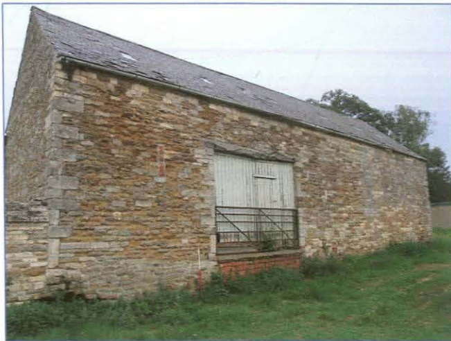
Plate 17: West elevation of threshing barn Building E. Looking east-south-east.
