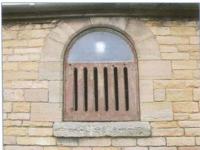
Plate 11: Detail of window in east elevation of Building B. Looking west-south-west.
