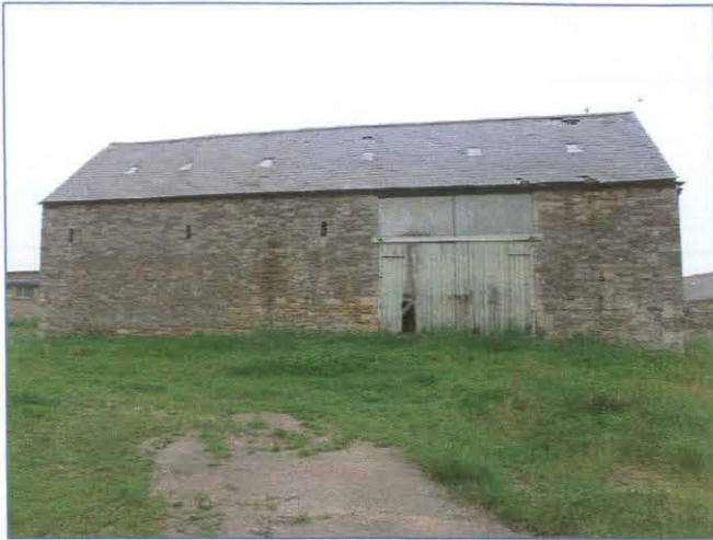
Plate 16: East elevation of threshing barn Building E. Looking west-south-west.
