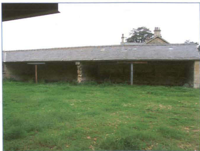
Plate 12: South elevation of cart shed Building C, looking north-north-west.
