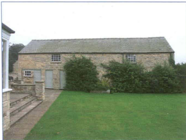
Plate 2: North elevation of granary Building A, looking south-east. The door and window at the east end of the elevation, and possibly the two adjacent doors, have replaced an opening into the cart shed.
