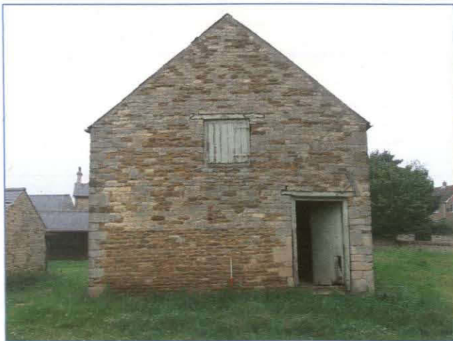
Plate 15: South elevation of threshing barn Building E. Looking north-north-west.
