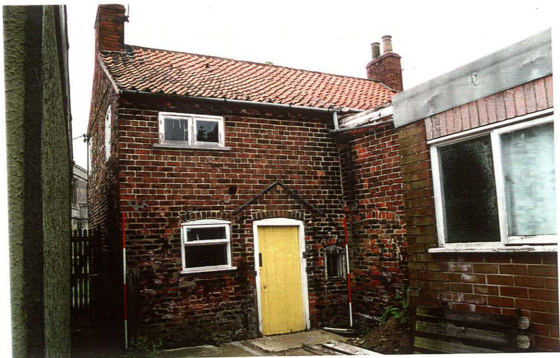
Pl. 2 Rear entrance to School House, prior to demolition of reading room. Looking E.
