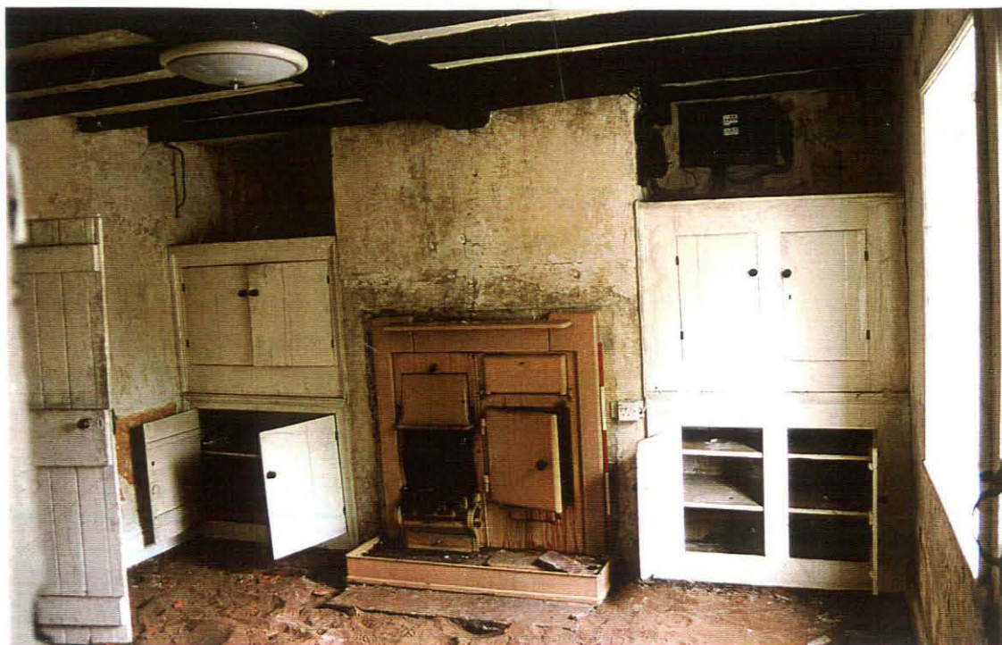
Pl. 5 School House kitchen with 1937 solid-fuel aga, looking NW. Tile floor has been removed, leaving sand levelling visible.
