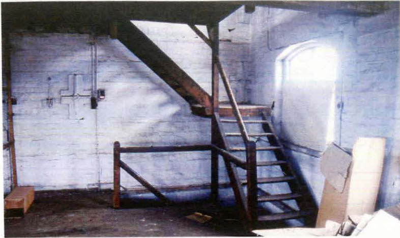
Plate 14 Detail of stairway, northern part of mill
