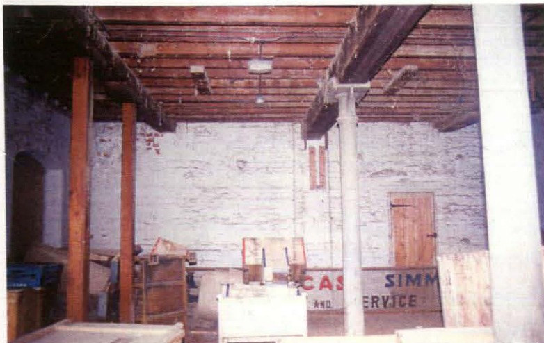
Plate 17 Mill southern part, showing timber and cast iron supports
