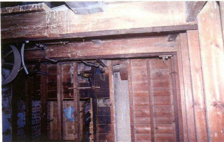
Plate 19 Panelling, 5 th storey. Note pulley wheel and shaft behind panelling, centre
