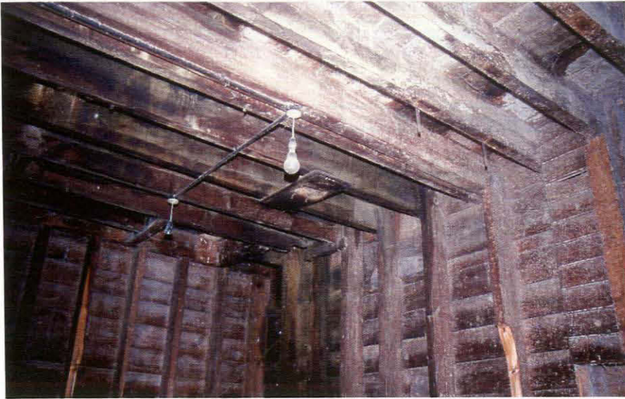
Plate 18 Timber panelling, 3 rd storey. Note elevator duct in ceiling
