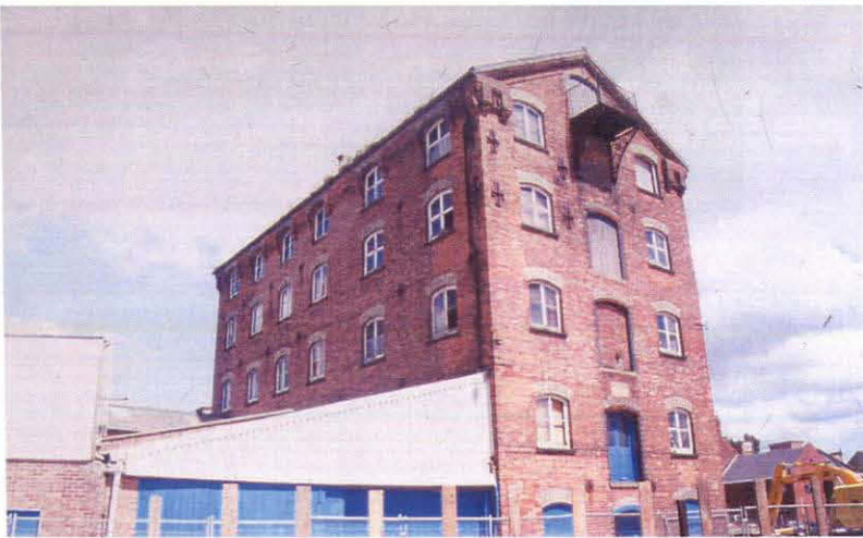
Plate 2 Mill building, south and west elevations
