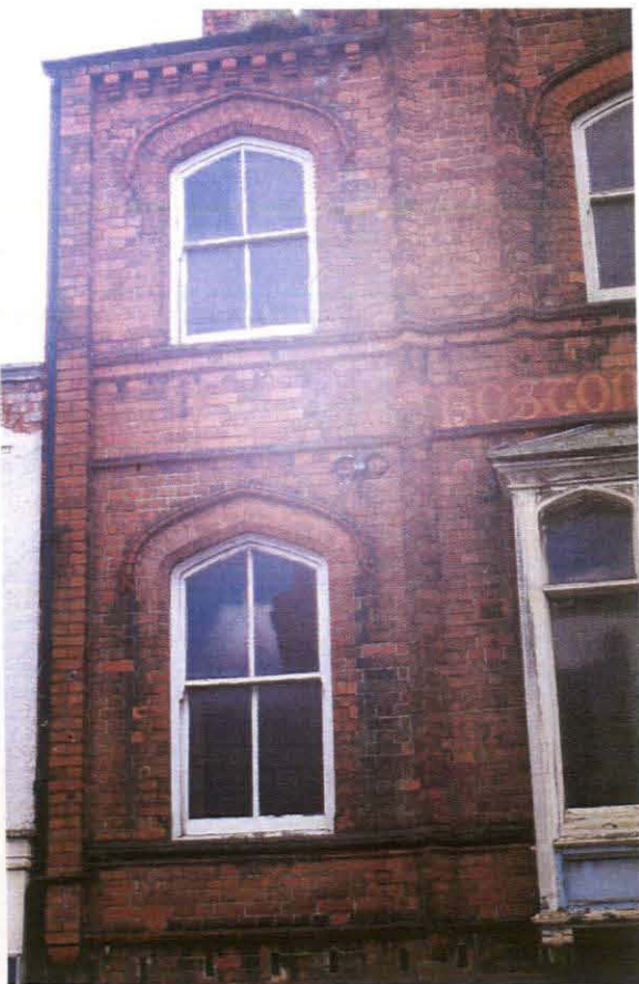
Plate 26 Boston Guardian building, windows with brick hood moulds
