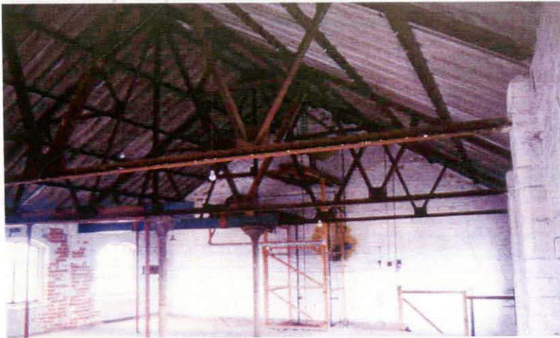
Plate 15 Cast iron roof trusses in northern part of mill
