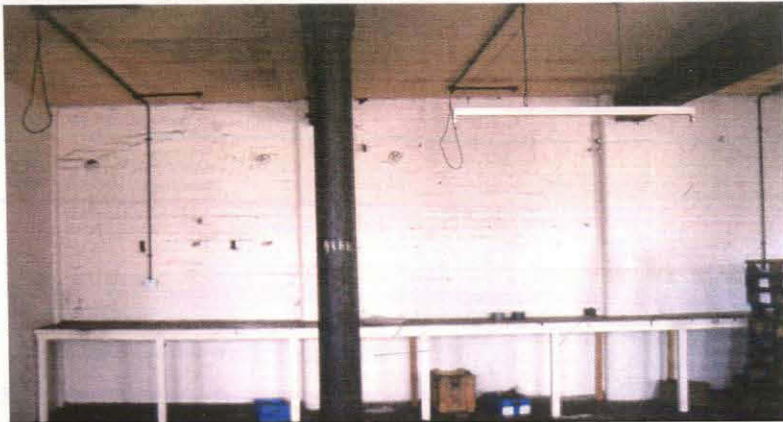
Plate 16 Mill west wall, showing blocked windows
