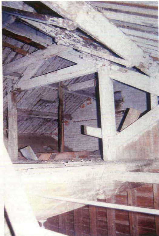
Plate 22 Queen post roof truss, mill southern part
