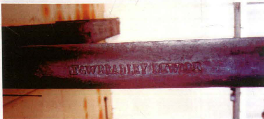
Plate 13 Detail of maker's name on cast iron column
