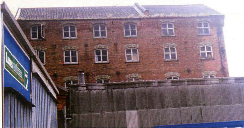
Plate 7 Mill, western elevation, showing dividing wall extending above roof line
