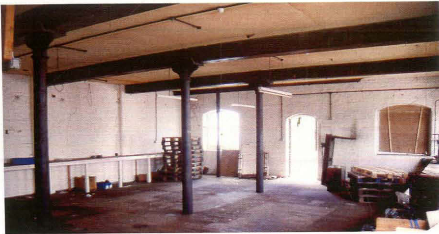
Plate 11 Mill second storey, northern part, showing cast iron columns
