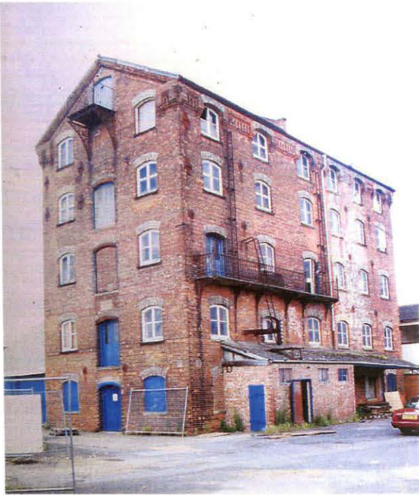
Plate 1 Mill building, south and east elevations
