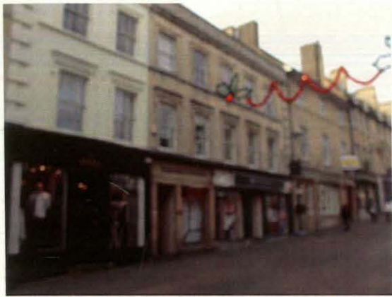
Plate 1 General View showing 10 Ironmonger Street frontage, looking northwest
