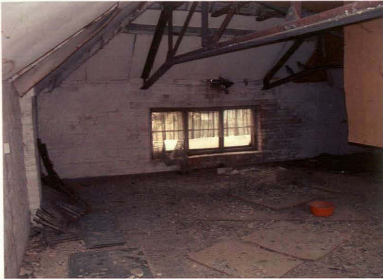
Plate 12 Assessed Building, 2 nd floor, general view, looking east
