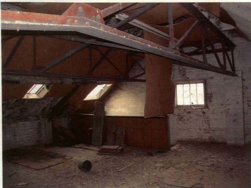
Plate 11 Assessed Building, 2 nd floor, view toward stairwell, looking southwest
