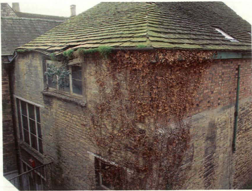
Plate 5 Assessed Building, eastern and northern elevations, looking south
