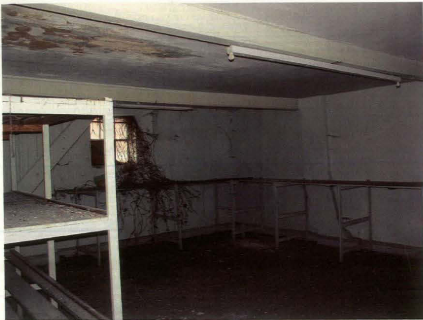
Plate 9 Assessed Building, 1 st floor, general view, looking west
