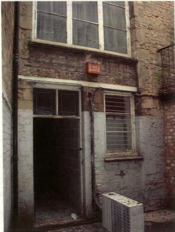
Plate 2 Assessed Building, eastern elevation (southern part), looking west
