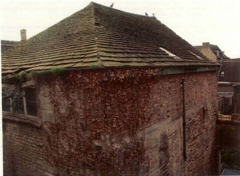
Plate 6 Assessed Building, northern elevation, showing offset, looking southwest
