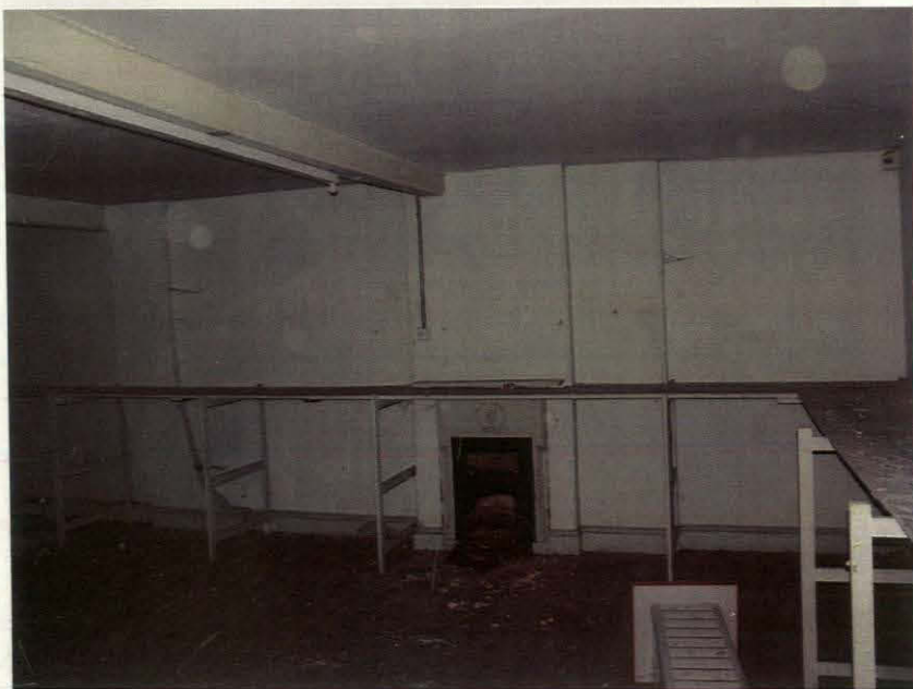
Plate 10 Assessed Building, 1 st floor north side, showing fireplace, looking northwest
