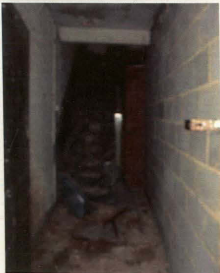
Plate 7 Assessed Building, ground floor passage and stairwell, looking southwest
