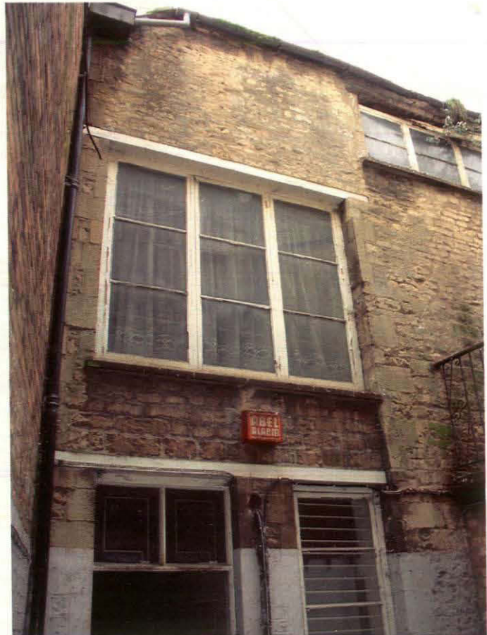
Plate 3 Assessed Building, eastern elevation, upper levels, looking west
