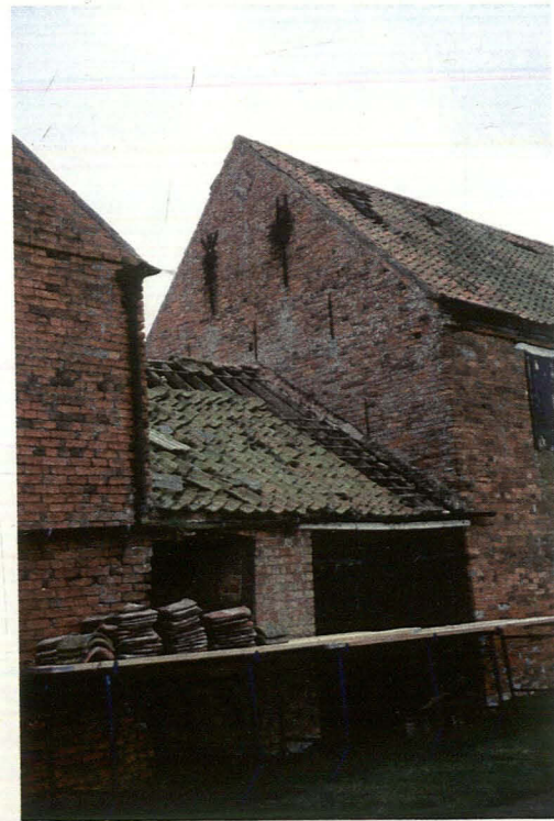
Plate 6 single storey covered passageway and garage, north elevation, and east elevation of main barn with initials 'W H' formed by stay plates, looking southwest
