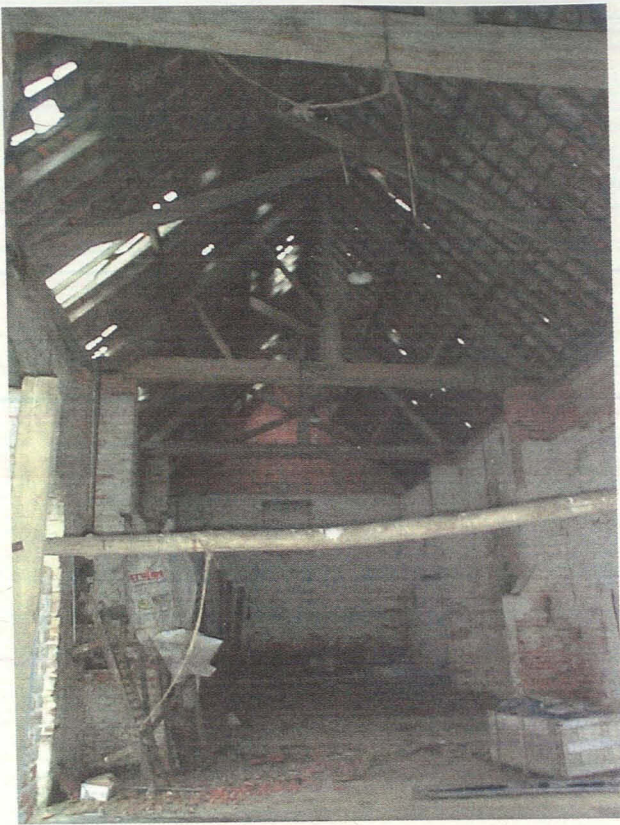
Plate 12 Interior of main barn, looking east
