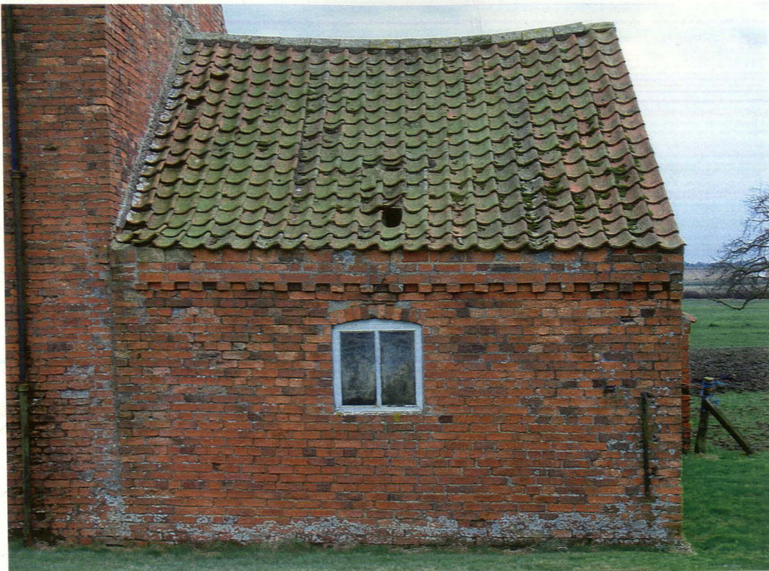
Plate 29 North elevation of probable shed addition to main barn, looking south
