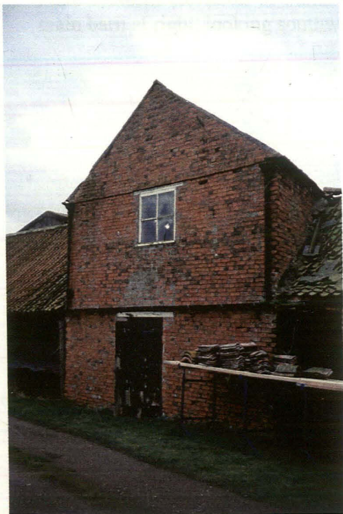
Plate 5 Two-storey northwest-southeast angled range, north elevation, looking southeast
