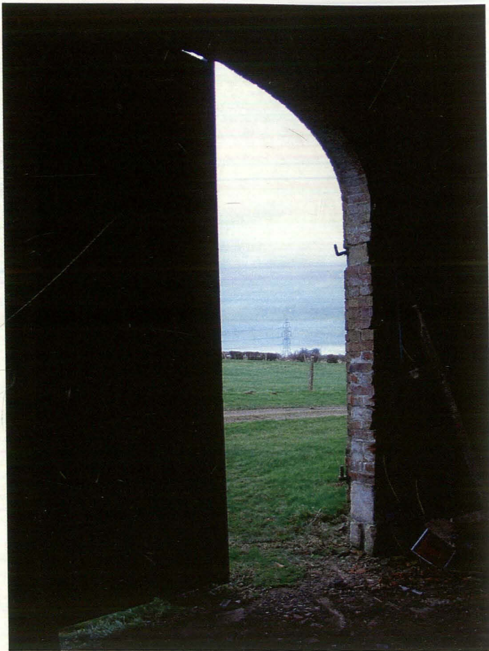
Plate 18 Interior of main barn, view of northern doorway including groove at base of door jamb, looking northeast
