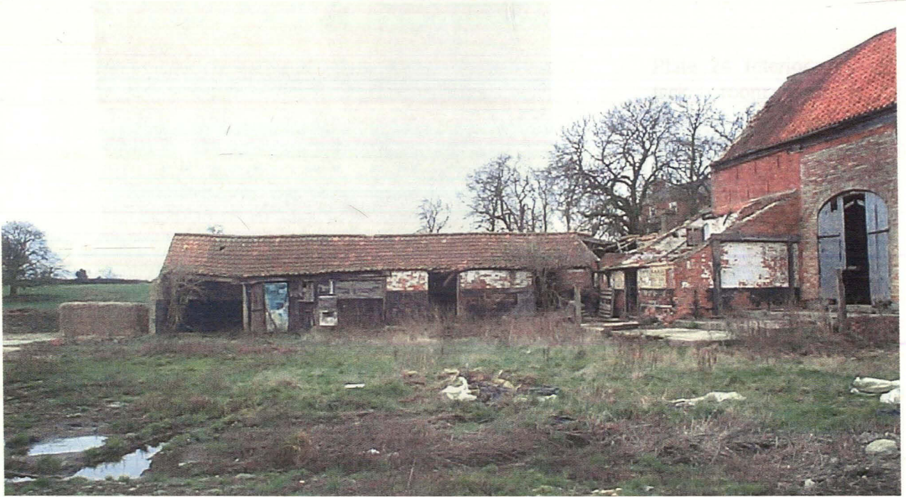
Plate 22 East elevation of north-south range of loose boxes and shelter shed, including lean-to stable and main barn at right. Rectangular arrangement of timbers of east elevation of lean-to stable is probably part of former yard covering, looking west
