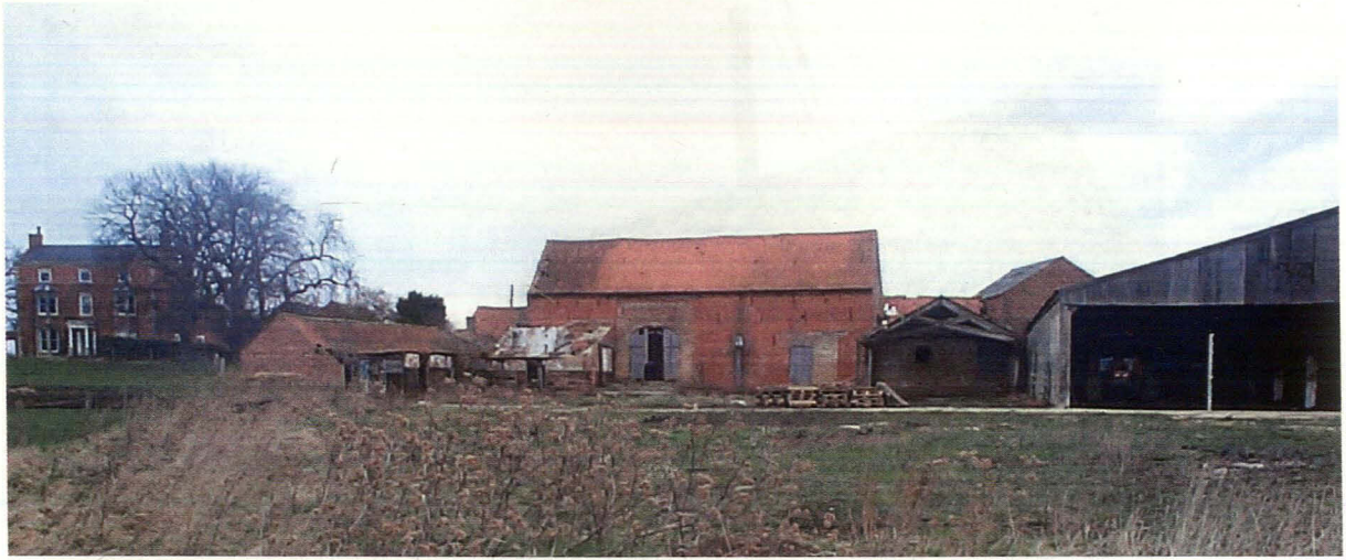
Plate 1 General view of barns, including Boughton House at left, looking north
