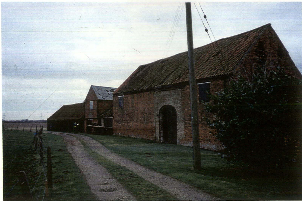
Plate 4 North elevation of barns with main barn in foreground, looking southeast
