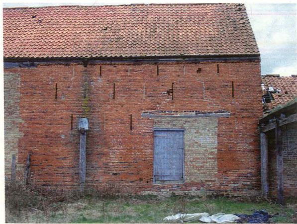
Plate 10 South elevation of main barn, east end, showing partially blocked doorway and breather slits (some blocked). Wood at left is probably part of former yard covering, looking north
