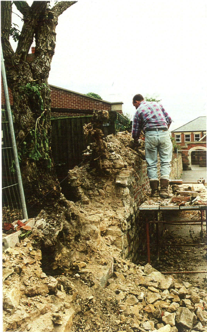
P.7 Working shot, showing dismantling of wall, looking east.
