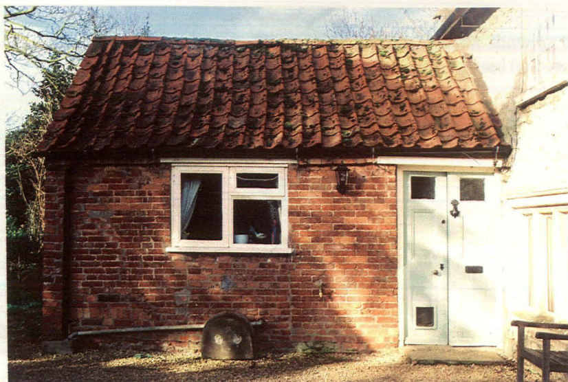
Plate 4 - The east facing elevation showing modern patching to left of picture and ragged joins below the window, looking west
