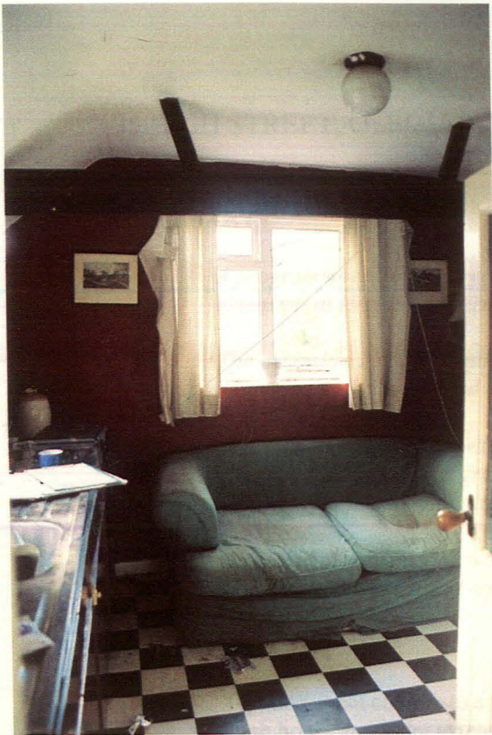
Plate 7 - View showing the larger room within the extension with exposed tie-beams and raking struts, looking south
