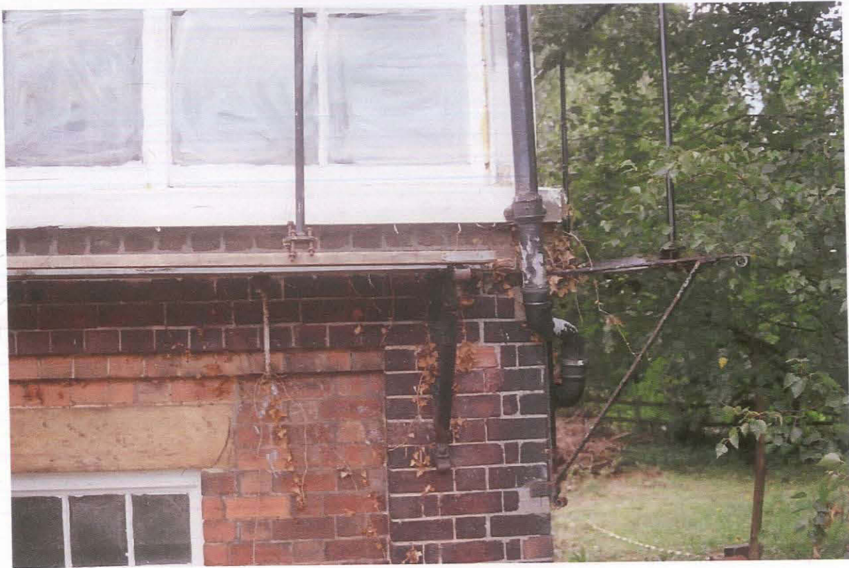
Pl. 13 A view showing the cast iron down pipes, recessed window, glazing and balcony on the south-western corner of the building.
