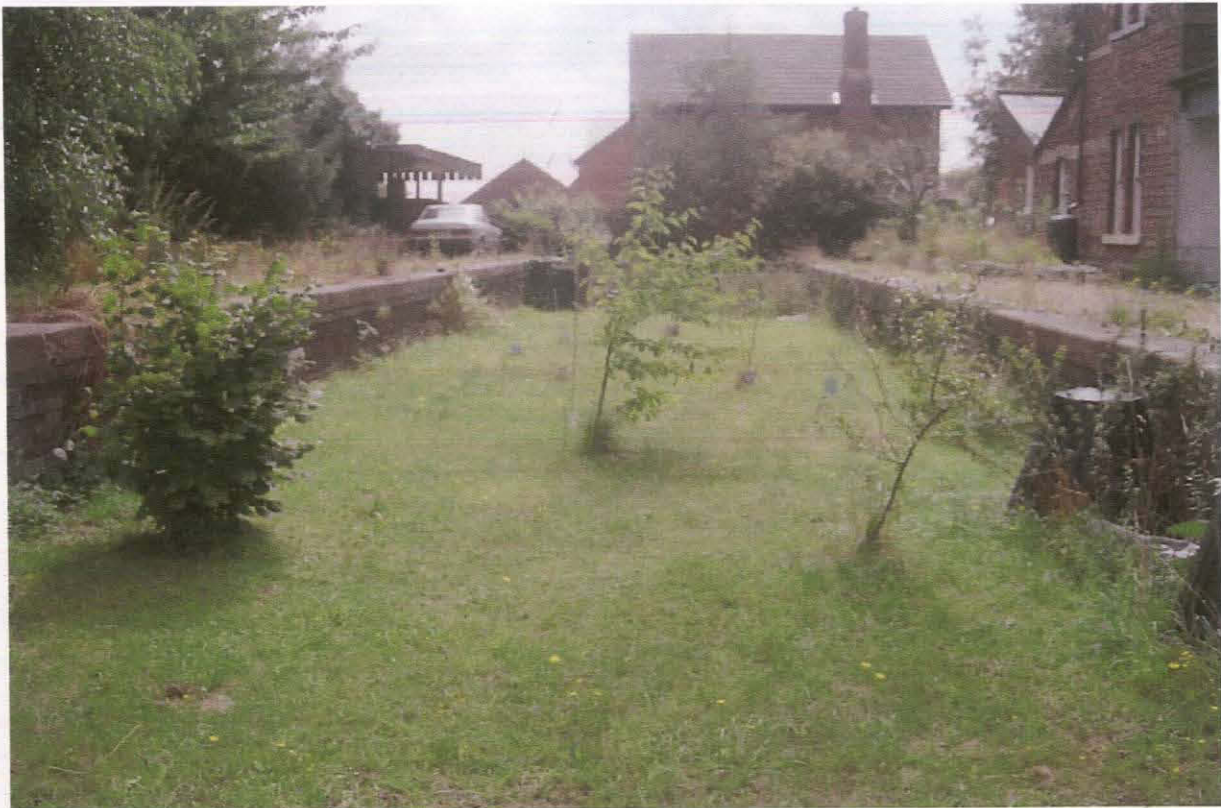
Pl. 16 The line of the former railway and station platforms to the immediate west of the signal box ✓
