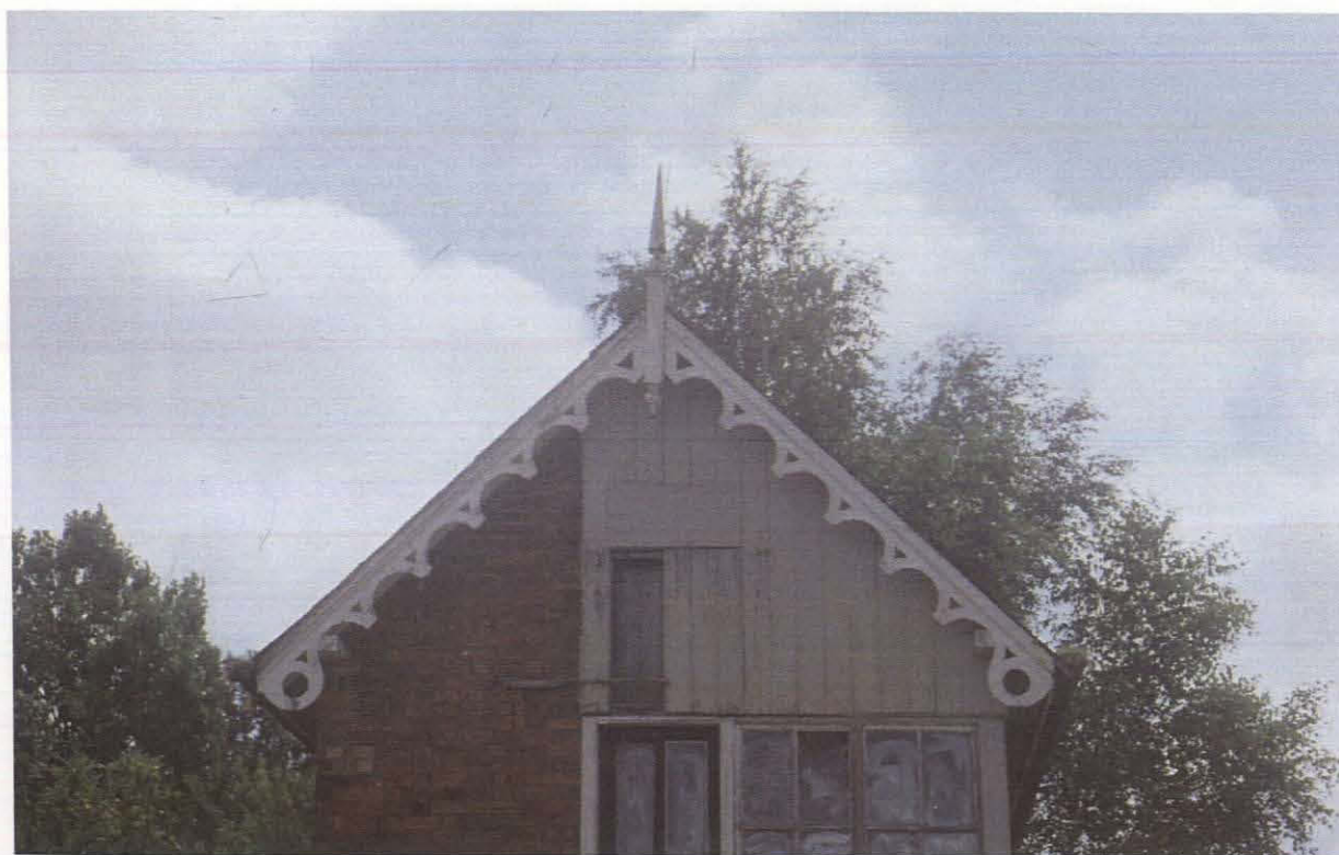
Pl. 8 The north elevation, detail of the bargeboards and finial
