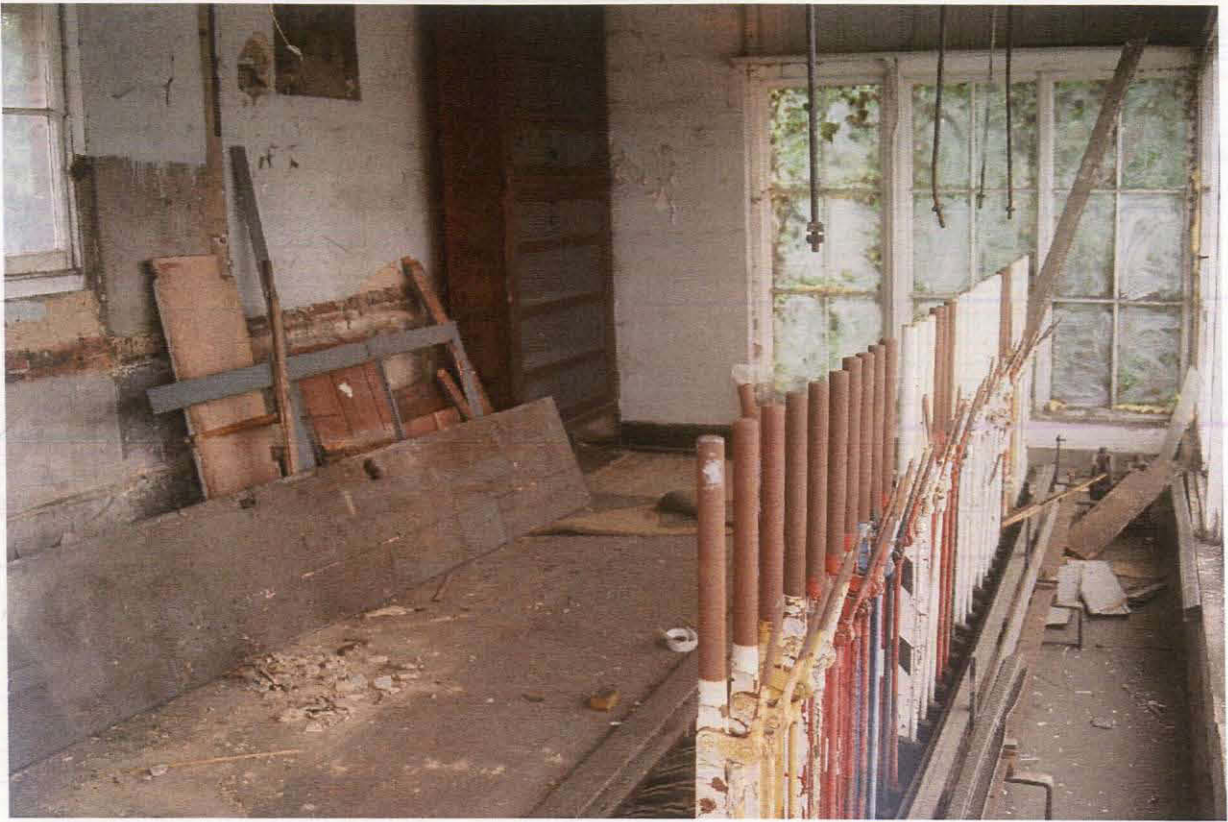
Pl. 13 General view Looking south-east across the first floor
