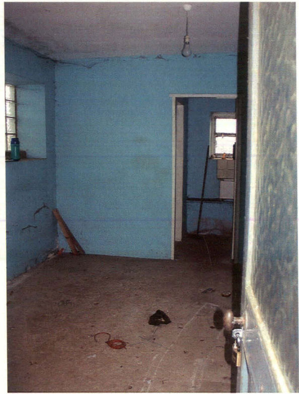
Plate 18 Wash rooms-southern central barn, looking southwest
