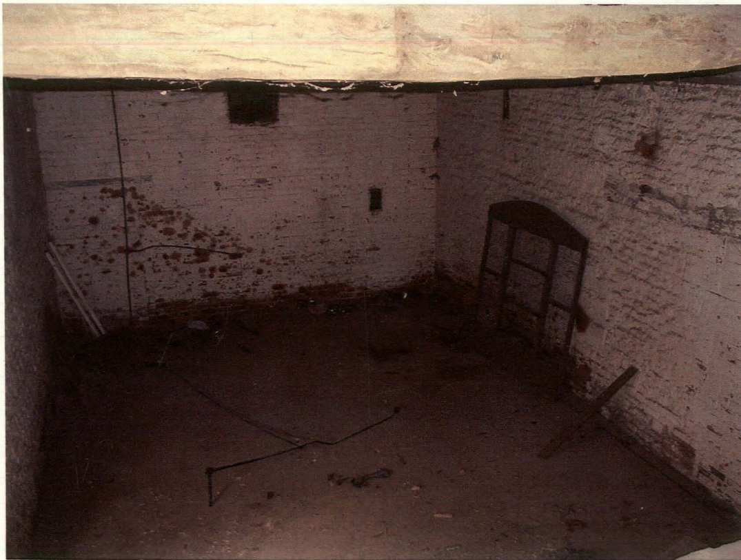
Plate 19 Blocked internal doorway, in southern central barn, looking southeast
