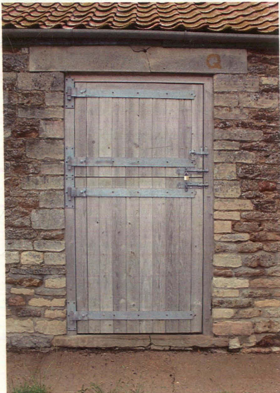
Plate 11 Barn door, in southeastern elevation of northern barn, looking northwest
