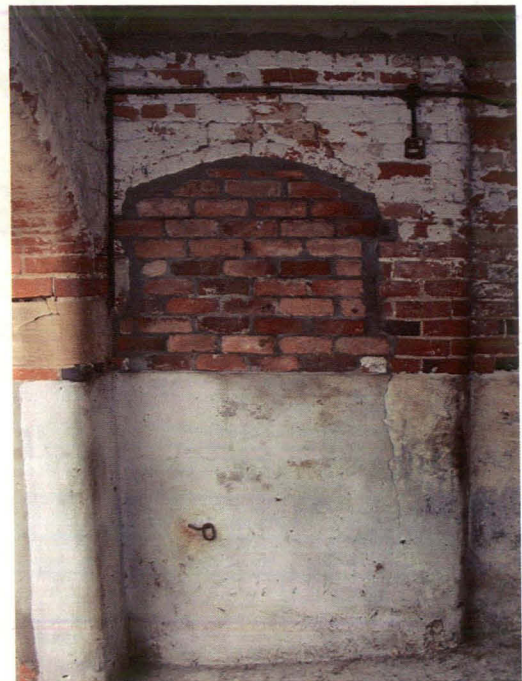
Plate 26 Blocked internal doorway, north central barn, looking northwest
