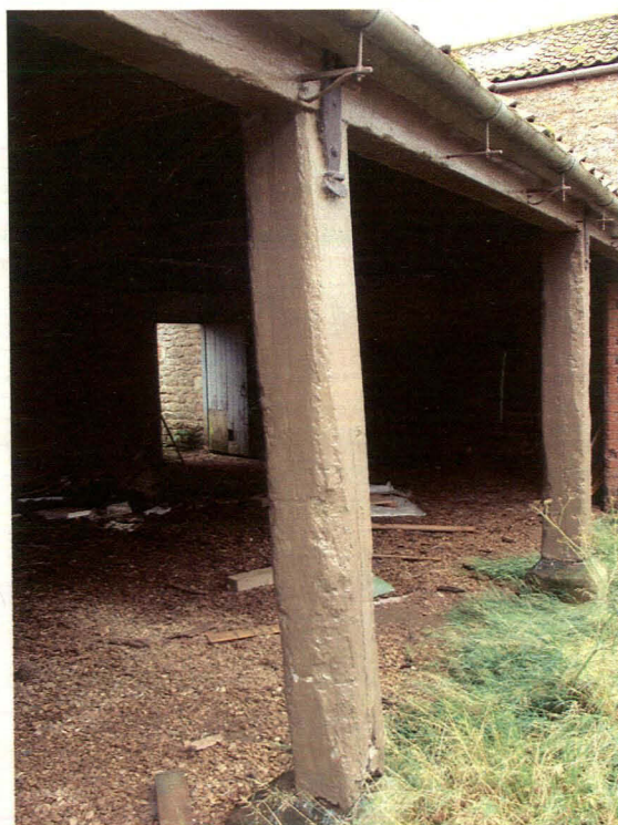
Plate 31 Wooden stanchions with iron tie bar, looking SSW
