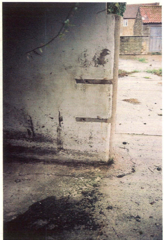
Plate 8 Southeastern cell of northern barn, removed gate latches, looking northwest
