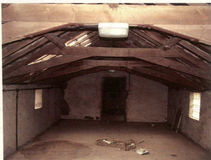
Plate 29 First floor of northern central barn, looking southeast
