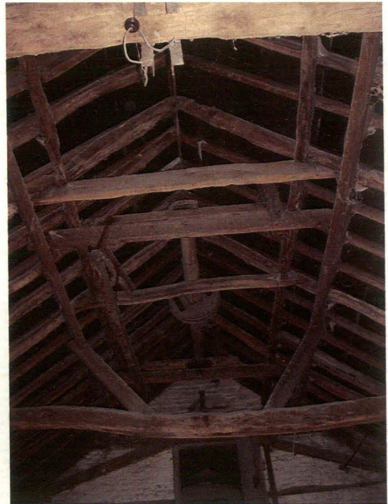
Plate 22 Timber roof in the southern central barn, looking northwest
