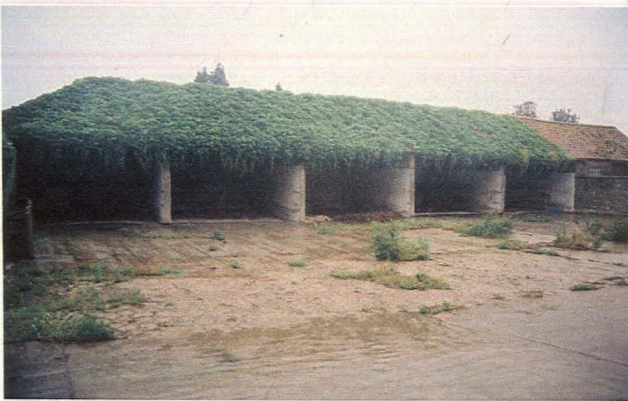
Plate 3 Western Barn, looking west
