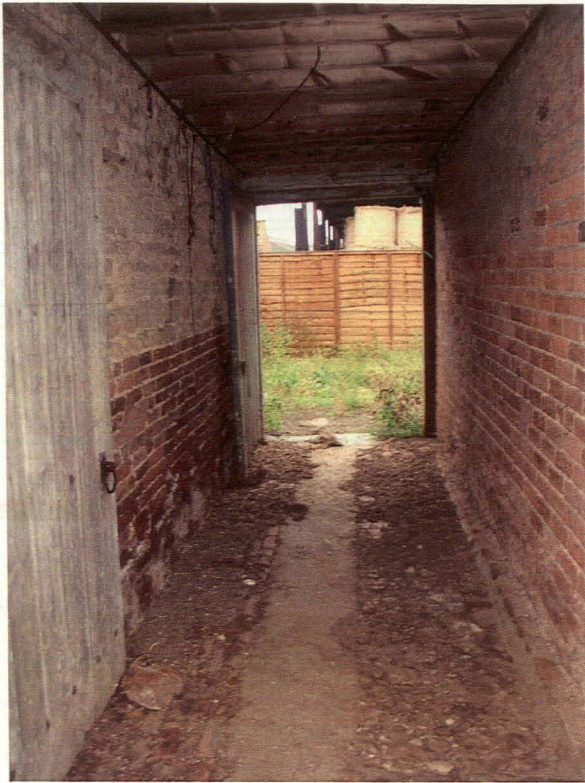
Plate 17 Brick flooring in passageway-southern central barn, looking northeast
