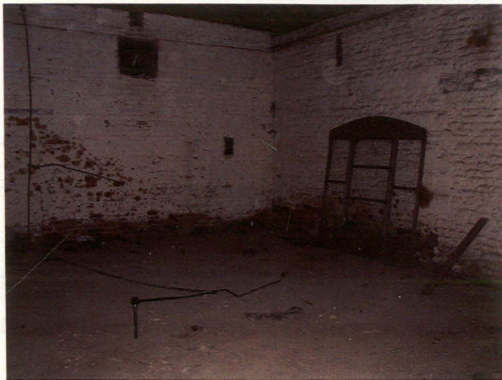
Plate 24 Blocking of recess and faint trace of removed machine, looking south
