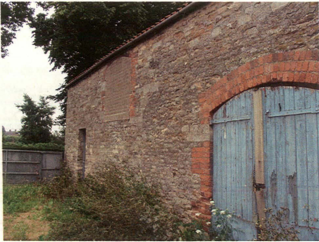
Plate 21 Northeastern elevation of southern central barn, showing large blocked window and segmental arched doorway, looking south
