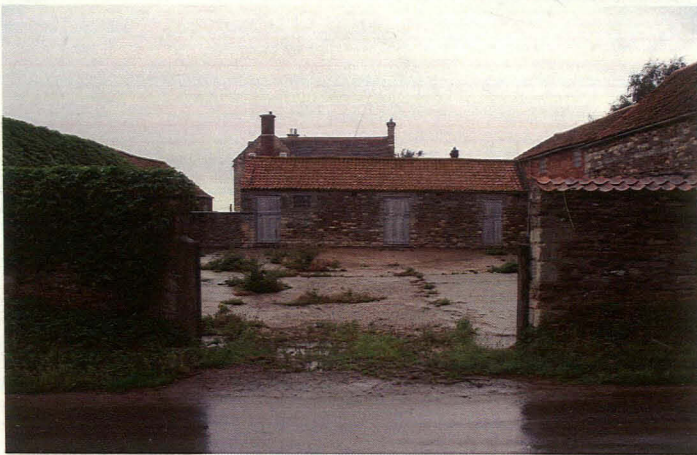
Plate 2 Eastfield Barns, looking northwest
