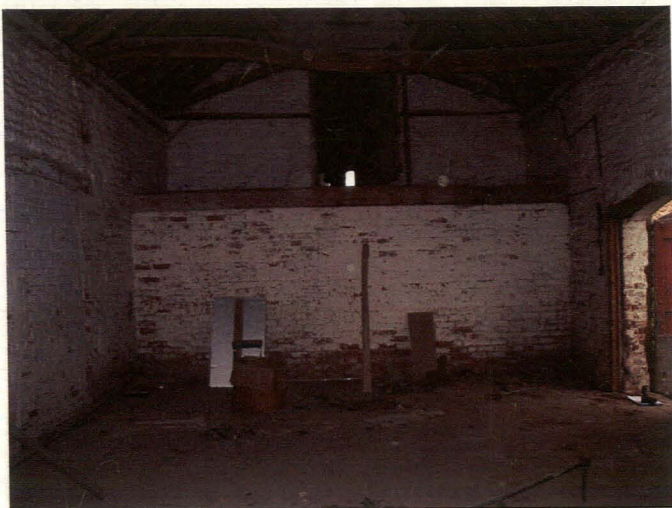
Plate 15 Mezzanine in central southern barn, looking northwest
