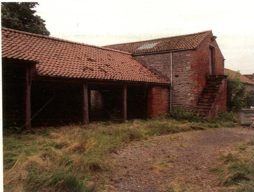
Plate 28 External staircase to first floor of northern central barn, looking south
