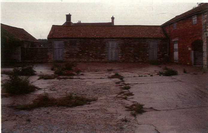
Plate 4 Northern Barn, looking northwest
