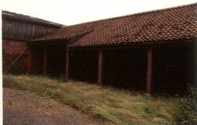
Plate 30 Northwestern stanchioned elevation of eastern barn, looking ENE
