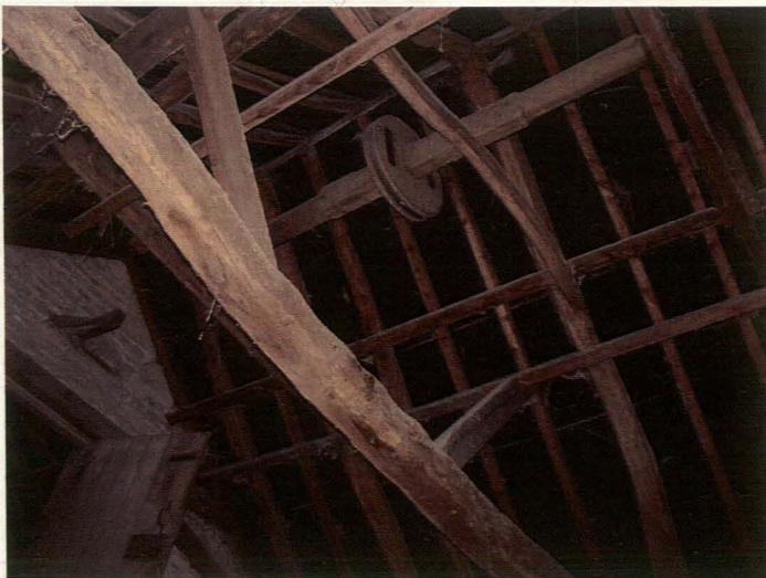
Plate 23 Hoist cog in southern central barn, looking north
