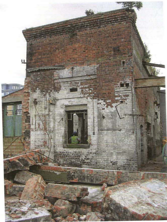
Pl. 17 Water tower after demolition of the north extension, looking south
