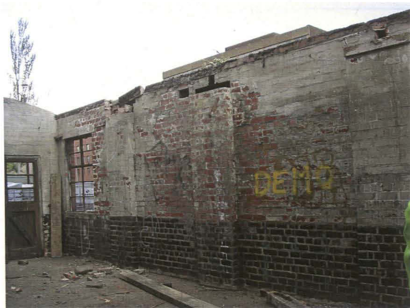
Pl. 22 East extension, interior looking NE
