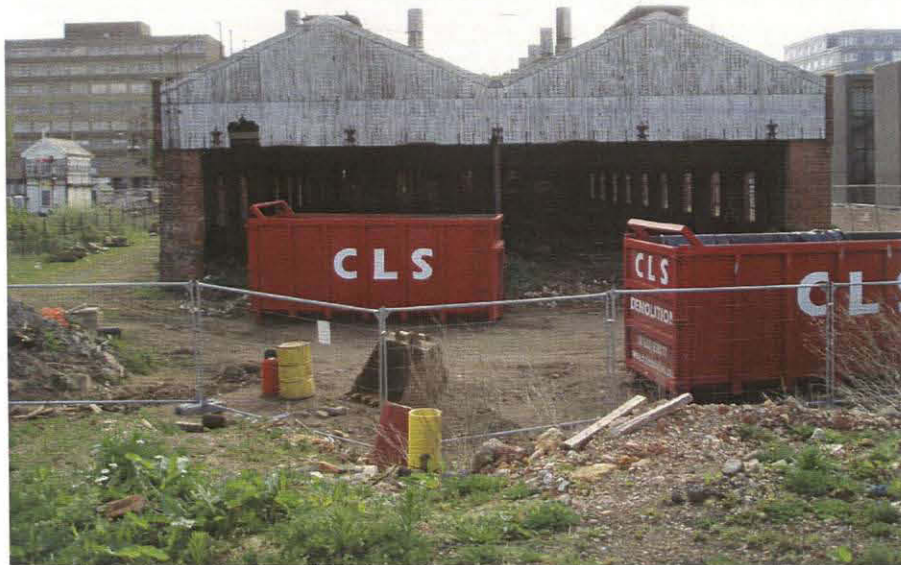
Pl. 7 Engine shed W elevation
