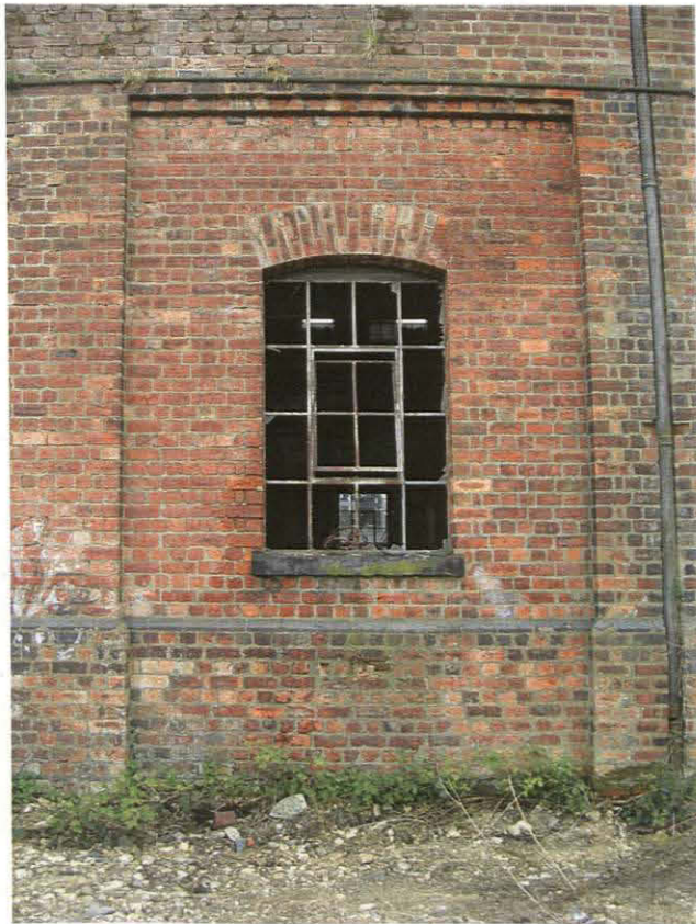
Pl. 14 Engine shed N elevation, window
