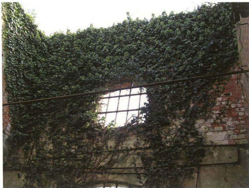
Pl. 26 Water tower interior, upper window in south elevation
