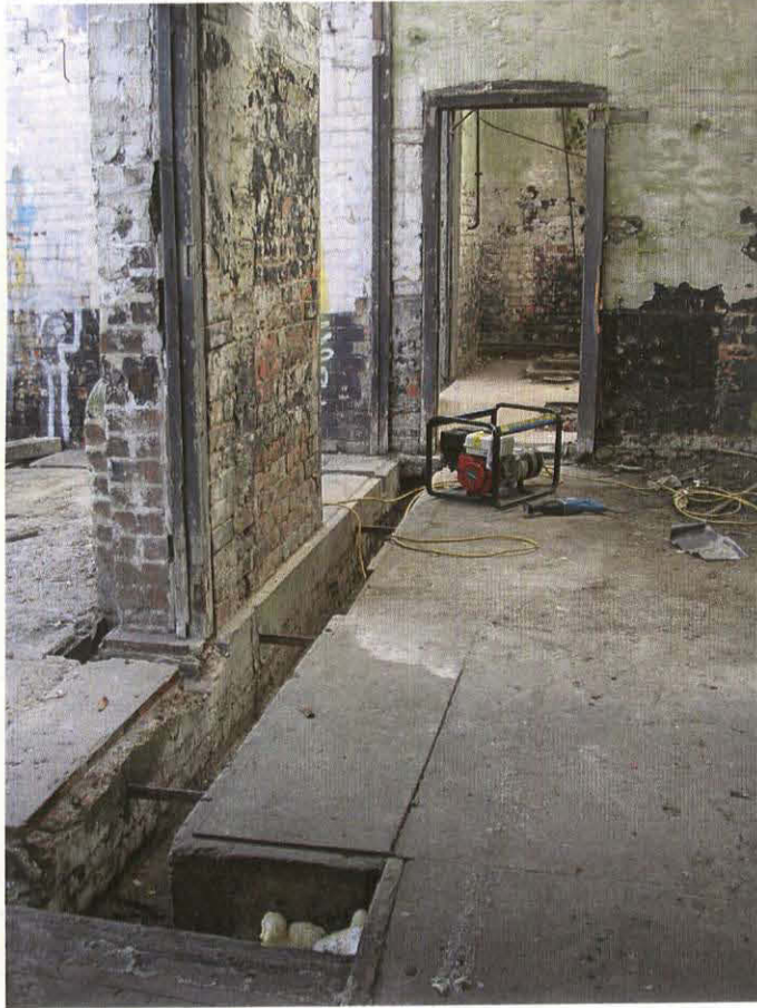
Pl. 29 Water tower interior, boiler room, looking N.
