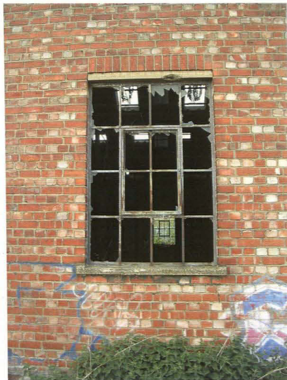
Pl. 12 Engine shed S elevation, window
