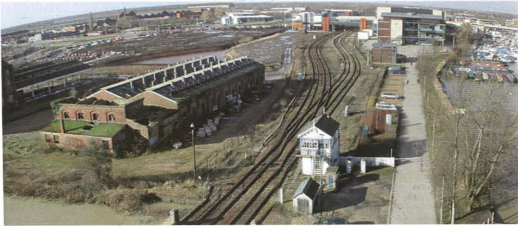
Pl. 1 General overhead view of the engine shed , water tower and associated outbuildings, taken in 2002. Photo courtesy University of Lincoln .
