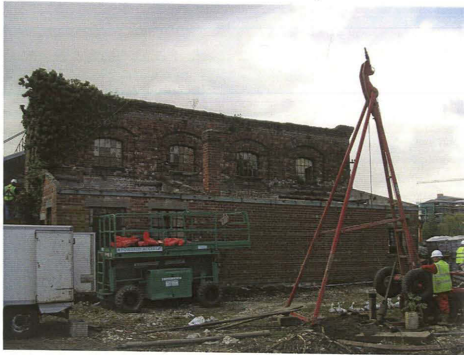
Pl. 33 Piling in progress to east of the water tower, looking NW.
