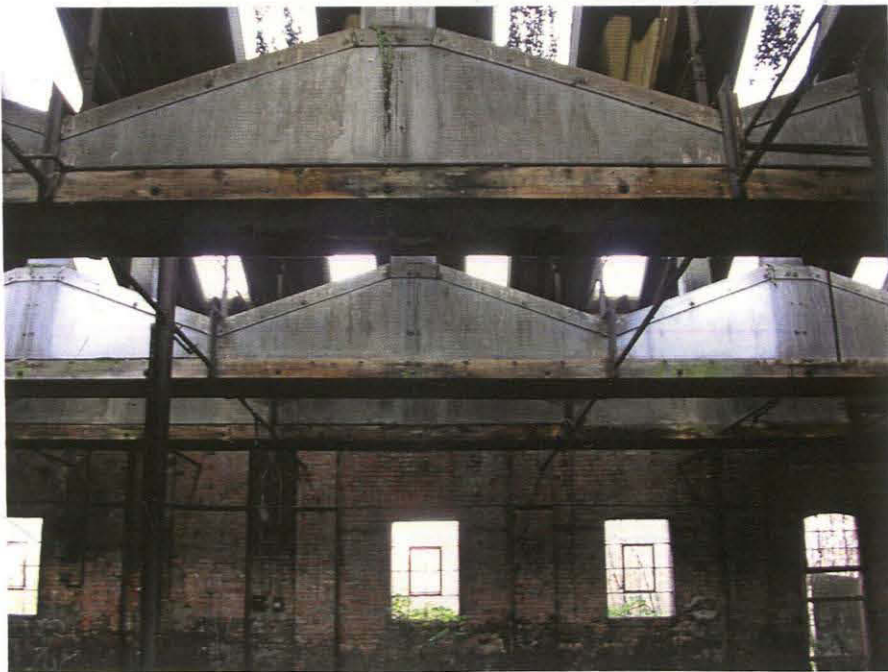
Pl. 10 Engine shed interior, detail of ventilation hoods
