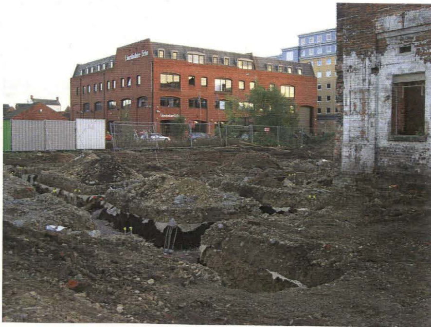
Pl. 34 Groundworks north and east of the water tower (looking south-east)
