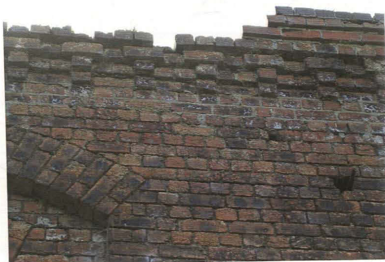
Pl. 18 Water tower , detail of decorative brickwork
