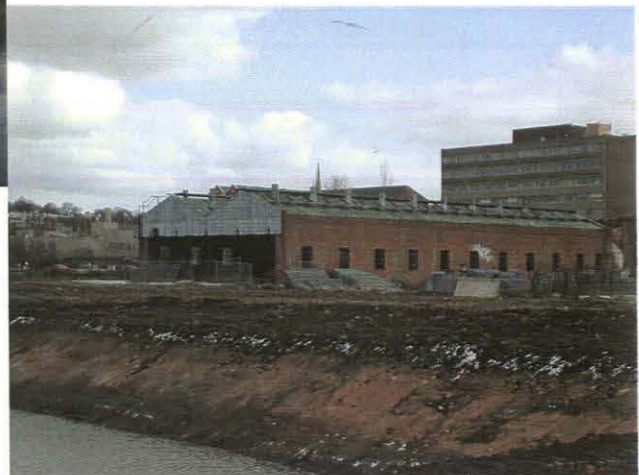
Pl. 6 General view of the engine shed S and W elevations (looking NE)
