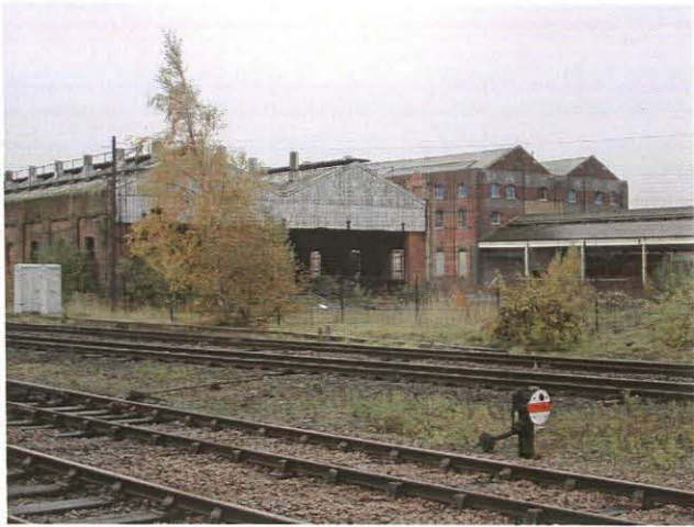
Pl. 3 General view of the engine shed W and N elevations (looking SW)
