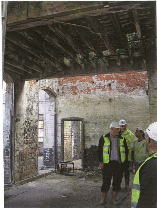
Pl. 31 Water tower interior, boiler room looking N
