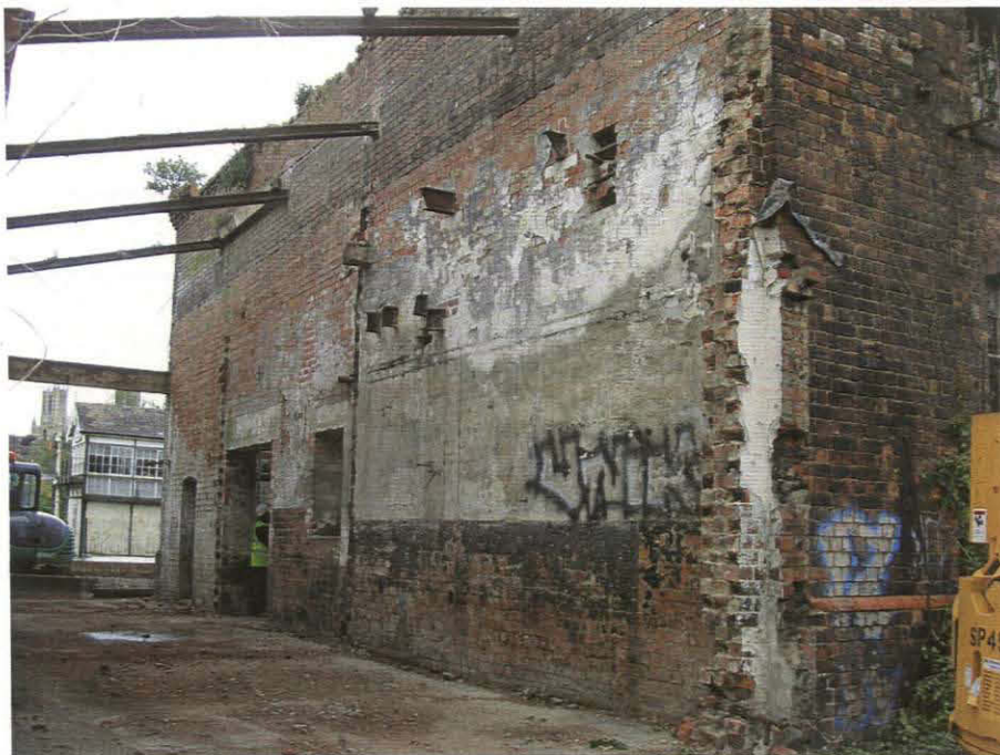
Pl. 20 Area to the west of the water tower after demolition
