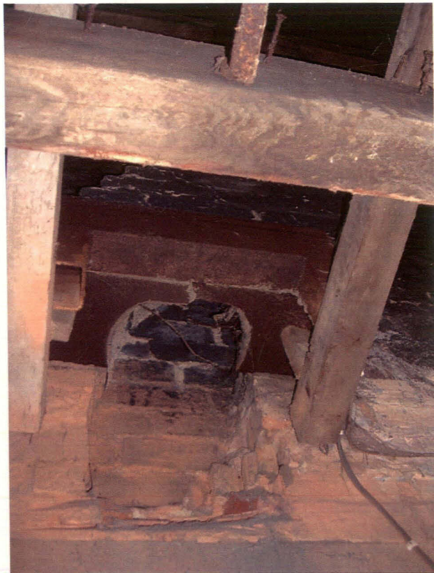
Plate 10 - Detail showing the chimney hood or collar within the larger room
