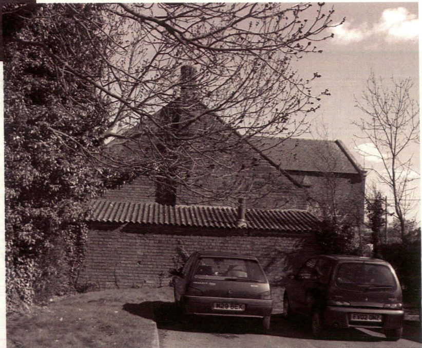
Plate 18 School western elevation and lean-to, looking east
