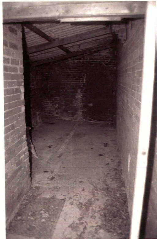
Plate 29 Lean-to, main room, showing wall scar on floor, looking north
