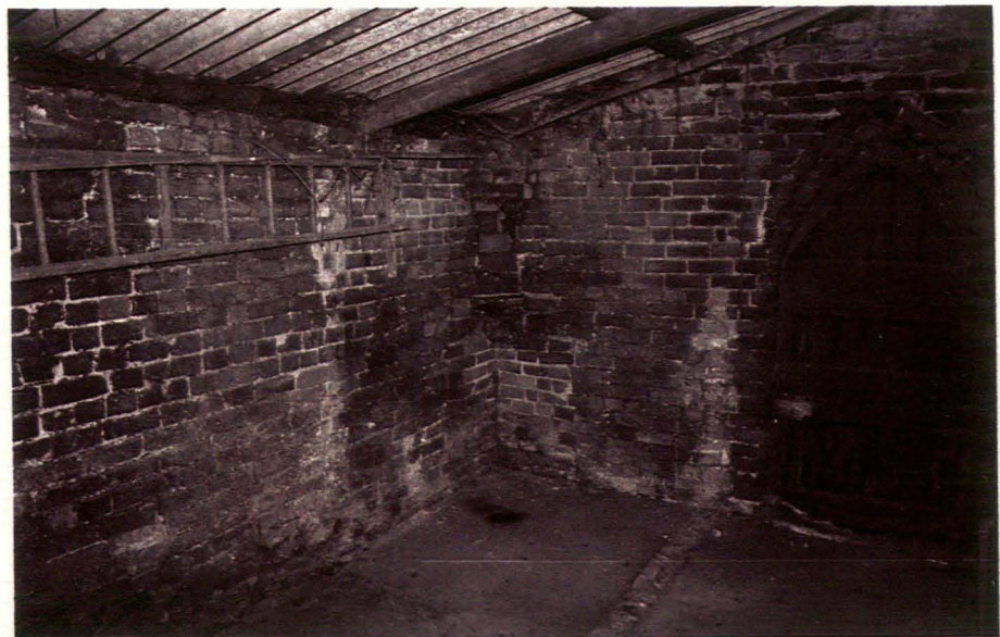
Plate 30 Lean-to interior, northwest corner, showing straight joins and possible chimney remnants, looking northwest
