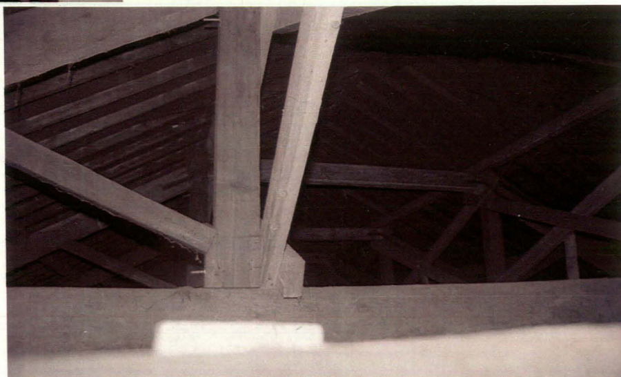
Plate 15 Timbering in roof space above church, looking south
