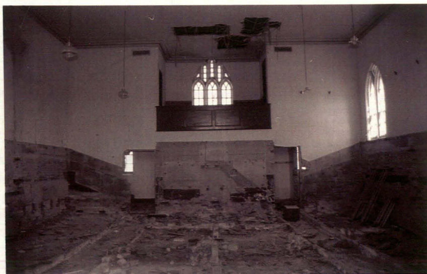
Plate 9 Church interior, showing scars of removed pulpit and first floor gallery, looking north
