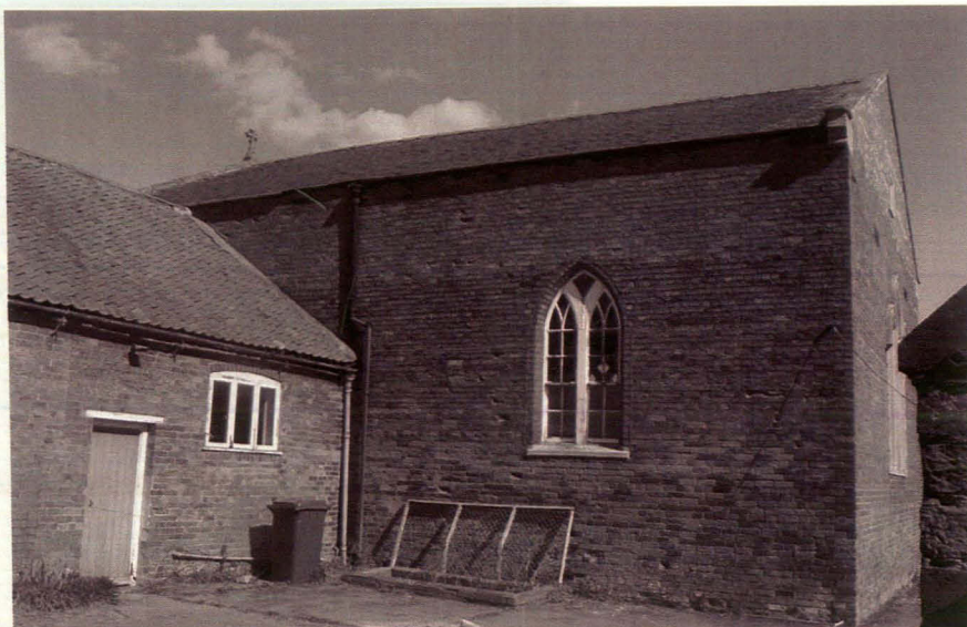
Plate 7 Western elevation of church, looking east
