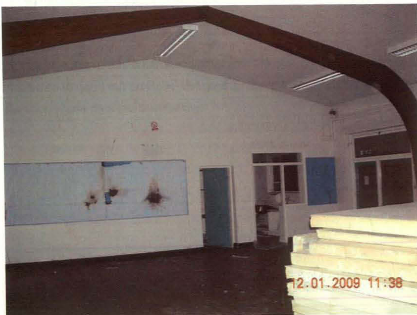
Plate 36 Northeastern extension, large hall, looking north
