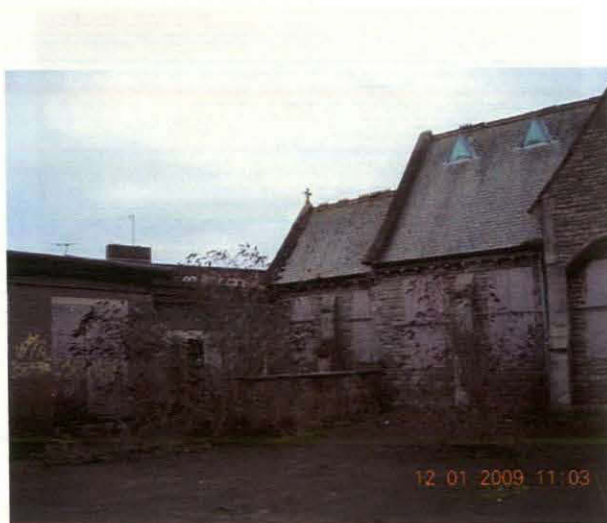
Plate 6 Northern elevation of chancel, showing cross finial, looking east
