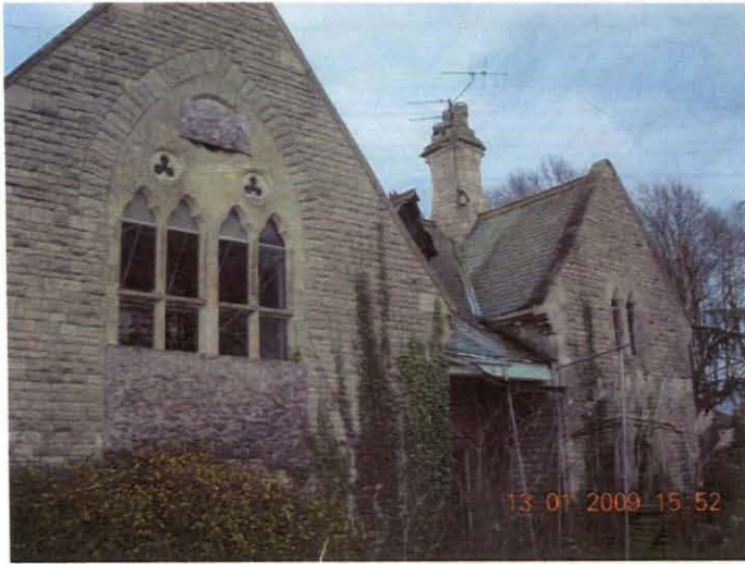
Plate 30 Western elevation, chapel and school house, looking southeast
