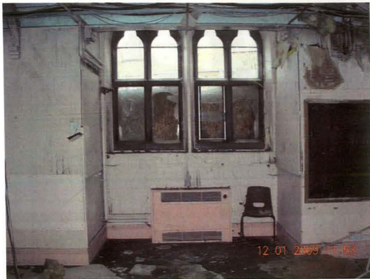
Plate 22 Alcove in school room, looking east
