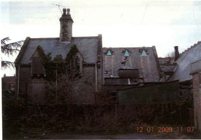
Plate 31 School house, southern elevation, looking north
