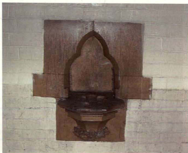
Plate 17 Chancel, piscina looking south
