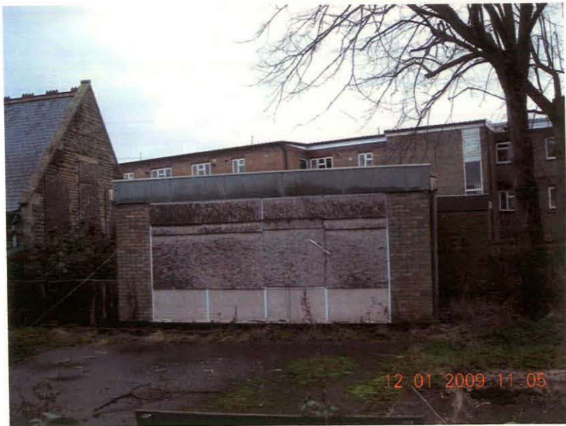
Plate 34 Extensions to southeast, looking east
