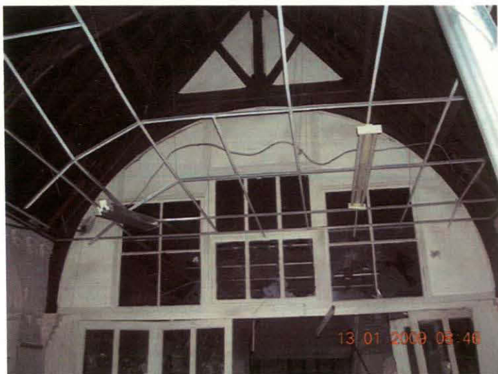
Plate 7 Nave interior, showing roof truss and inserted modern partition, looking east
