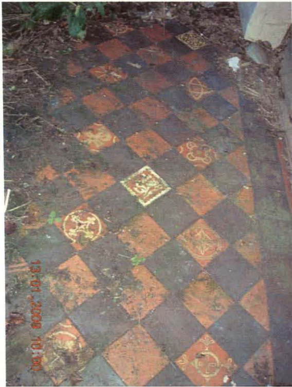
Plate 27 School house porch floor, looking north
