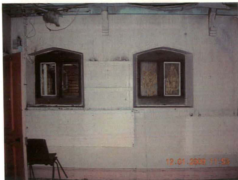
Plate 23 Windows in school room, looking east
