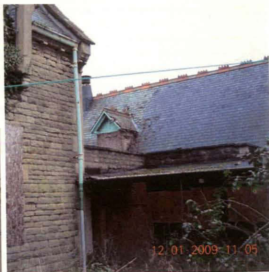
Plate 25 External wall and doorway to room south of nave, looking north
