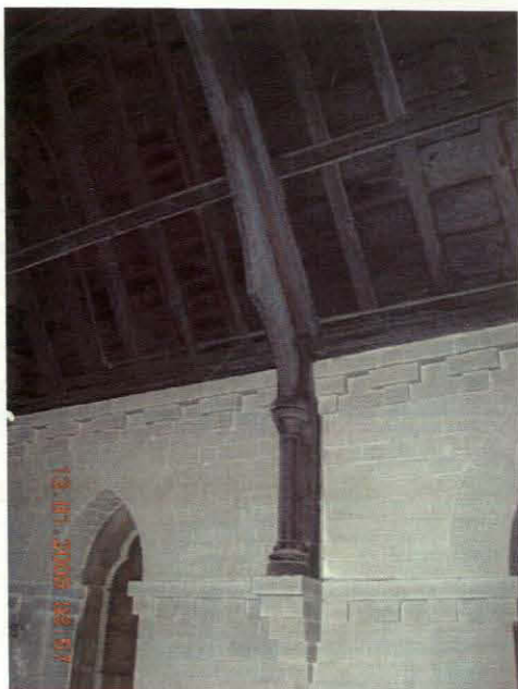
Plate 9 Detail of truss support timber in chancel, looking northwest
