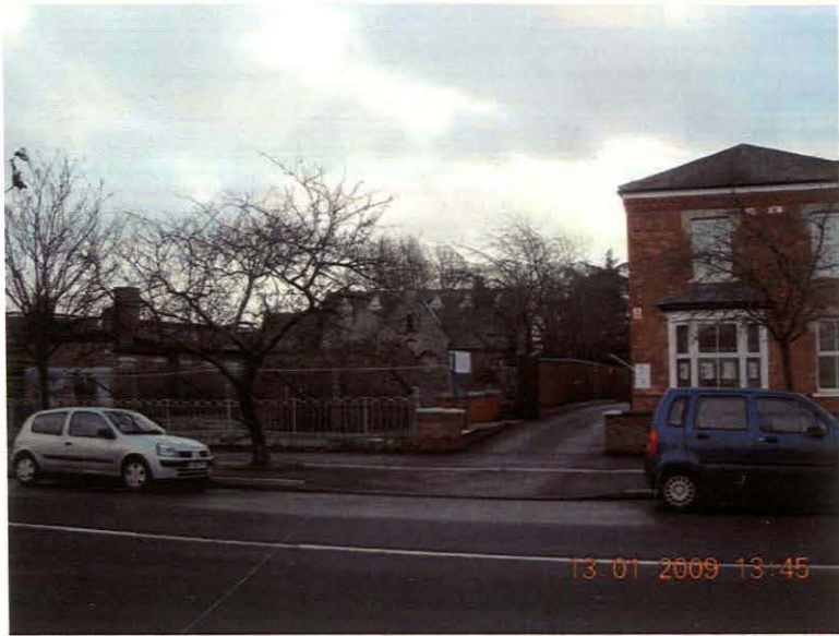
Plate 1 General view of school frontage, looking southeast
