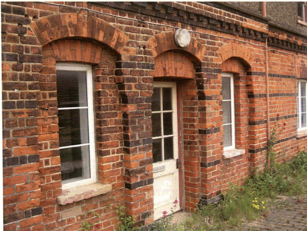
Plate 5 Block 2, southern entrance, looking northeast
