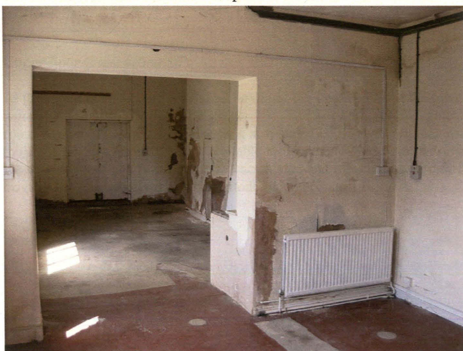
Plate 16 View from Room 2 to Room 1, looking west
