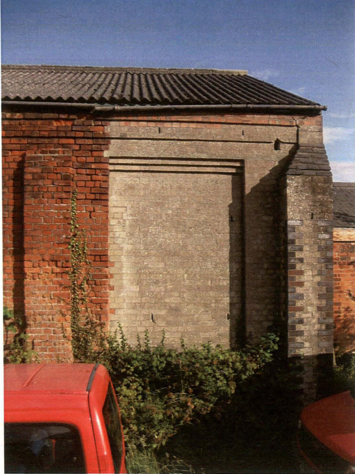
Plate 26 Western end of northwestern elevation, showing repair, looking southeast
