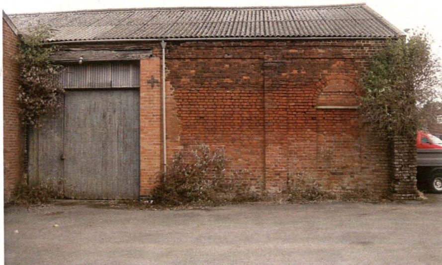
Plate 29 Eastern end of southeastern elevation of goods shed, looking northwest
