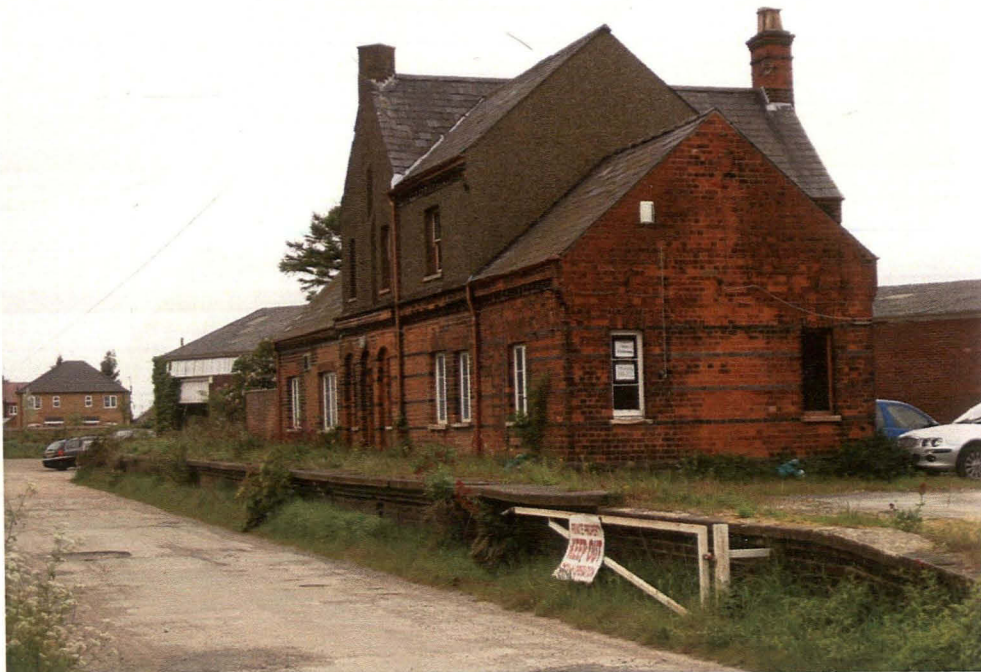
Plate 6 General view of southern and eastern sides of station house, looking northwest
