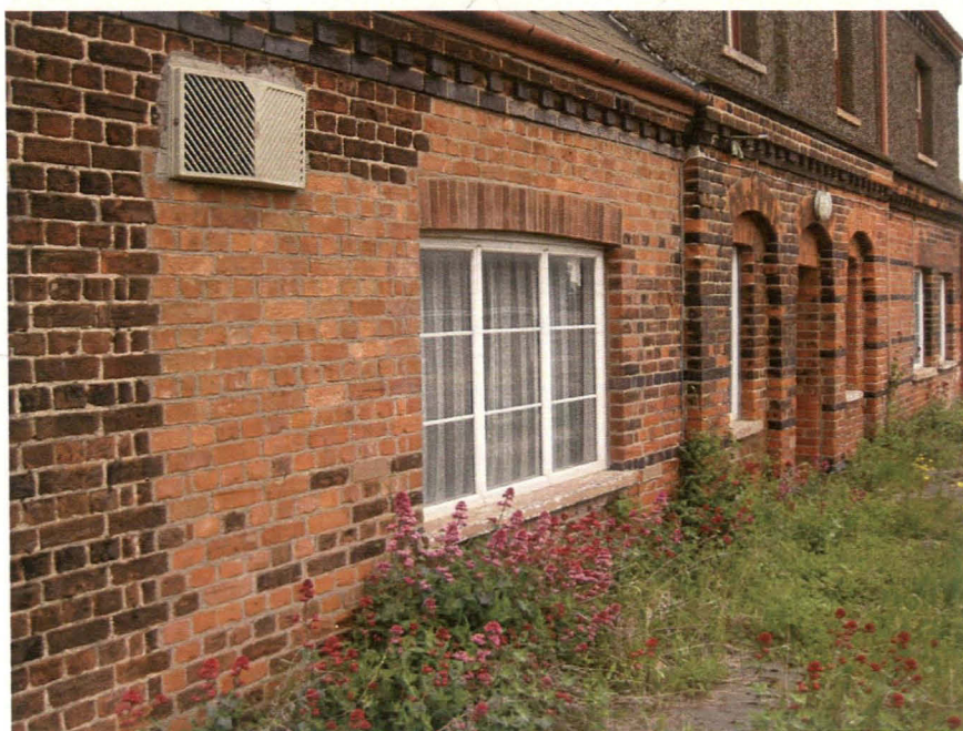
Plate 4 Block 1 (foreground), showing brick patching and inserted window, looking northeast
