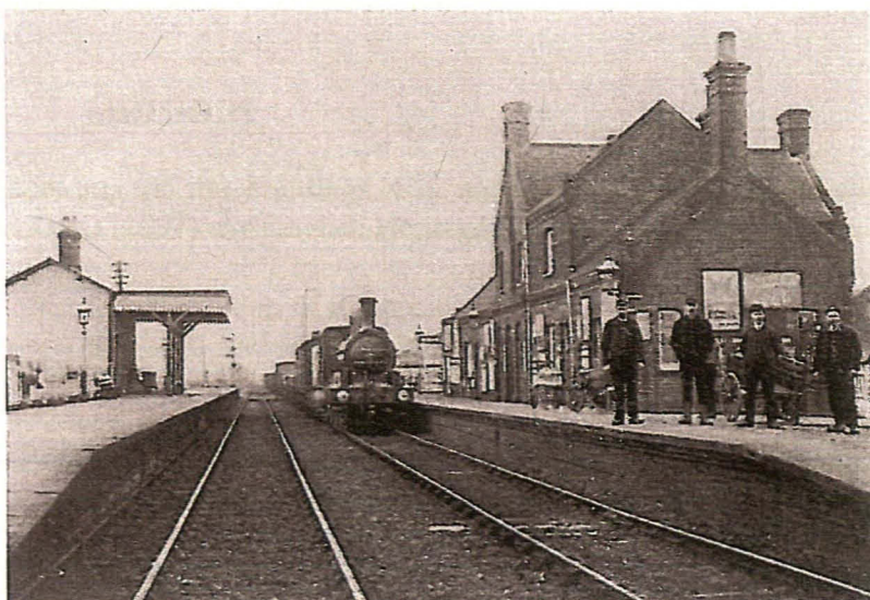
Plate 2 Holbeach Station House, c. 1906
