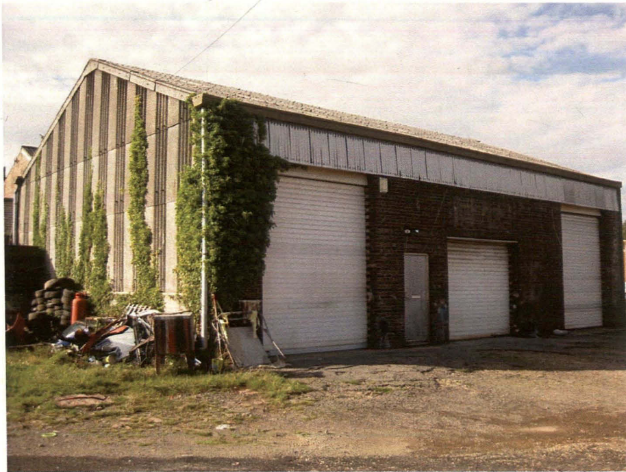
Plate 32 Western and southern sides of Block 3, looking north
