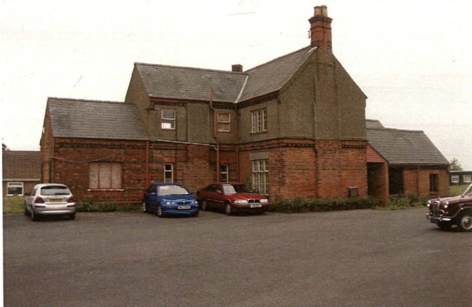
Plate 10 General view of northern elevation of station house, looking southwest
