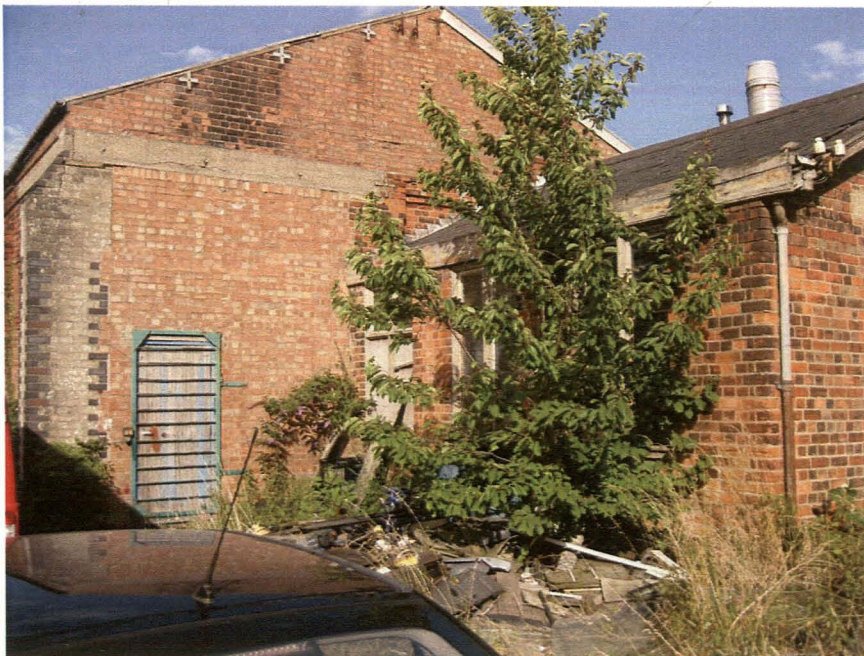
Plate 27 Southwestern elevation of goods shed, and attached Block 2, looking east
