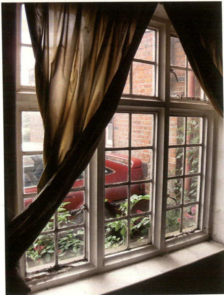
Plate 14 Room 8, detail of mullioned and transomed window, looking east
