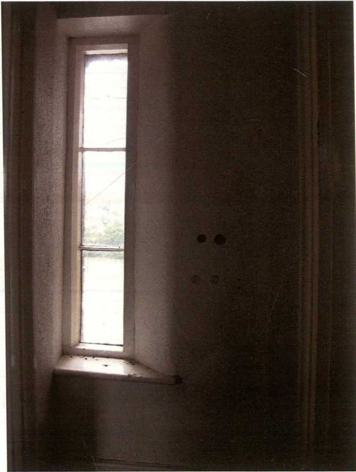
Plate 18 Narrow window on landing at top of stairs, looking northeast
