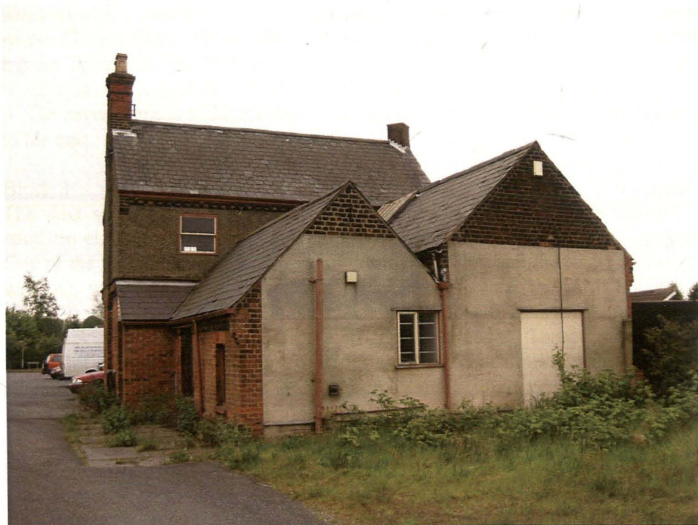
Plate 7 General view of western elevations of station house: Block 1 right foreground; Block 5 left foreground; Upper part of Block 2 to rear, looking east
