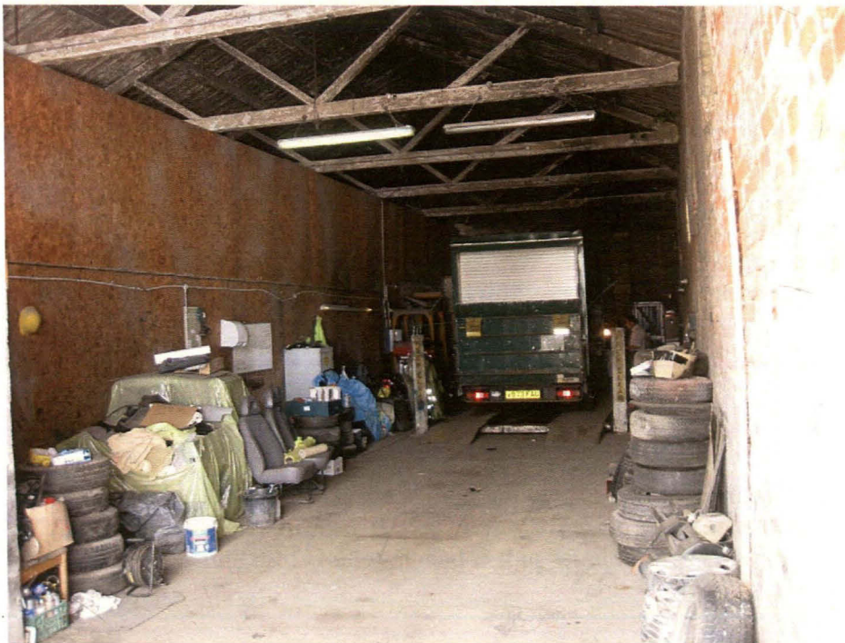
Plate 34 Goods shed Room 1, showing roof trusses and inserted partition, looking west
