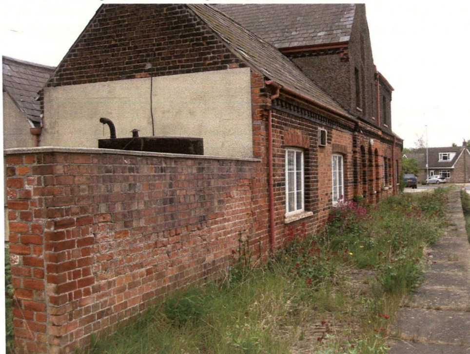
Plate 3 Southern façade of station house, and western gable end of Block 1, with boundary wall in foreground, looking northeast
