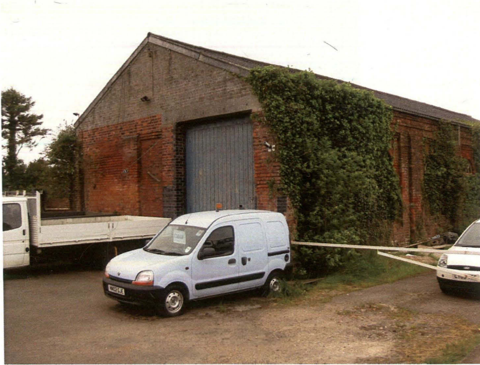
Plate 24 Goods shed, northeastern and northwestern elevations, looking south
