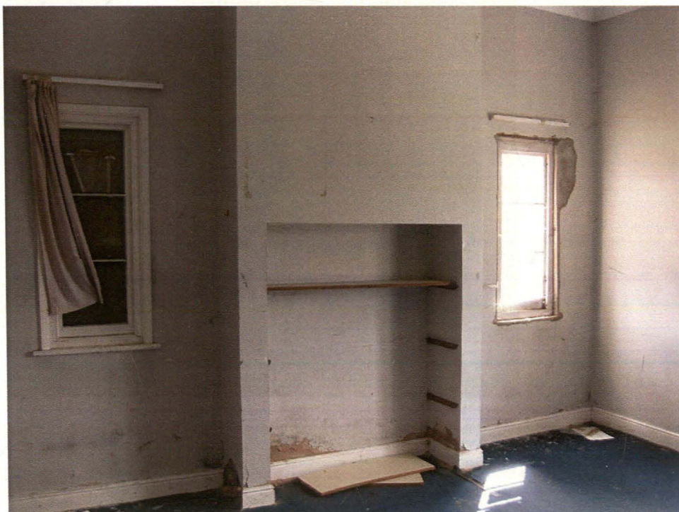
Plate 17 Room 7, showing former fireplace and windows, looking east
