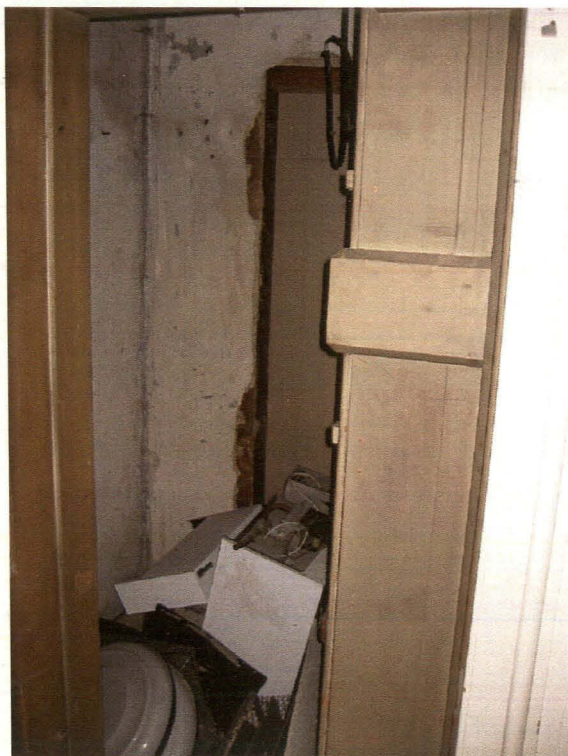
Plate 23 Room 16, storage area, showing blocked opening at rear, looking north
