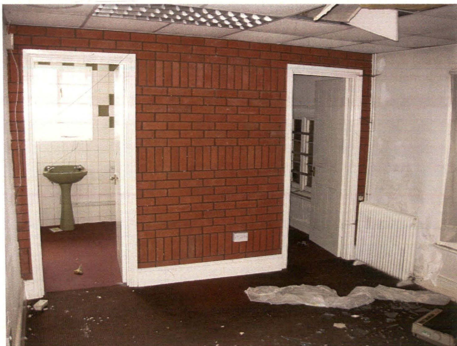
Plate 15 Room 9, view towards inserted partition and Rooms 10 (right) and 11(left), looking west
