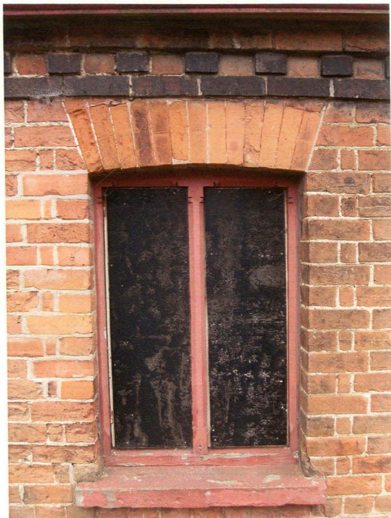
Plate 12 Carved window glazing bar, Block 5, northern elevation, looking south
