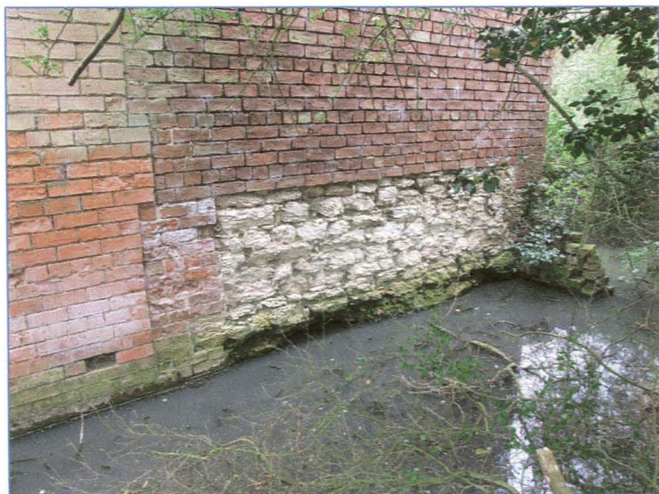
Plate 21: Chalk blocks in the south-east corner of the south range. Looking north. Note also the difference in brickwork at the left of the shot.
