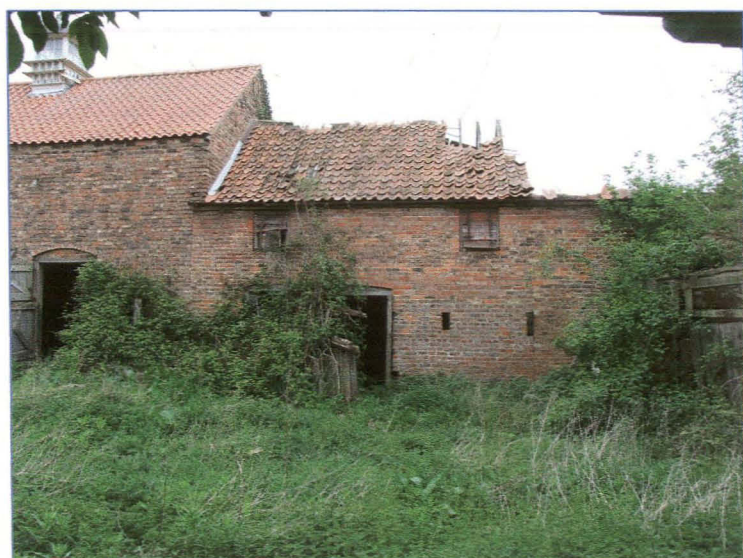
Plate 5: Stable block and hayloft in the south elevation of the north range. Looking north-north-west.
