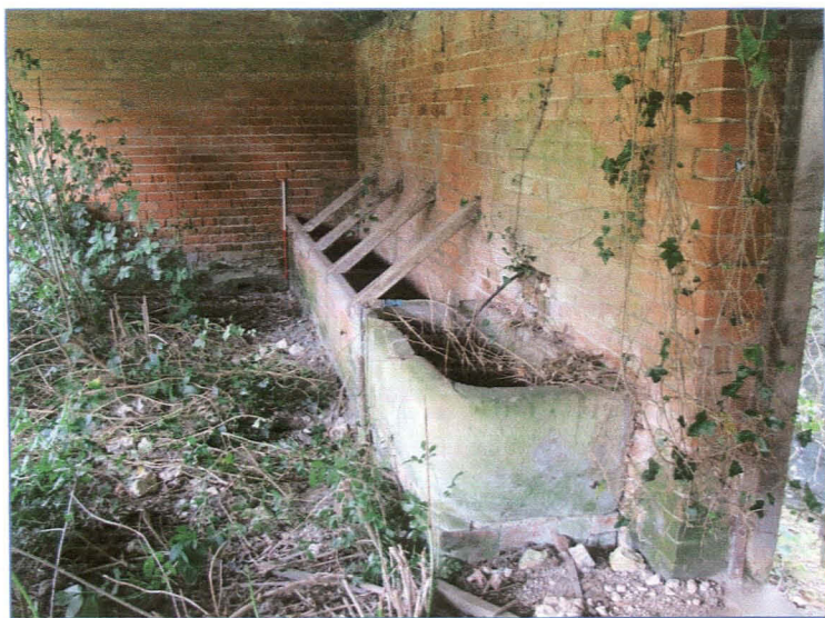
Plate 24: Feed trough and water trough at the east end of the south wall in the middle bay of the south range. Looking east.
