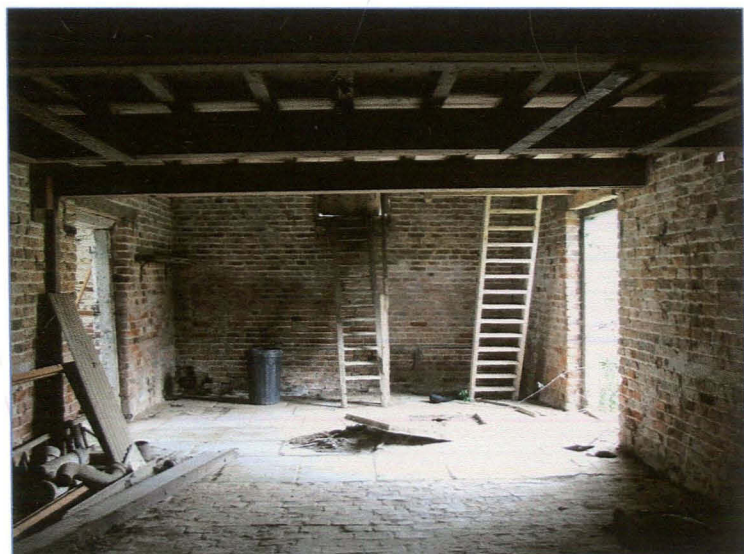
Plate 11: Ground floor of the threshing barn, looking east-north-east towards the flagstone threshing floor, with the large doors at either side allowing the through-flow of air to carry away the chaff.
