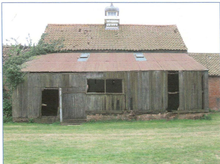
Plate 9: Lean-to on the north elevation of the north range. Looking south-south-east.
