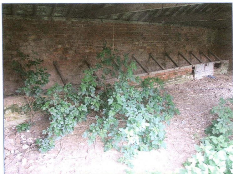
Plate 26: Feed troughs along the south wall of the western bay of the south range. Looking south.
