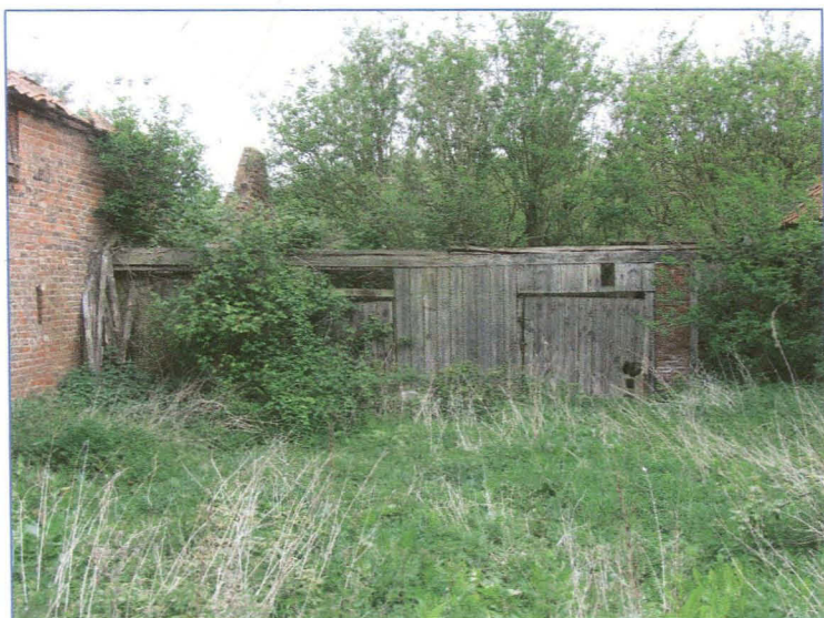
Plate 20: West elevation of the barn at the east end of the crew yard. Looking east-north-east.
