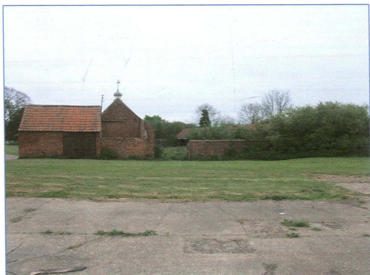
Plate 27: West elevation of the barns, showing the outbuildings at the end of the north range and the boundary wall attached to the south range, with the gates between. Looking east-north-east
