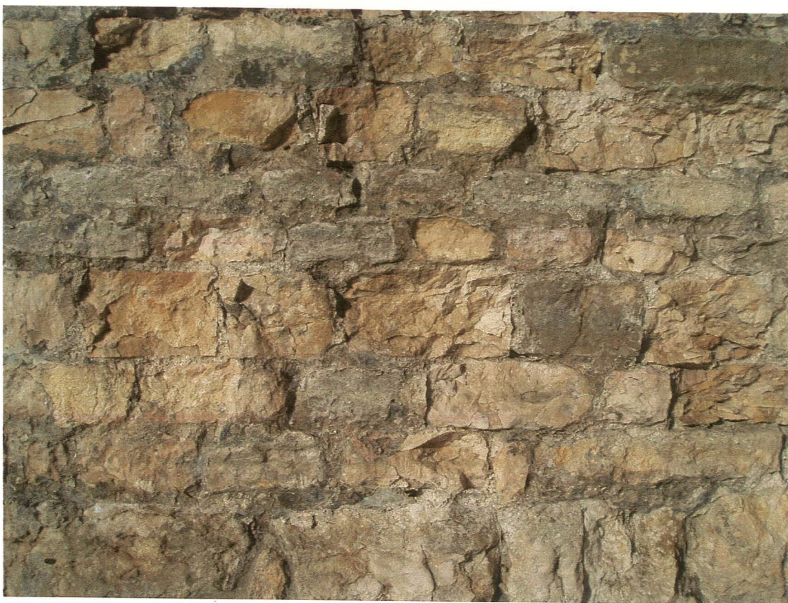
Pl. 7. Detail of medieval fabric of upper Close Wall 104. Looking north
