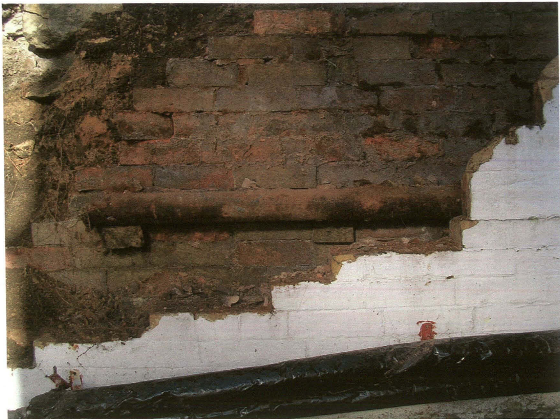
Pl. 5. Surviving orangery wall. Looking north
