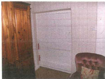
19. A nice example of an 18 th century boarded and ledged back door, with 18 th century latch and strap hinges, within Room 6 (Unit 1), taken from the south-west
