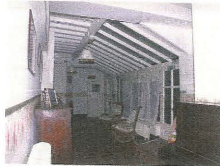
34. Corridor of Unit 4 showing former conservatory features, taken from the south
