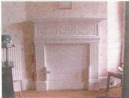
163. Detail of fireplace in Room 59, taken from the north-west
