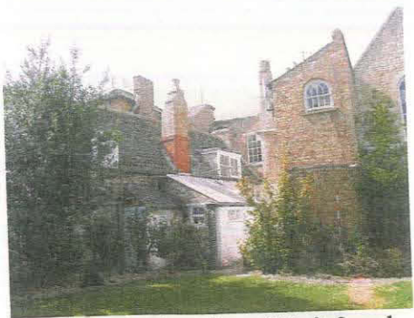
113. North elevation of Unit 8 and east elevation of Unit 8 (left) and Unit 7, taken from the north-east
