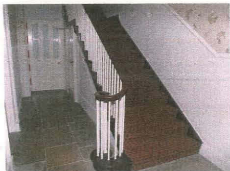
11. Open string stair in hall of Unit 1, taken from the north-west
