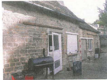
105. South elevation of Unit 8, taken from the south-west
