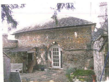
117. South elevation of outbuilding, taken from the south
