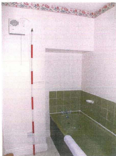
154. Room 55 showing position of possible former doorway, taken from the south-east
