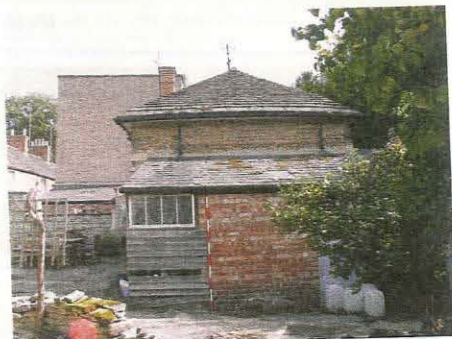
116. West elevation of outbuilding, taken from the west
