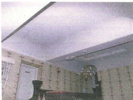
147. Ceiling of hall (Unit 4), taken from the north-west
