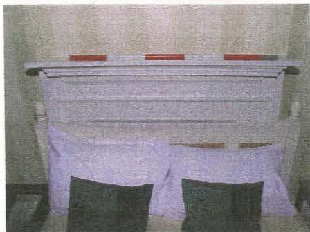
81. Detail of mantel shelf with fine dentilated moulding in Room 34, taken from the north
