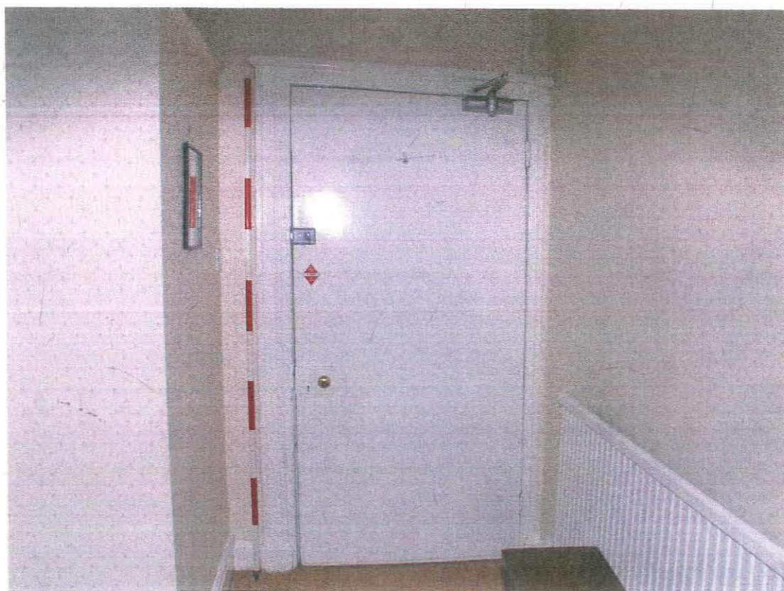
Plate 22 Detail of door (Room 40) showing moulded panel on the left jamb and possibly 19 th century rim-lock, taken from the west (89)
