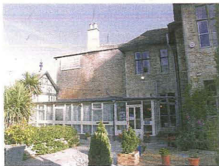
92. South elevation of Units 5, 6 and 13, taken from the south
