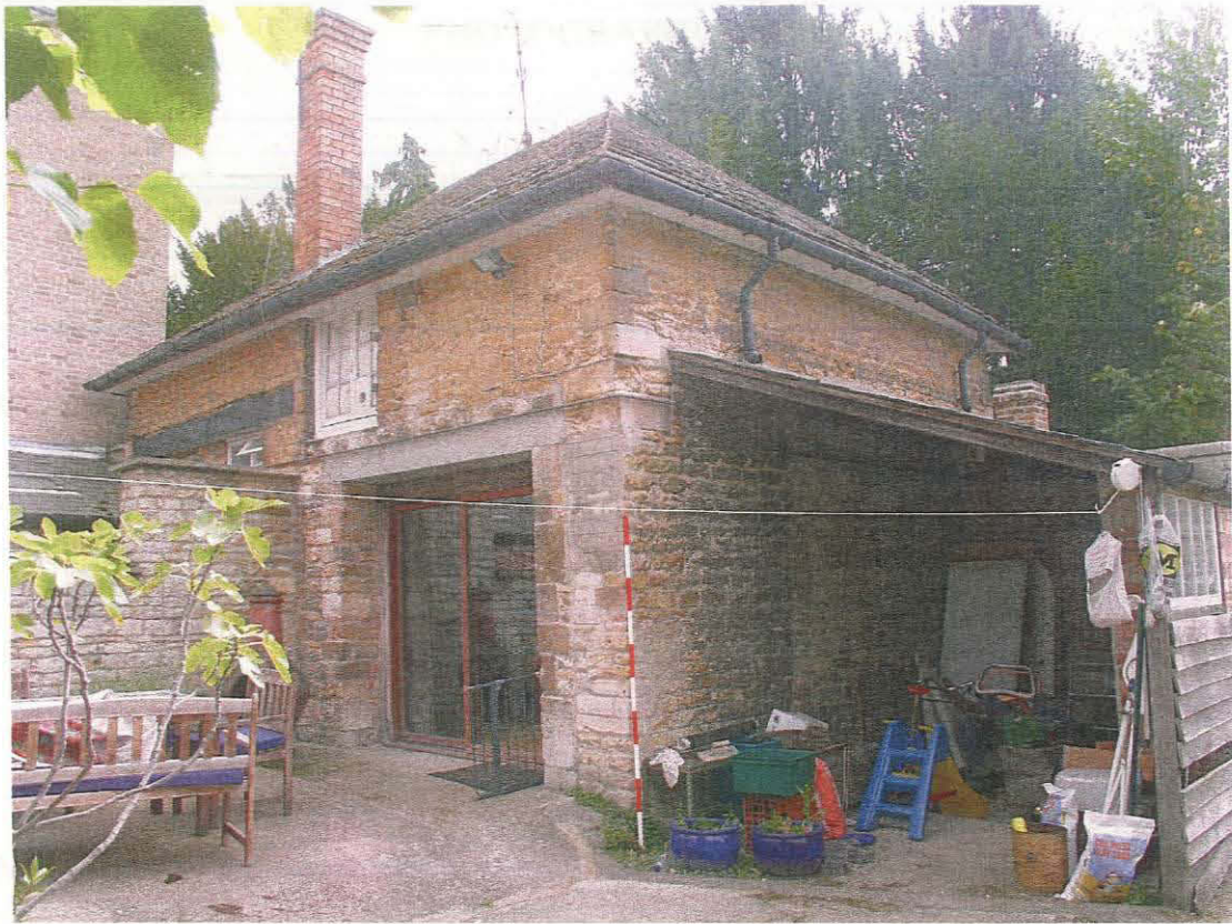
Plate 37 North elevation of outbuilding, taken from the north-west (125)
