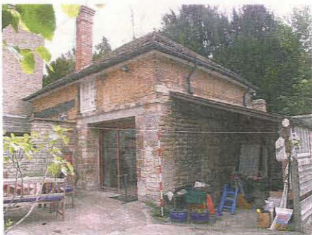
125. North elevation of outbuilding, taken from the north-west
