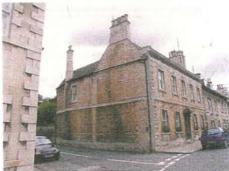
127. North elevation of Unit 1, taken from the north-west
