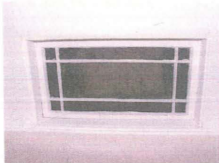
159. Detail of roof light in corridor (Unit 14) showing 19 th century etched glass, taken from the north
