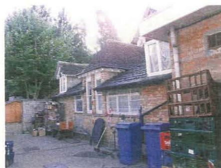
103. North elevation of Unit 11, taken from the north-west
