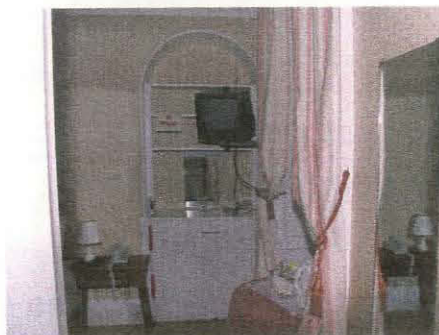
10. Cupboard with a two leaf door in the recess west of the fireplace in Room 3, taken from the north
