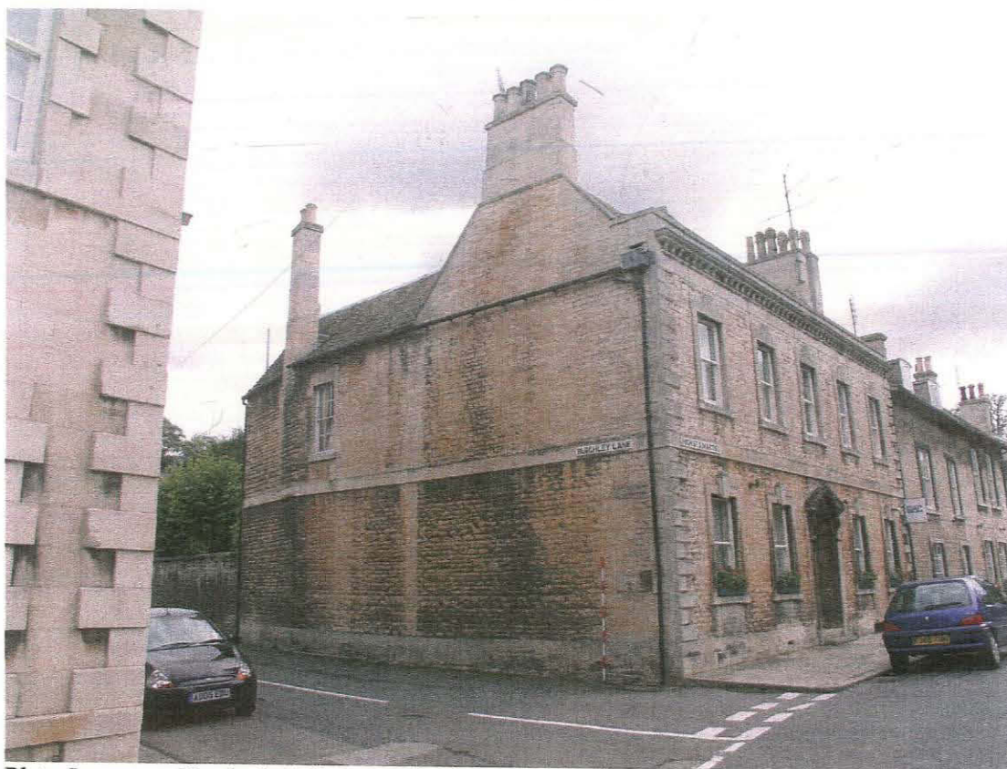
Plate 5 North elevation of Unit 1, taken from the north-west (127)
