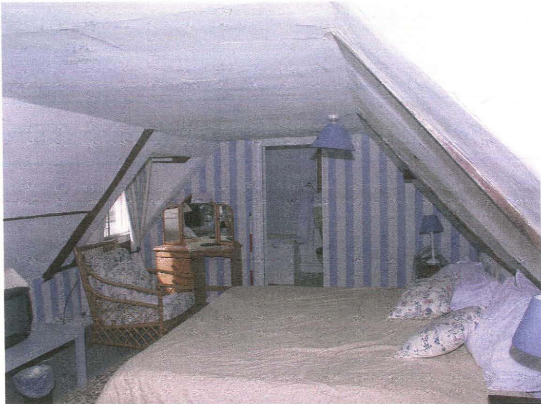
Plate 31 Room 63 (Unit 1) showing principal rafters with joggled butt purlins and dormer window, taken from the south-east (171)
