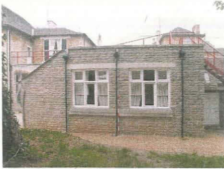
95. East elevation of Unit 12, taken from the east
