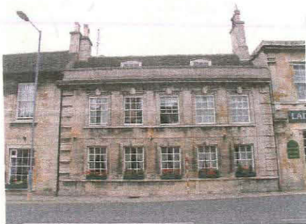
109. West elevation of Unit 4, taken from the west
