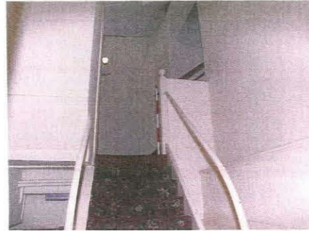
132. Stairway between ground floor and first floor of Unit 2, showing simple iron handrail and ball finial, taken from the east
