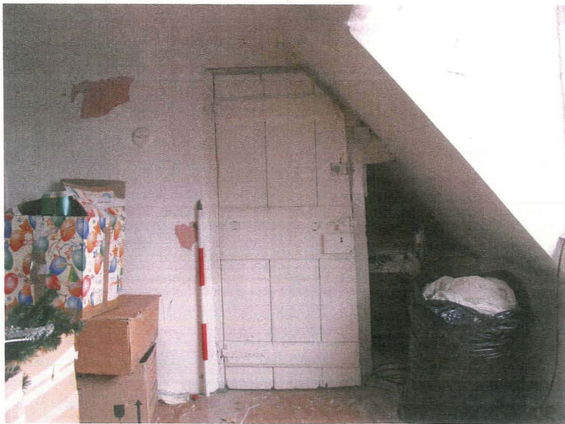
Plate 34 Detail of door (Room 68), taken from the north (146)
