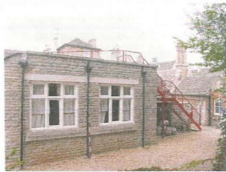
96. East elevation of Unit 12 and south elevation (east end) of Unit 8, taken from the south-east
