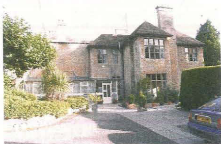
91. South elevation of Units 5, 6, 13 and 14, taken from the south
