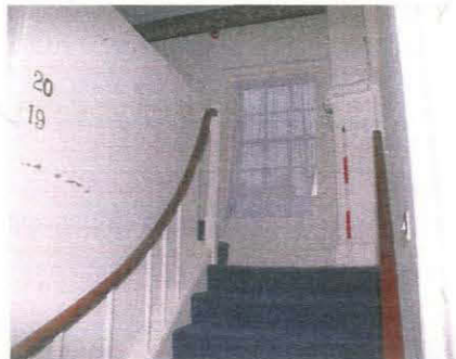
135. Shared stair of Units 2 and 3 between the first floor and second floor, taken from the south-west
