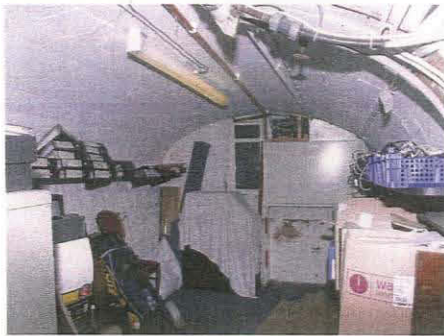
17. Room 7 (cellar room of Unit 1), taken from the north-east
