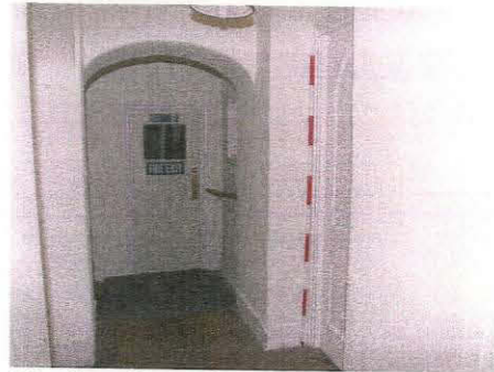
26. Corridor of Unit 2, taken from the south
