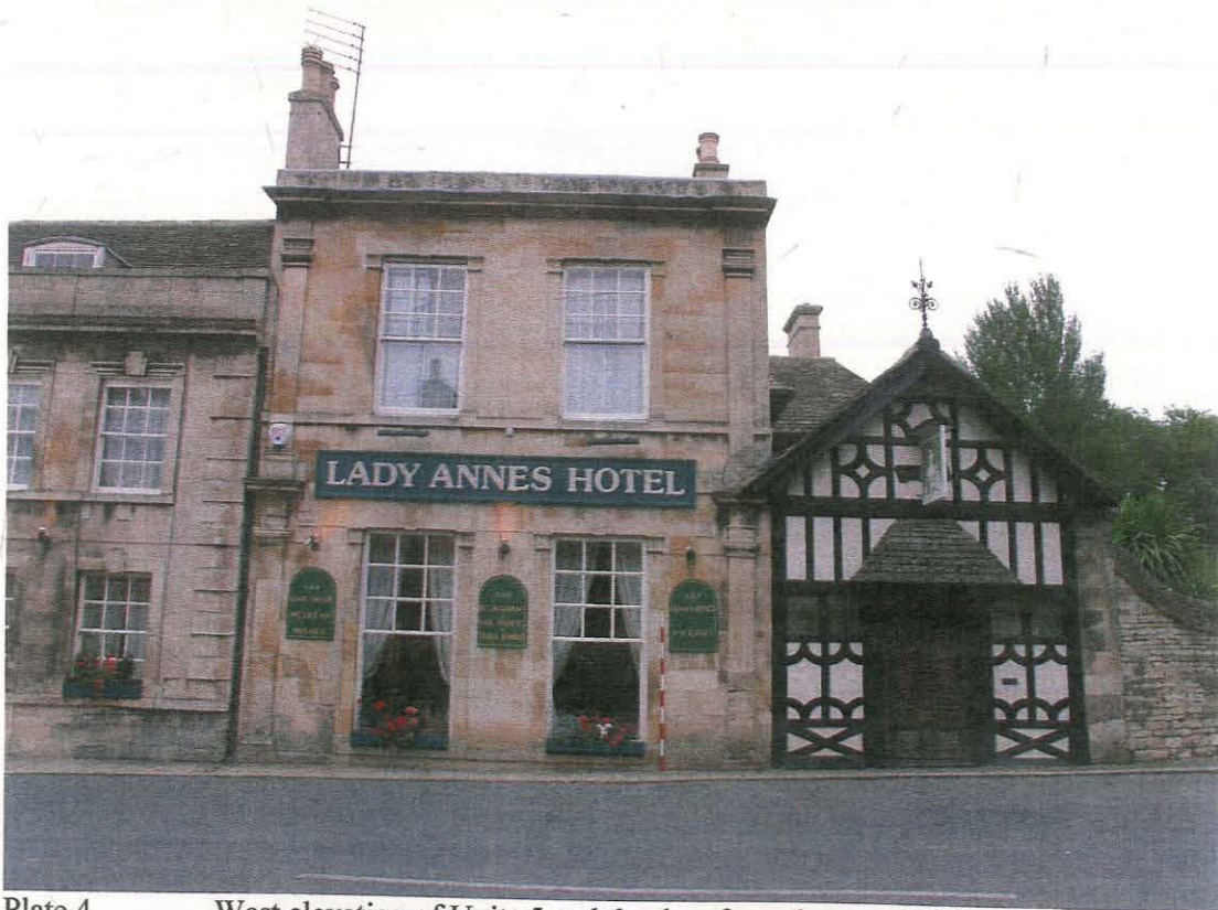
Plate 4 West elevation of Units 5 and 6, taken from the west (108)
