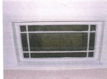
160. Detail of roof light in corridor (Unit 14) showing 19 th century etched glass, taken from the north
