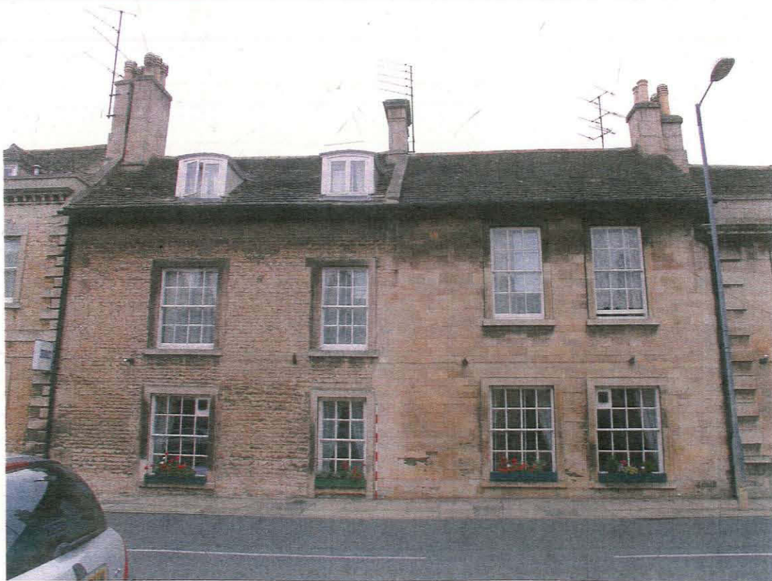
Plate 2 West elevation of Units 2 and 3, taken from the west (110)
