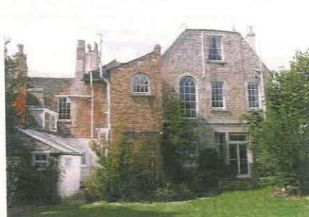
112. East elevation of Unit 7 (centre) and Unit 1, taken from the east
