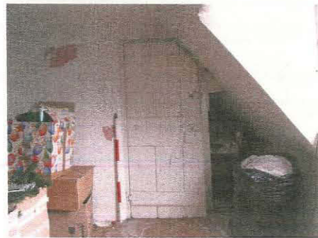
146. Detail of door (Room 68), taken from the north
