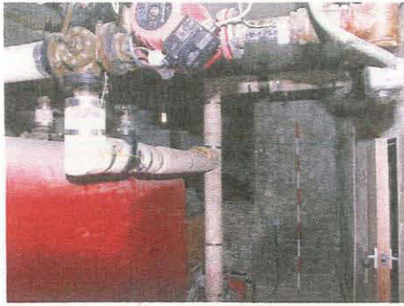
71. Cellar Room 71 (Unit 3), taken from the west
