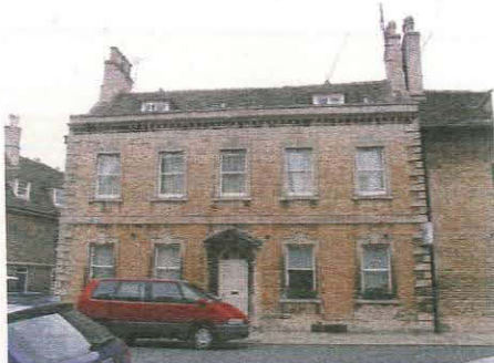
111. West elevation of Unit 1, taken from the west
