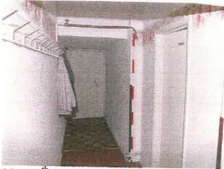
33. 19 th century red and buff coloured tiles at the west end of the corridor (Unit 11)
