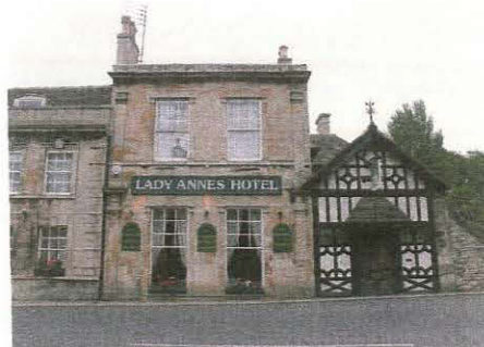
108. West elevation of Units 5 and 6, taken from the west
