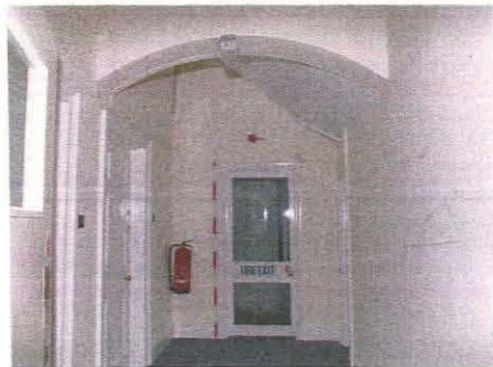
133. Landing of Unit 2, taken from the south
