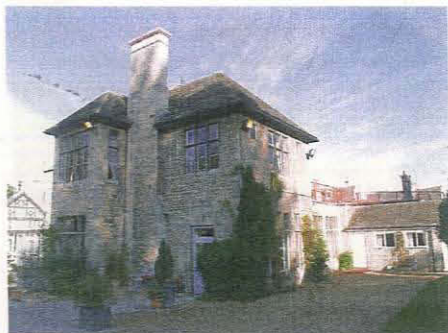
93. South elevation of Units 14 and 12 (right) and east elevation of Unit 14, taken from the south-east
