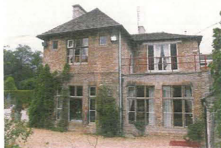
94. East elevation of Units 14 and 13 (top right), taken from the east
