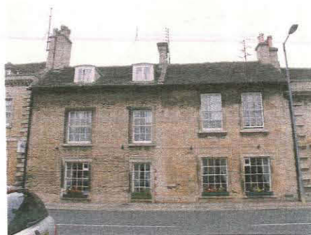
110. West elevation of Units 2 and 3, taken from the west
