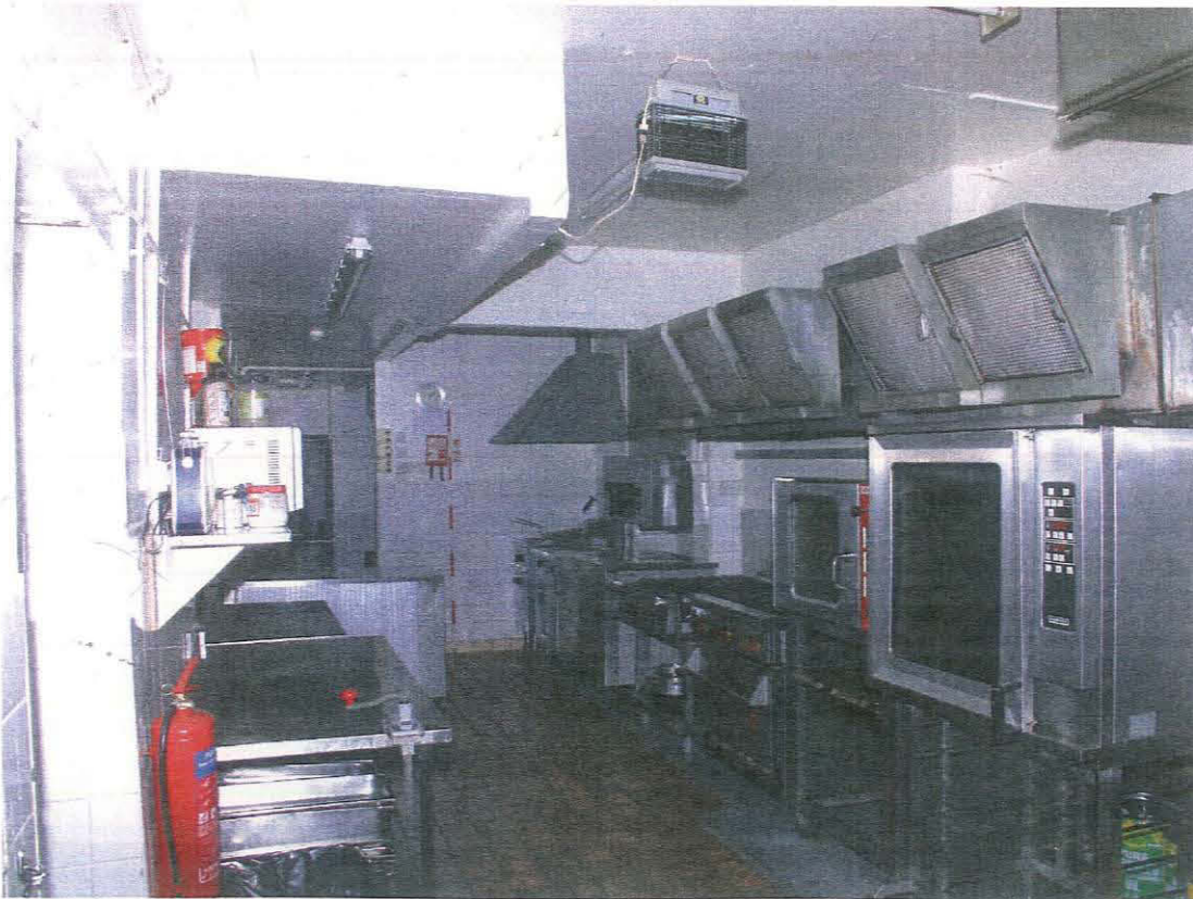
Plate 12 Room 15 (Unit 8) showing axial and co-axial beams, taken from the east (30)
