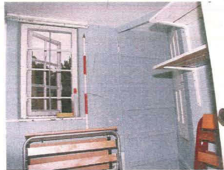
134. Room 43 (Unit 2), taken from the west
