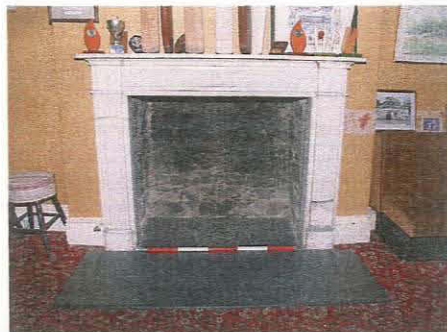
54. Detail of fireplace in Room 29, taken from the north
