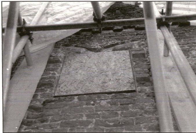
Plate 8: The garret window of the West Elevation showing the same architectural detailing as those of the ground floor. Note also, a second dentil string above the Dutch Arch.
