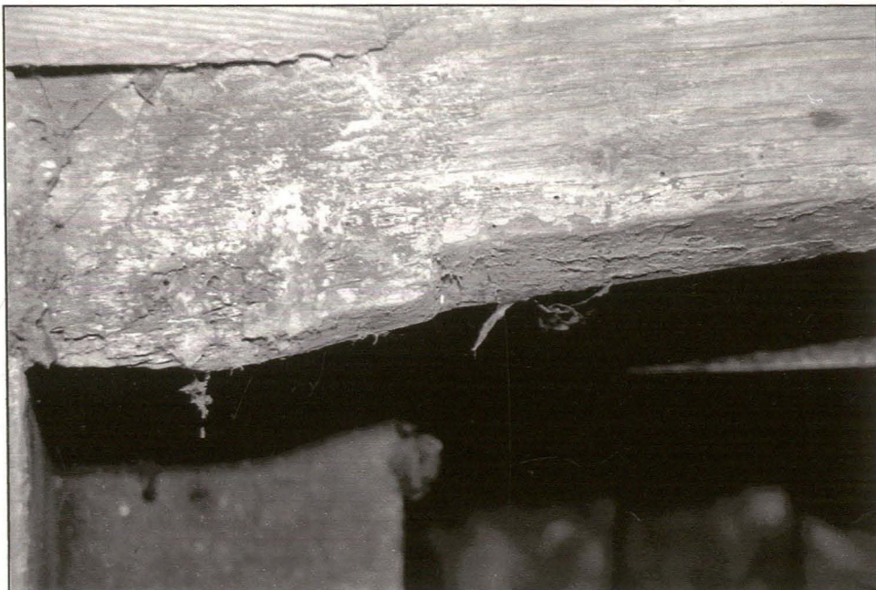
Plate 29: Detail of reverse ogee or cyma reversa, in this case from the east side, south end, of the surviving tiebeam.
