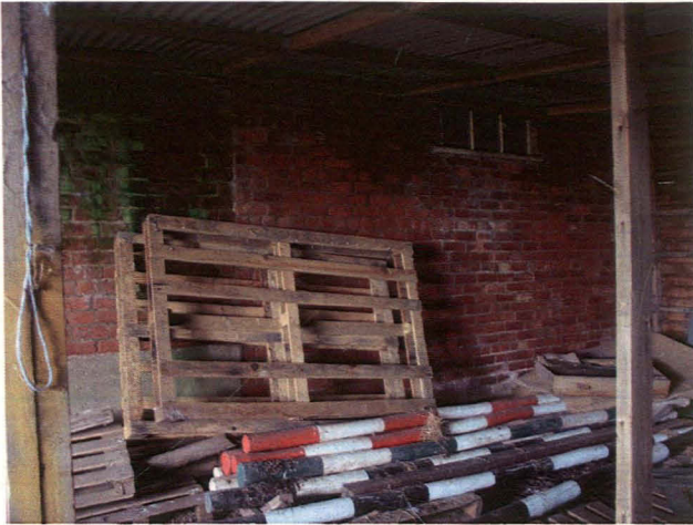
Plate 17 Interior of timber lean-to, showing straight join junction between NW-SE range (on right) and NE-SW range (to left), looking south
