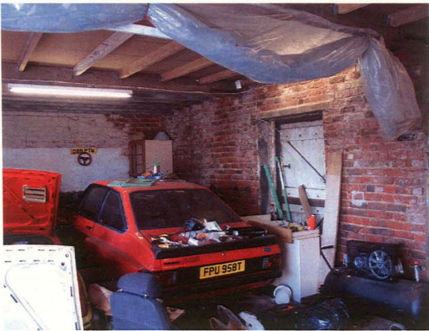
Plate 18 NE-SW Range, interior view, looking southwest
