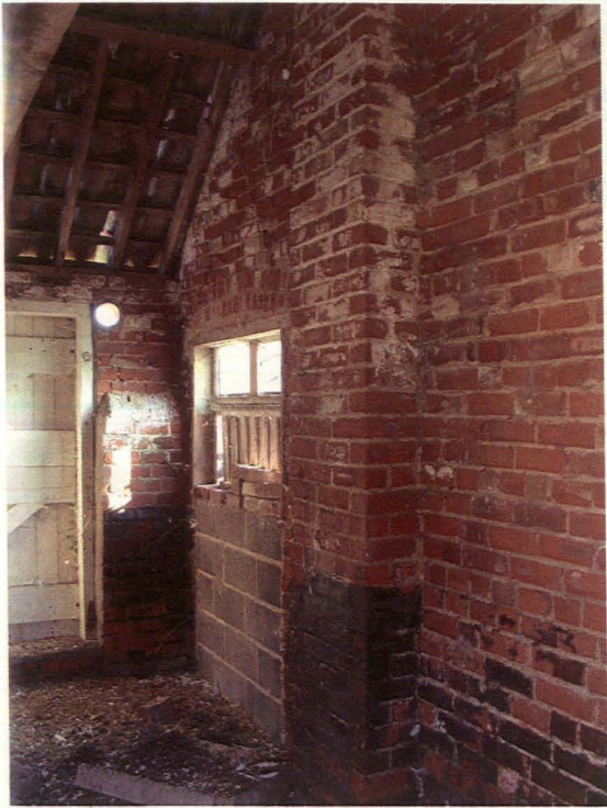
Plate 9 NW-SE Range, SE room, showing former fireplace and chimney and blocked door, looking northeast
