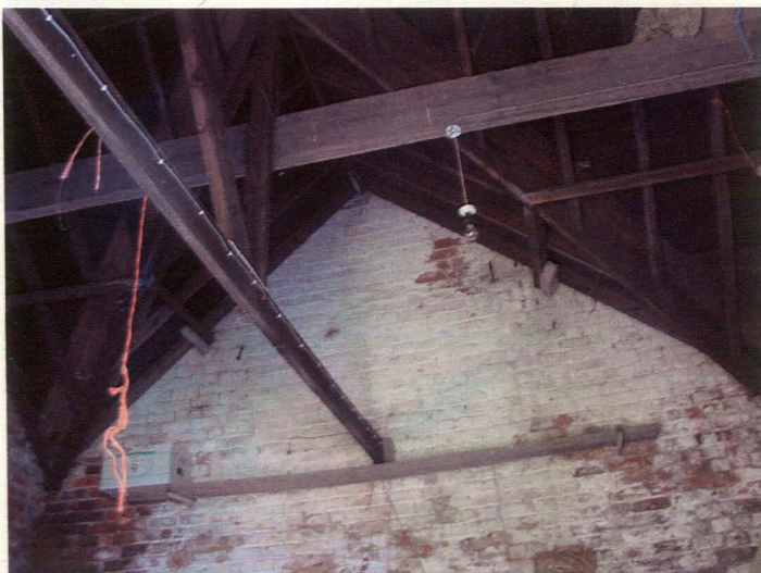
Plate 4 NW-SE Range, northwest room, showing roof timbering, looking northeast
