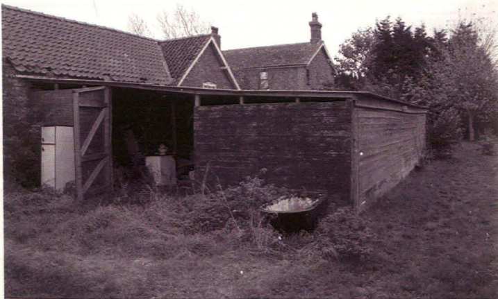
Plate 19 Timber Lean-to, northeastern elevation, looking south
