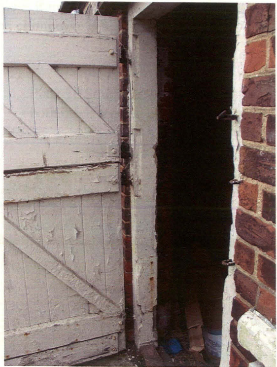
Plate 6 NW-SE Range, detail of door jamb rebates, looking north
