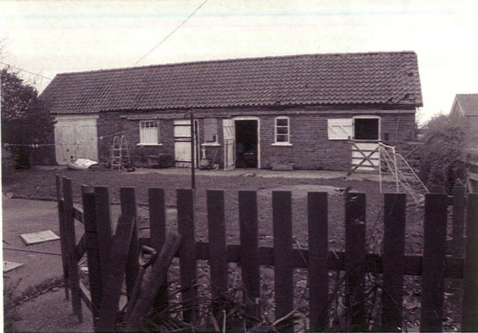
Plate 2 NW-SE Range, SW elevation, looking northeast
