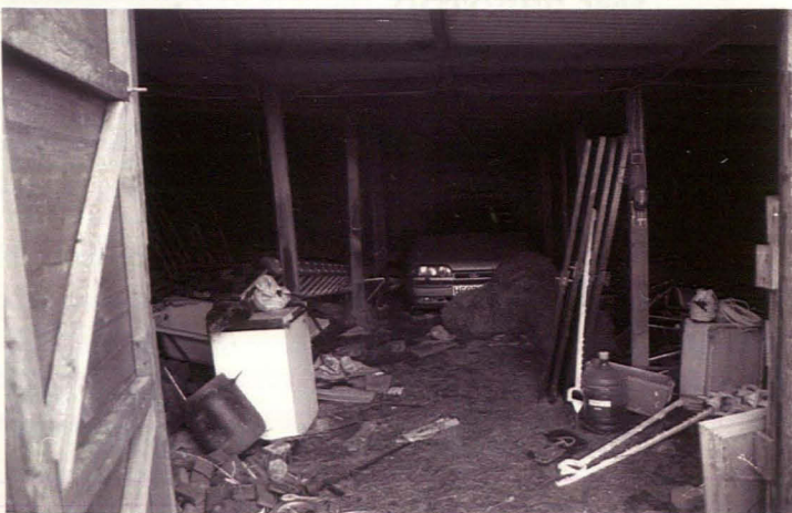
Plate 20 Timber Lean-to, interior, showing aisles, looking southwest
