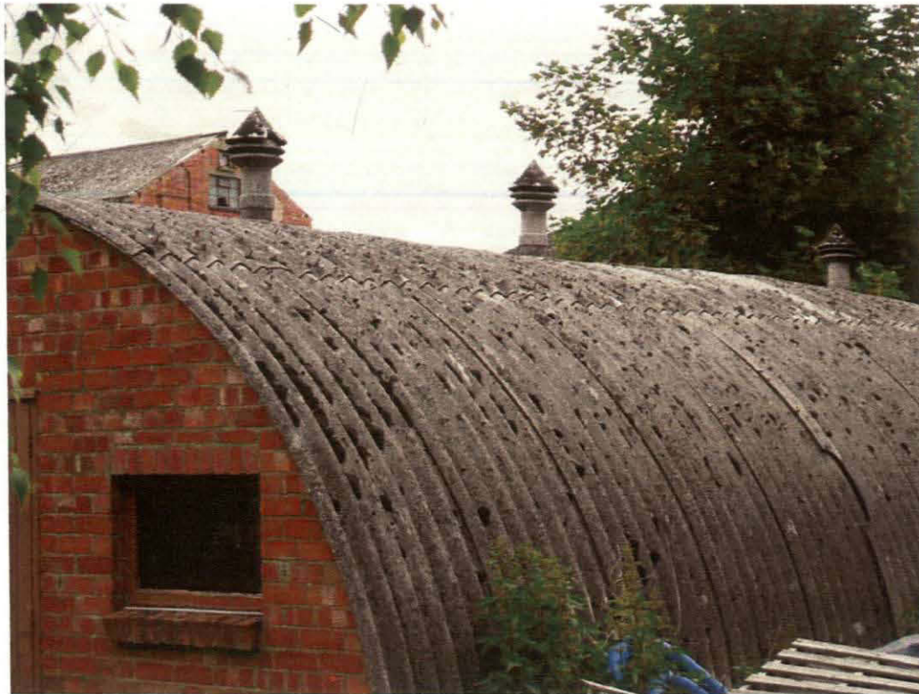
Plate 3 Detail of chimneys in Nissen hut roof, looking northeast
