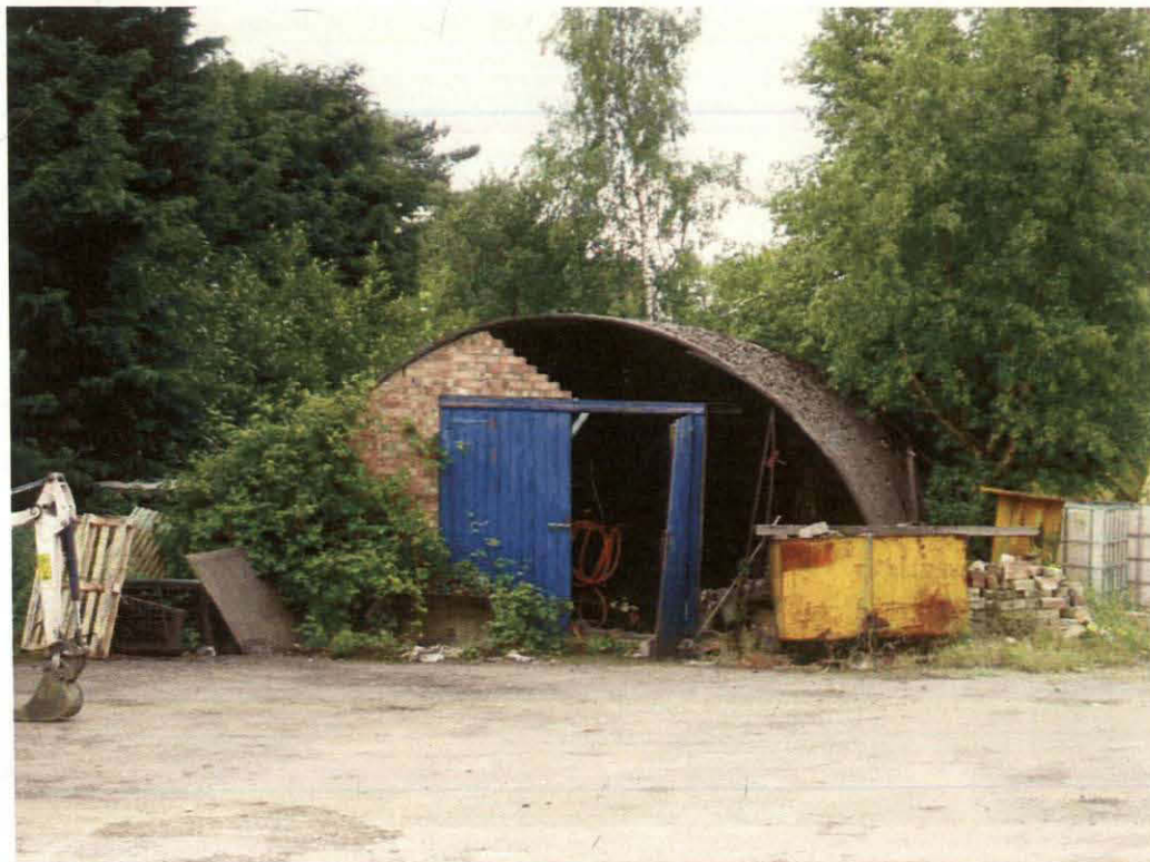
Plate 9 Eastern elevation of Room 2 of Nissen hut, looking west
