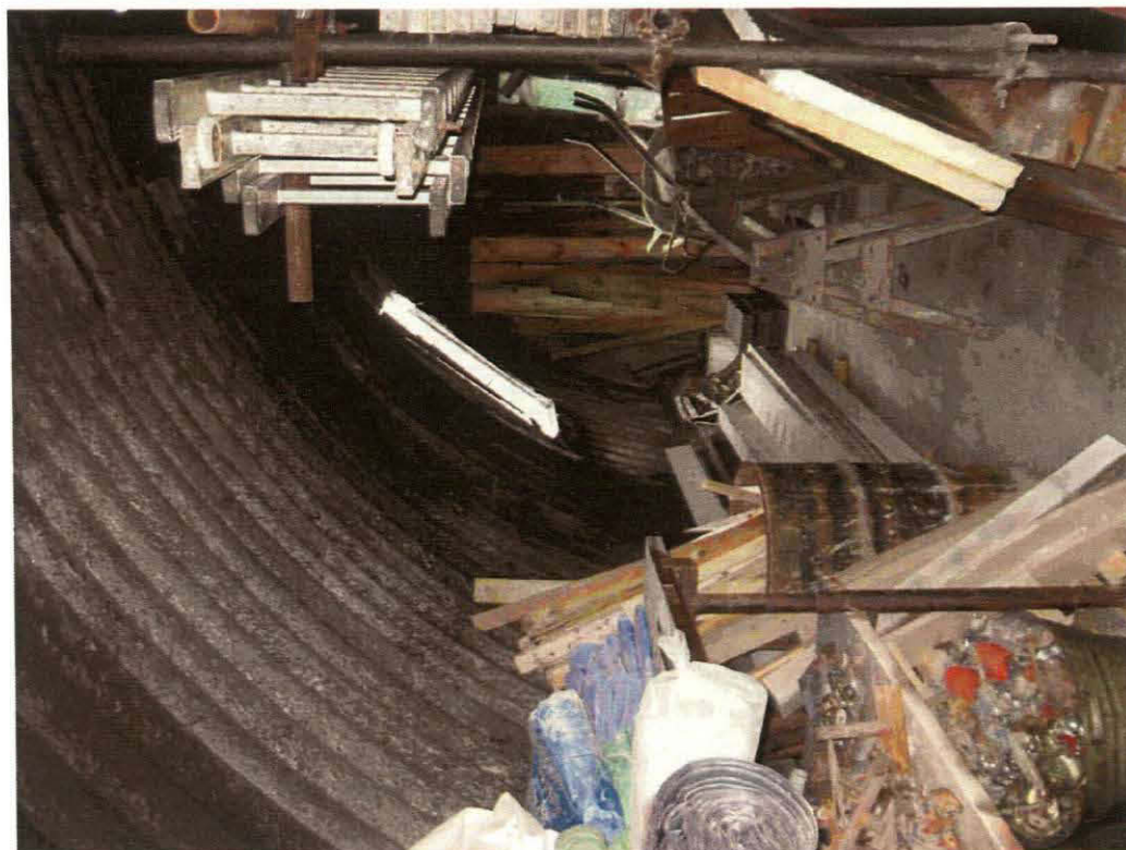
Plate 6 Interior of Room 1 of Nissen hut, north side, looking east
