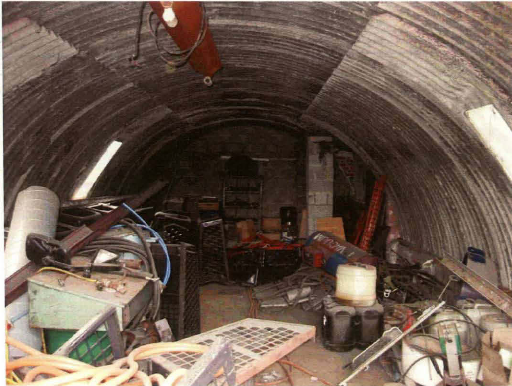
Plate 10 Interior of Room 2 of Nissen hut, view toward dividing wall, looking west
