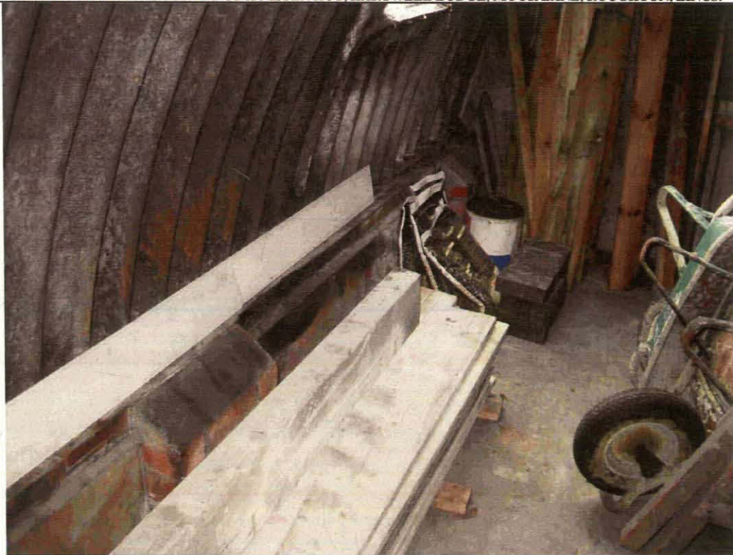
Plate 7 Detail of plinths in Room 1 of Nissen hut, looking east
