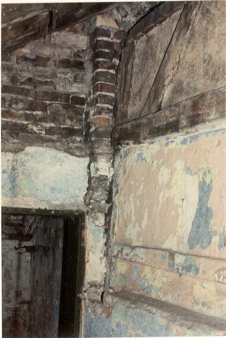
Pl. 30. East gable, clasp ing north-east corner of frame (plinth below), from west.
