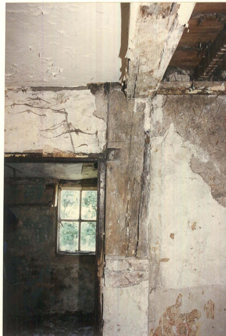
Pl. 47. Post and half-bricks on plinth wall in kitchen north wall.
