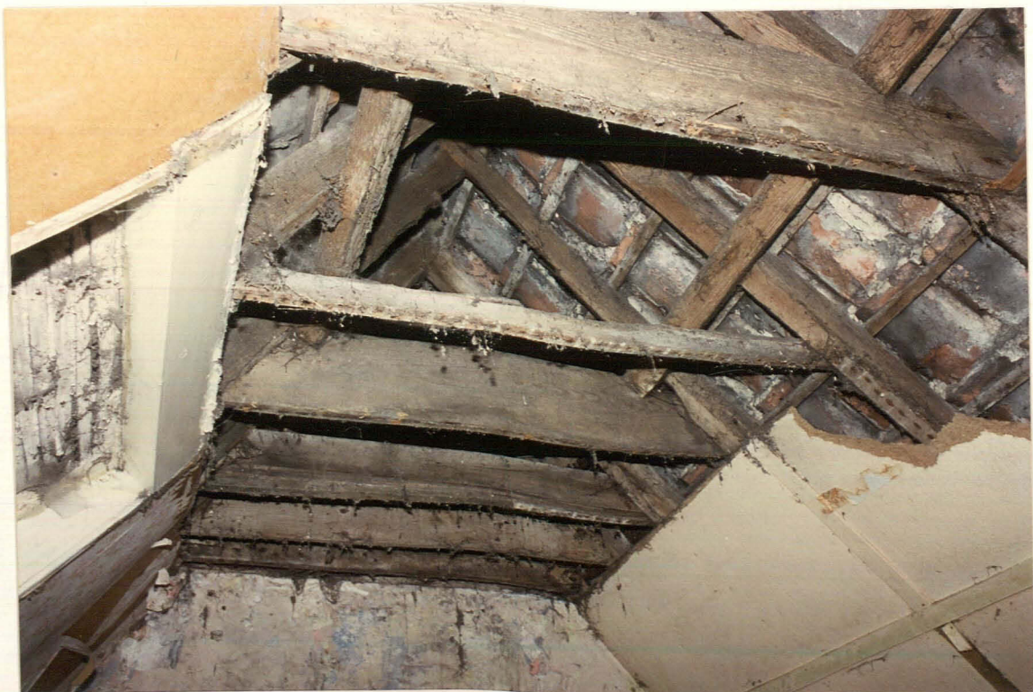
PI. 55. Roof at west gable: Nailed truss assembly, from east.
