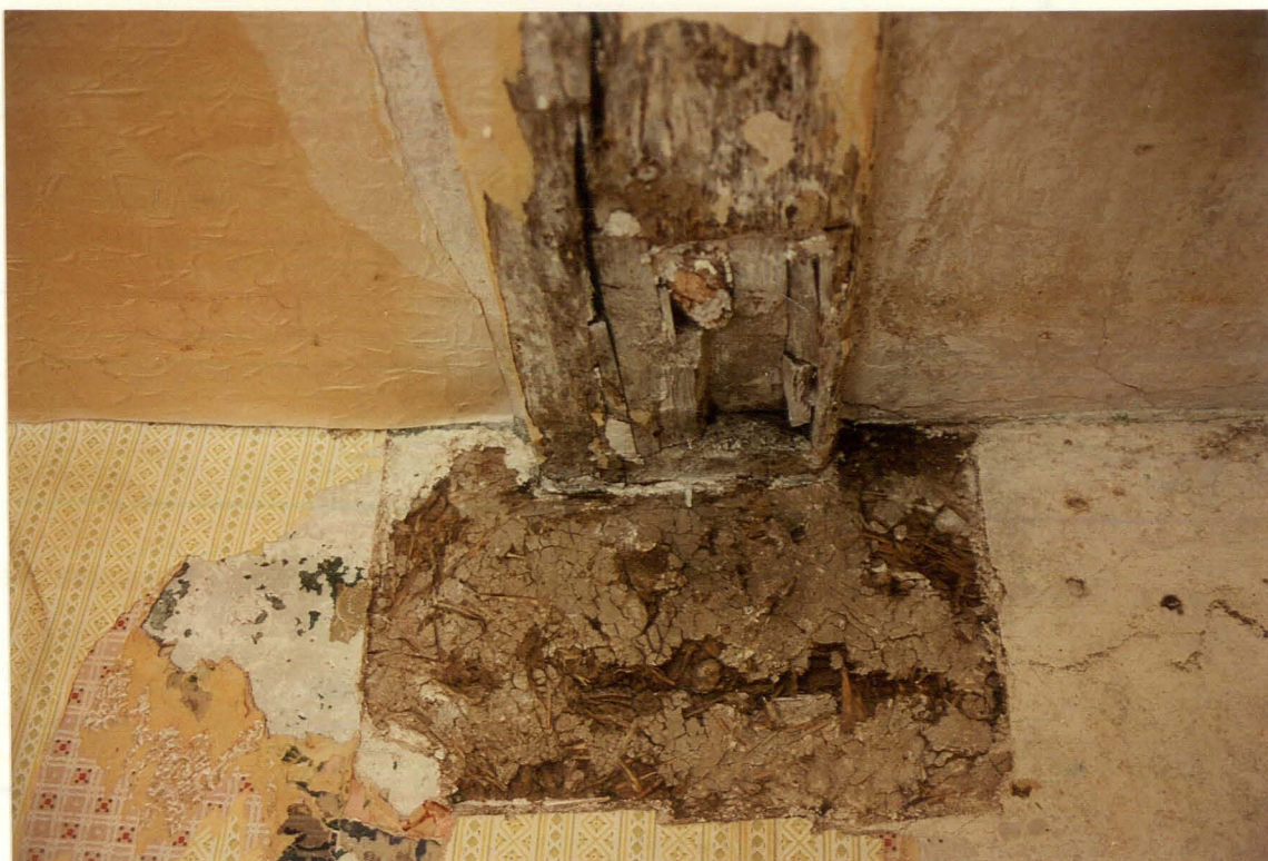
Pl. 43. West binder, north end; daub and unidentified joint (parlour).
