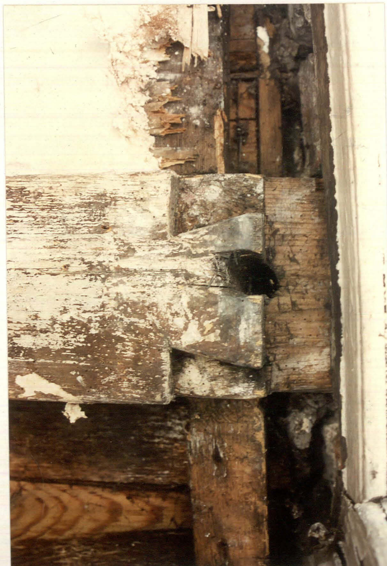
Pl. 46. West binder, south soffit, detail of dovetail (parlour).
