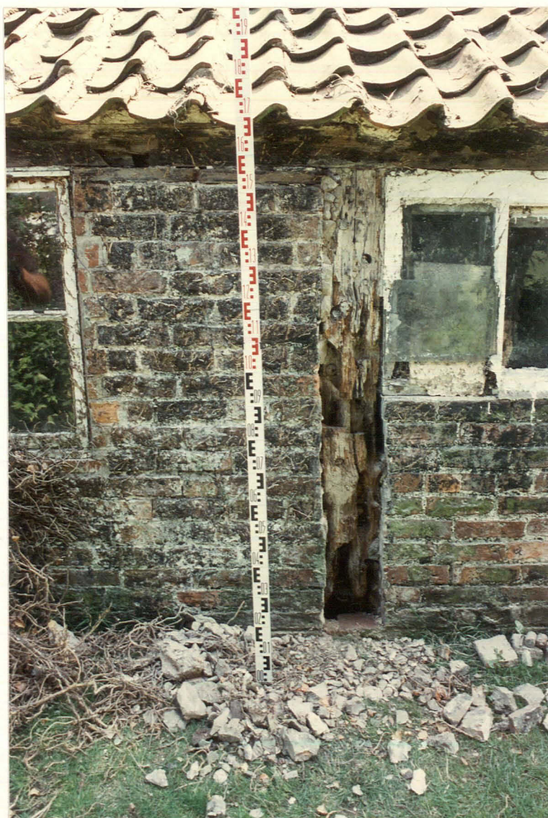
Pl. 41. Outshot north wall: sawn rails and braces.
