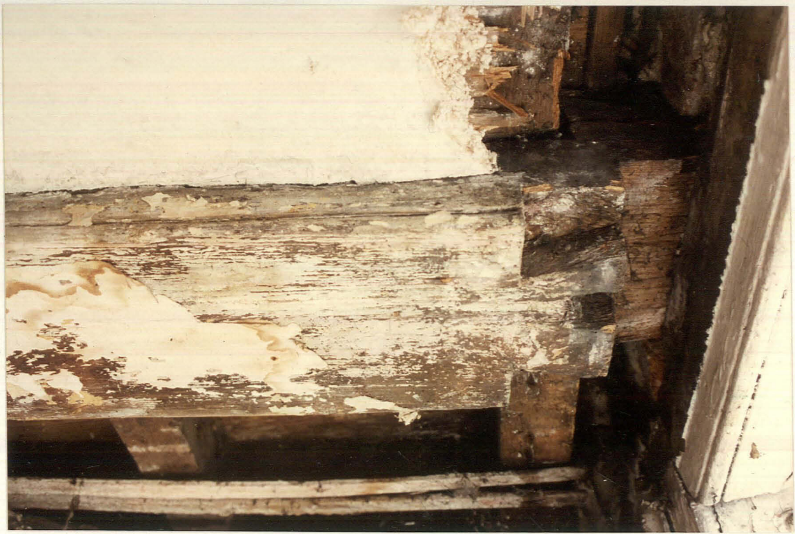
Pl. 45. West binder, south dovetail cut for ledging (parlour).
