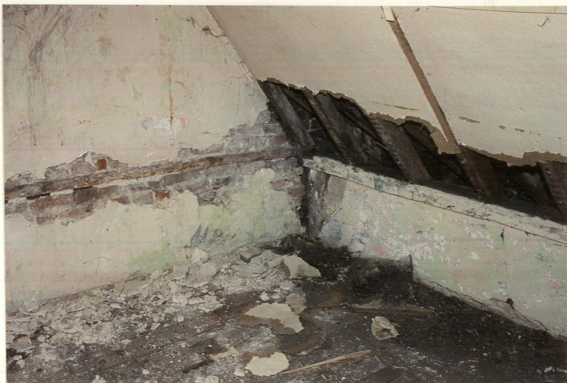
Pl. 50. Eaves plate and west gable tie; room 9, from south-east.
