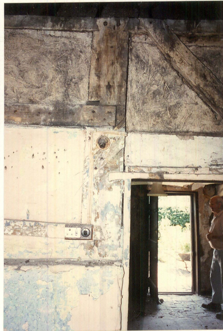
Pl. 30. East gable, clasp ing north-east corner of frame (plinth below), from west.
