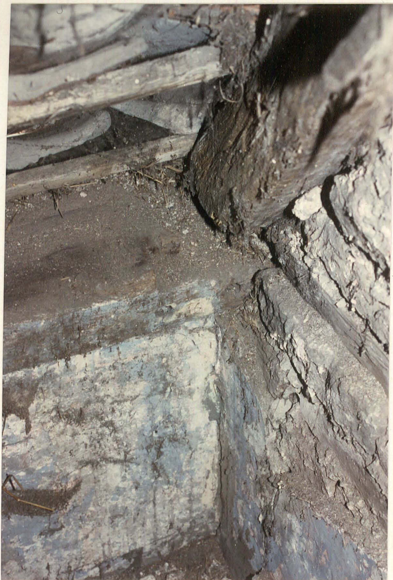
Pl. 52. South-west corner: plate and gable tie detail.
