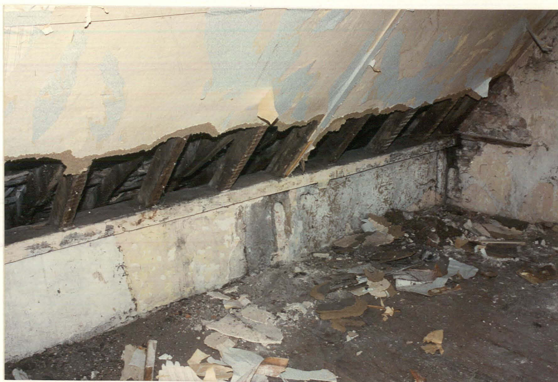
Pl. 51. Eaves plate and east gable tie; room 10, from south-west.
