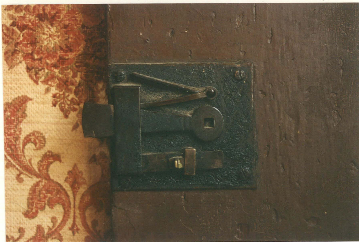
Pl. 14. Understair cupboard door latch.
