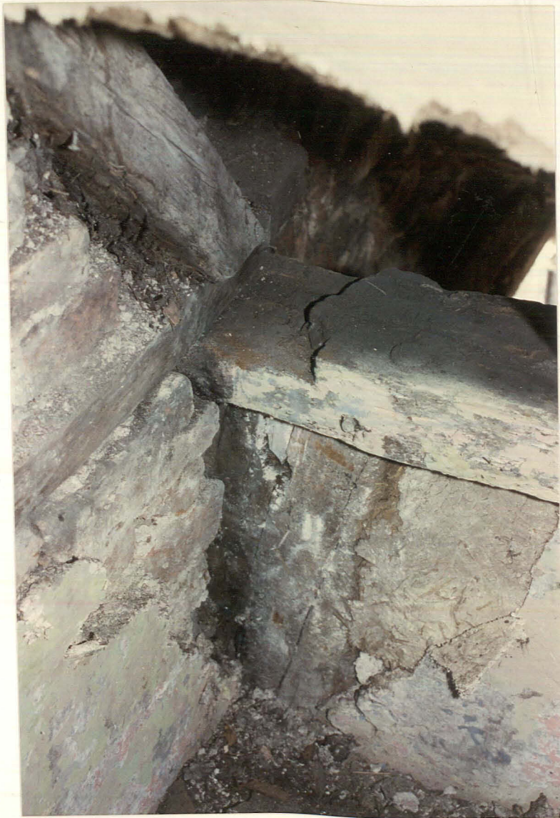
PI. 54. North-west corner: eaves plate and gable tie. Dovetail mortise.
