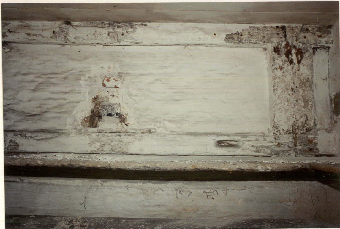
Pl. 34. North Wall-frame, kitchen/parlour brick partition visible in larder.
