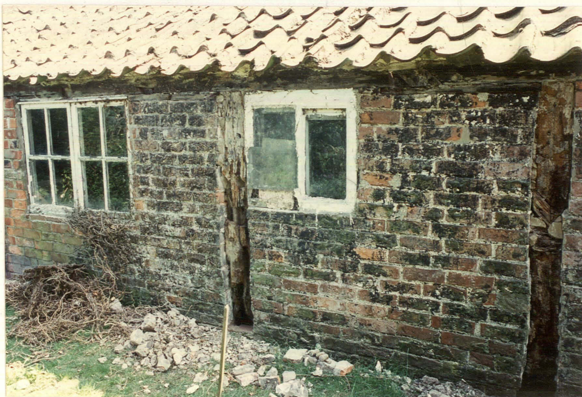
Pl. 40. Outshot north wall: exposed posts, from north.
