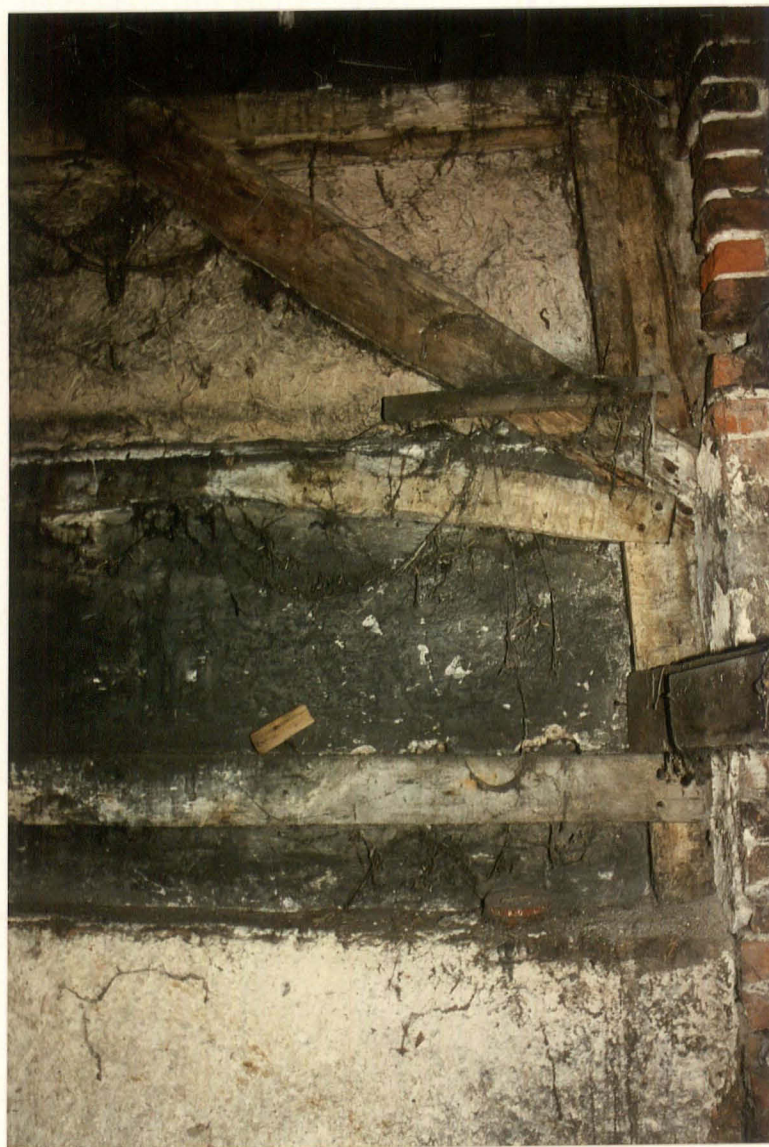
Pl. 36. West gable clasp and north-west corner post (plinth below), from north.
