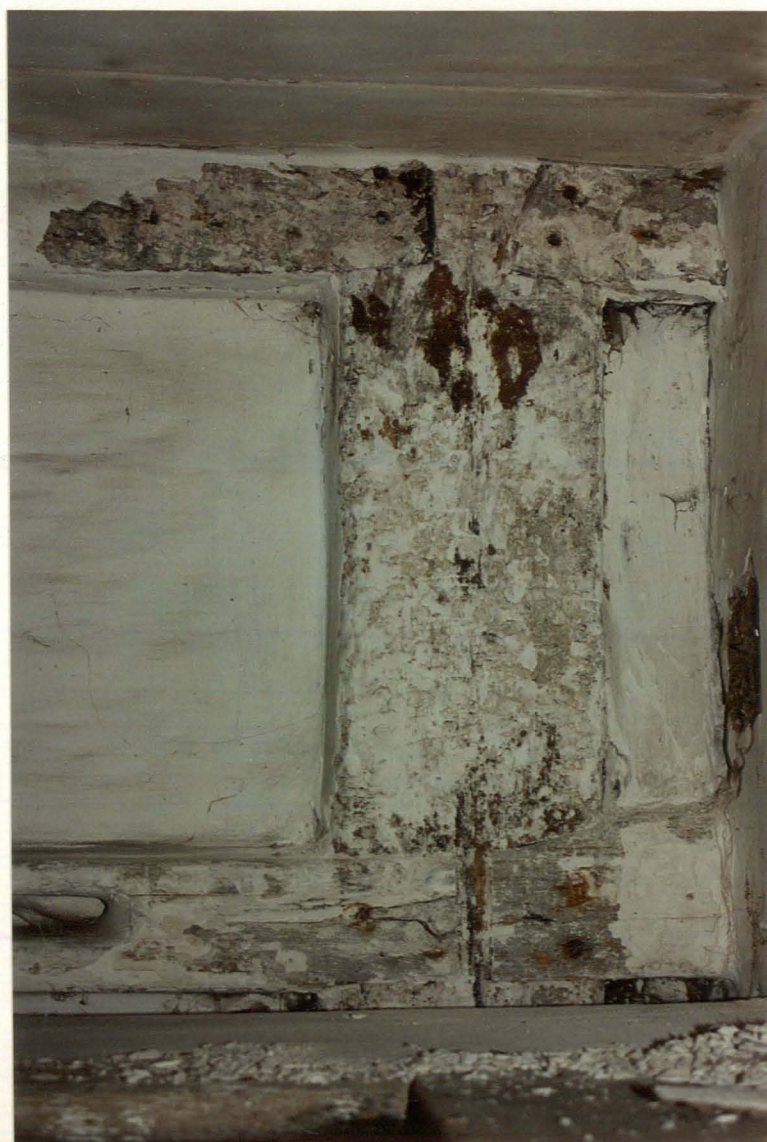
Pl. 35. North wall-frame, larder: Rail fixings.
