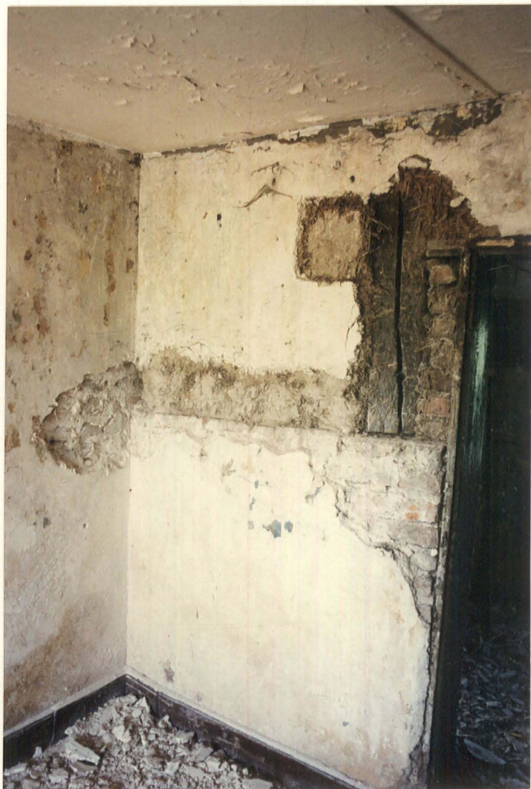
Pl. 47. Post and half-bricks on plinth wall in kitchen north wall.
