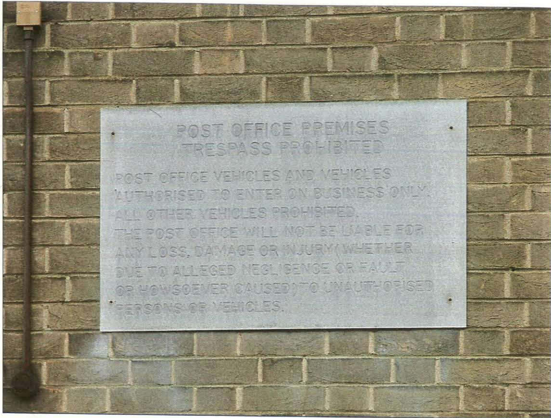
Plate 5. Post Office notice, north-west elevation
