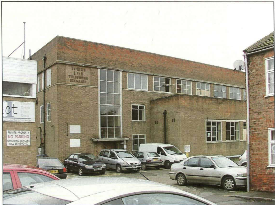
Plate 2. North-west (main) elevation as seen from Gore Lane
