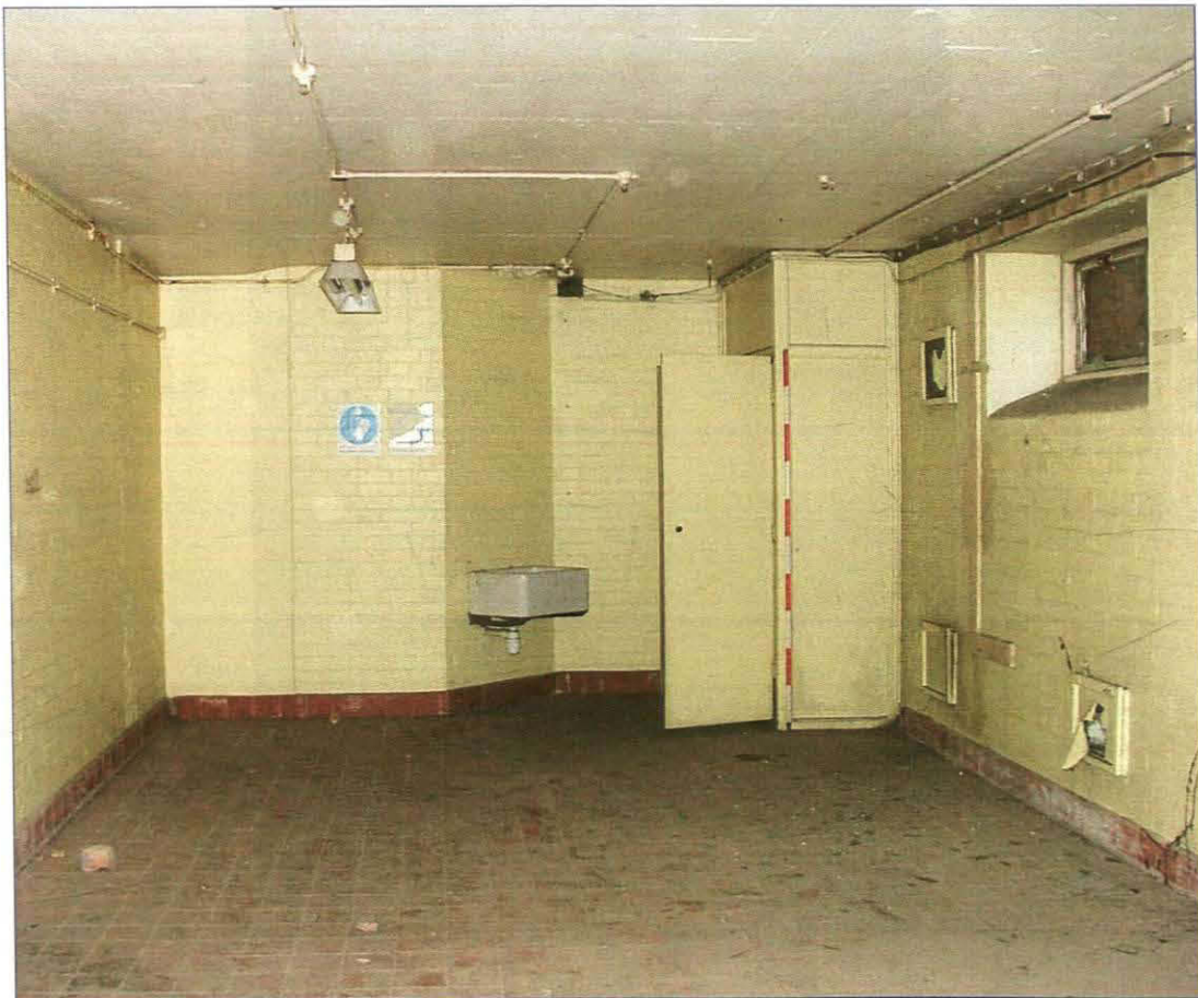
Plate 36. View looking north-east of the interior of the Battery Room (Scale = 2m)
