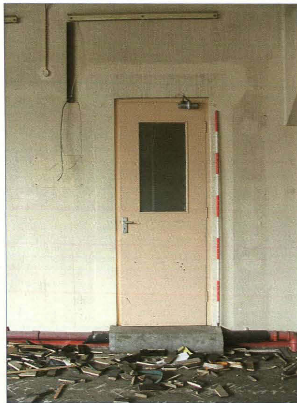
Plate 34. Door at north-east end of ground floor large hall (Scale = 2m)
