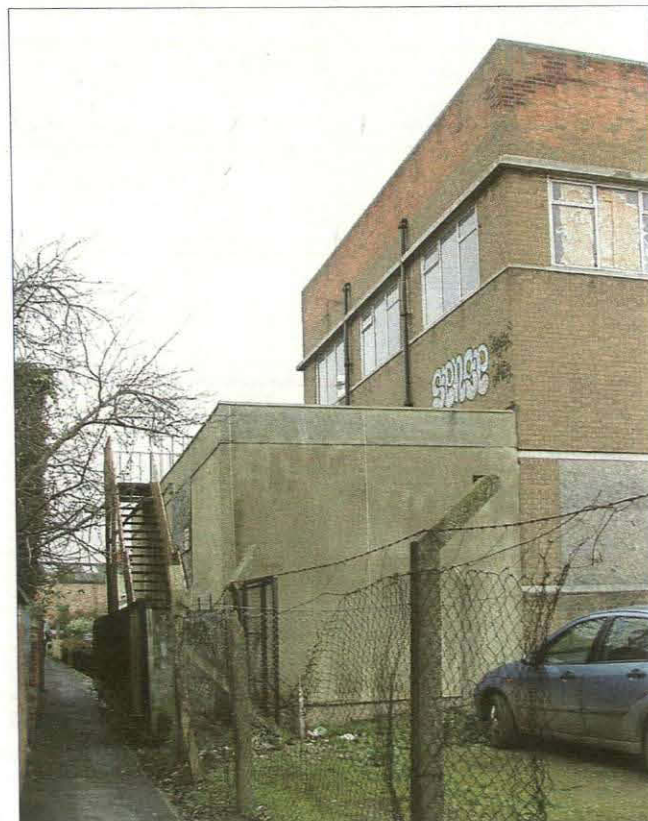
Plate 14. View from Abbey Path showing the single-storey extension against the south-west elevation
