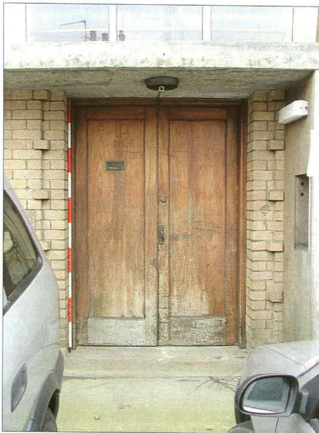
Plate 6. Main entrance into the telephone exchange (Scale = 2m)
