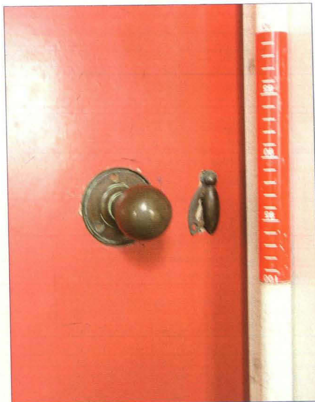
Plate 38. Detail of door knob and lock, first floor
