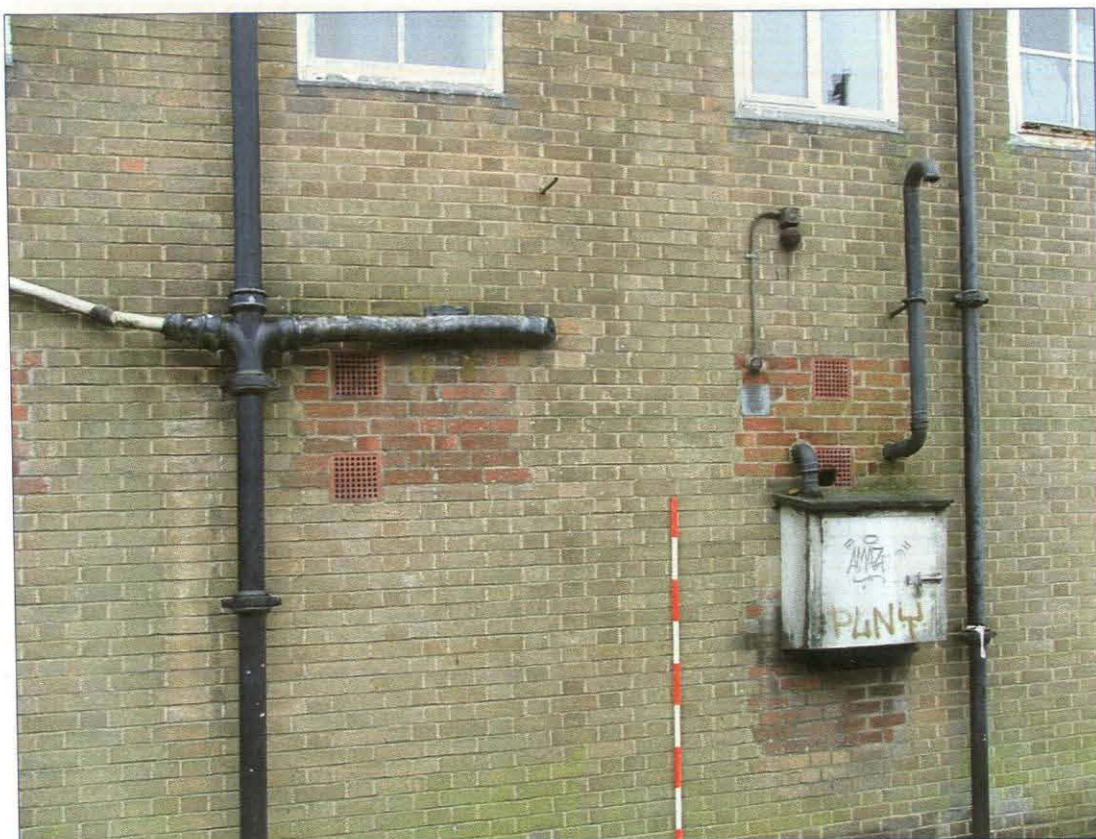
Plate 11. Detail of bricked-up holes in north-east elevation (Scale = 2m)
