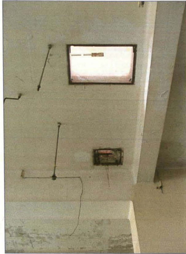
Plate 33. Square holes in the ceiling of the ground floor hall
