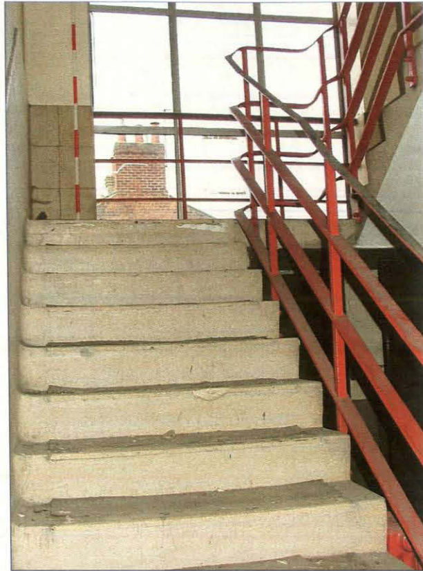
Plate 21. Detail of metal handrail and balusters of staircase
