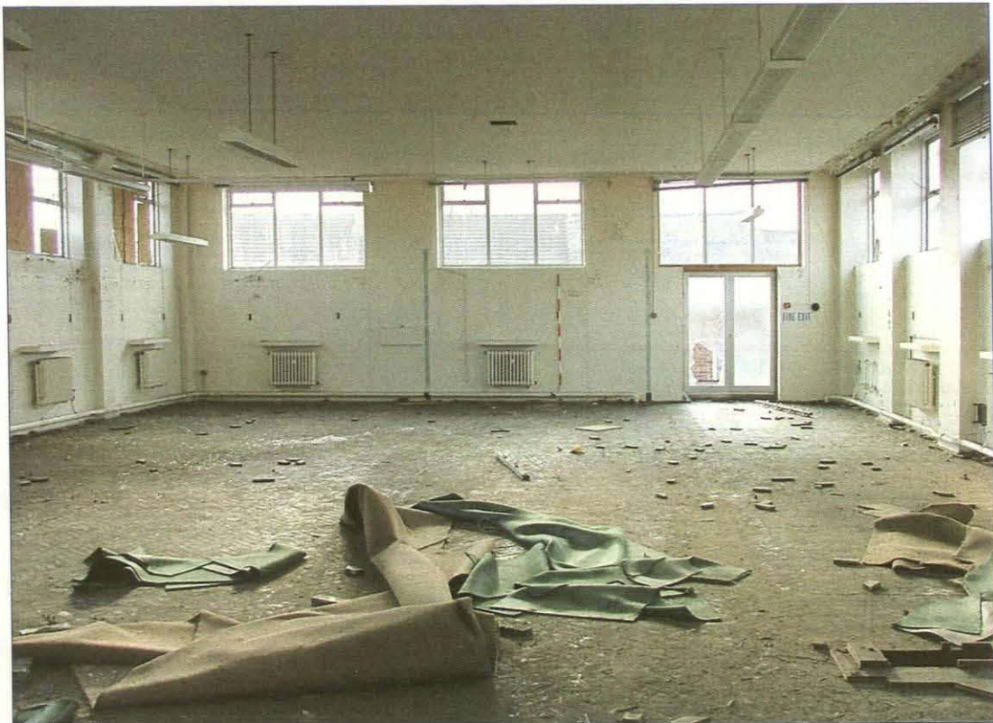
Plate 42. View looking south-west of the Operating Room (Scale = 2m)
