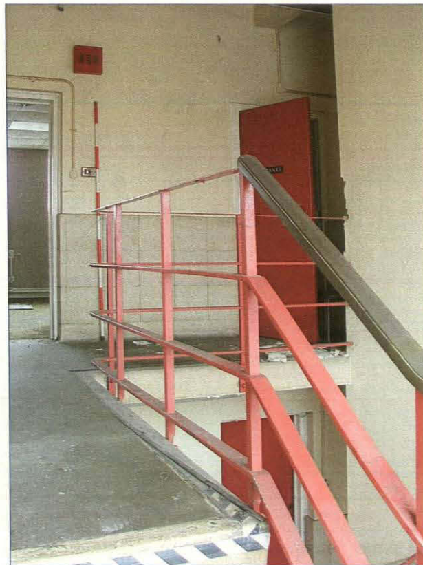
Plate 22. Detail of staircase at second floor level showing surviving section of brass handrail (Scale = 2m)
