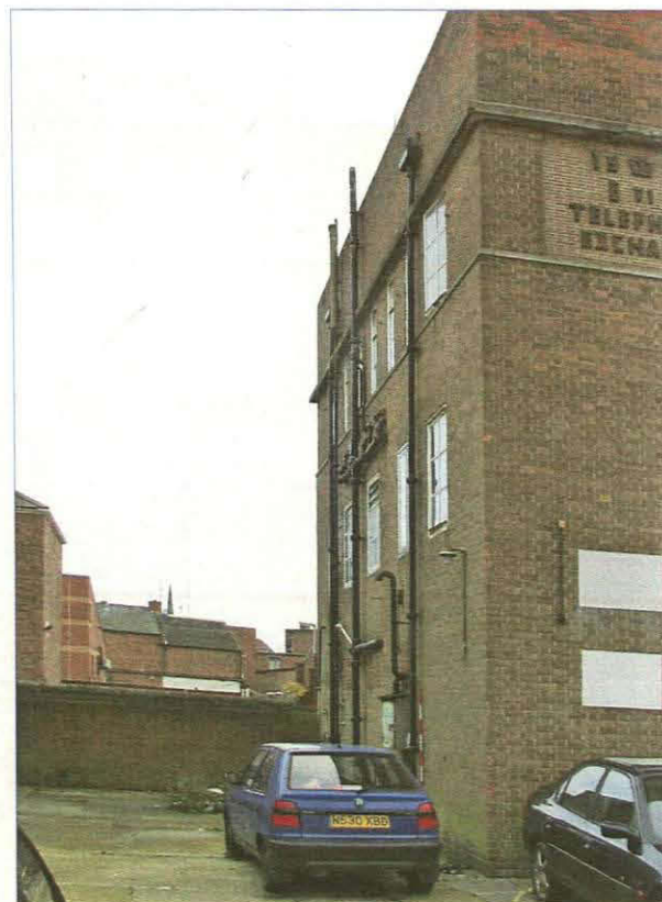
Plate 10. View looking south-east of the north-east elevation
