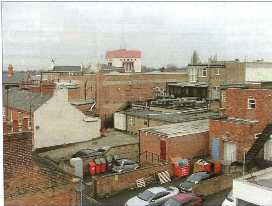
Plate 53. View looking north towards the water tower on Kings Road 5
