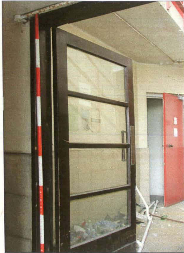
Plate 17. Door to stairwell from main entrance (Scale = 2m)
