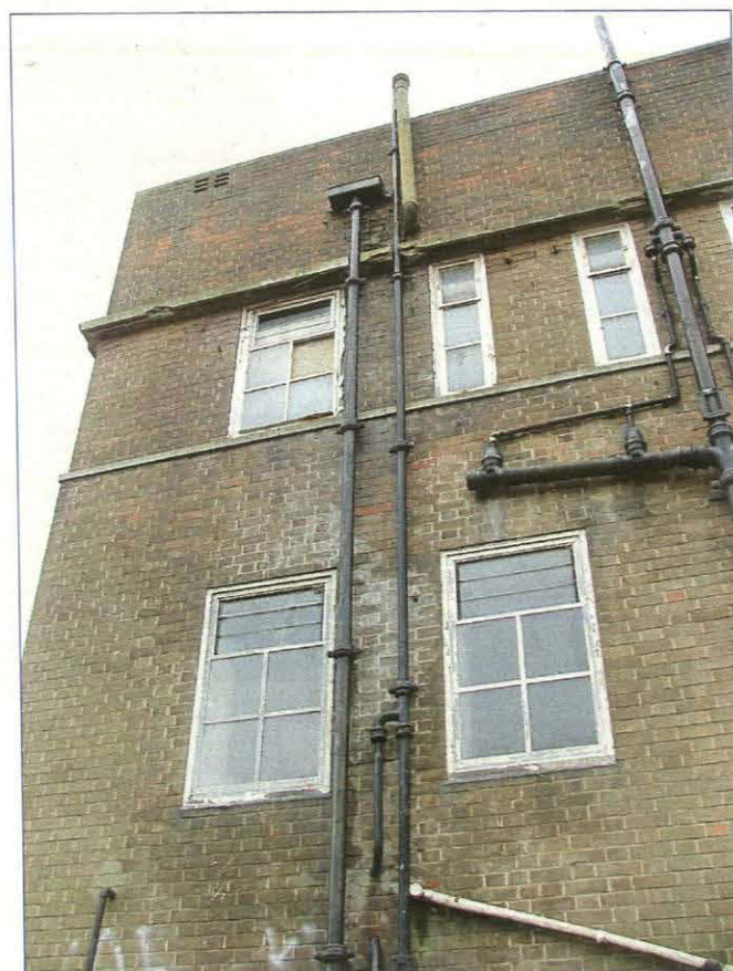
Plate 12. Detail of windows at first and second floor level, north-east elevation
