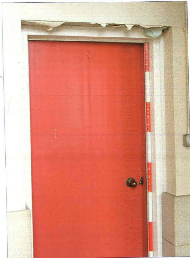
Plate 37. Door to the Retiring Room (No.9) (Scale = 2m)
