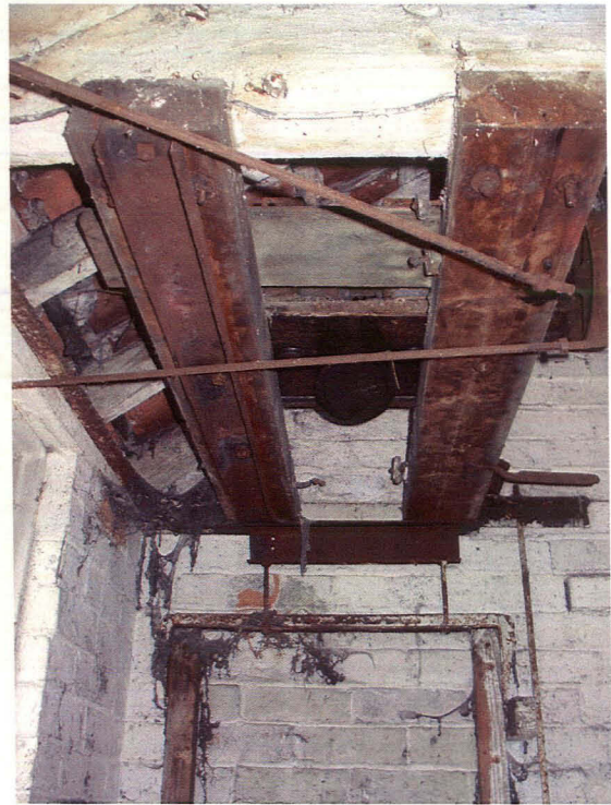
Plate 13 Girder supports for overhead generator, looking SW
