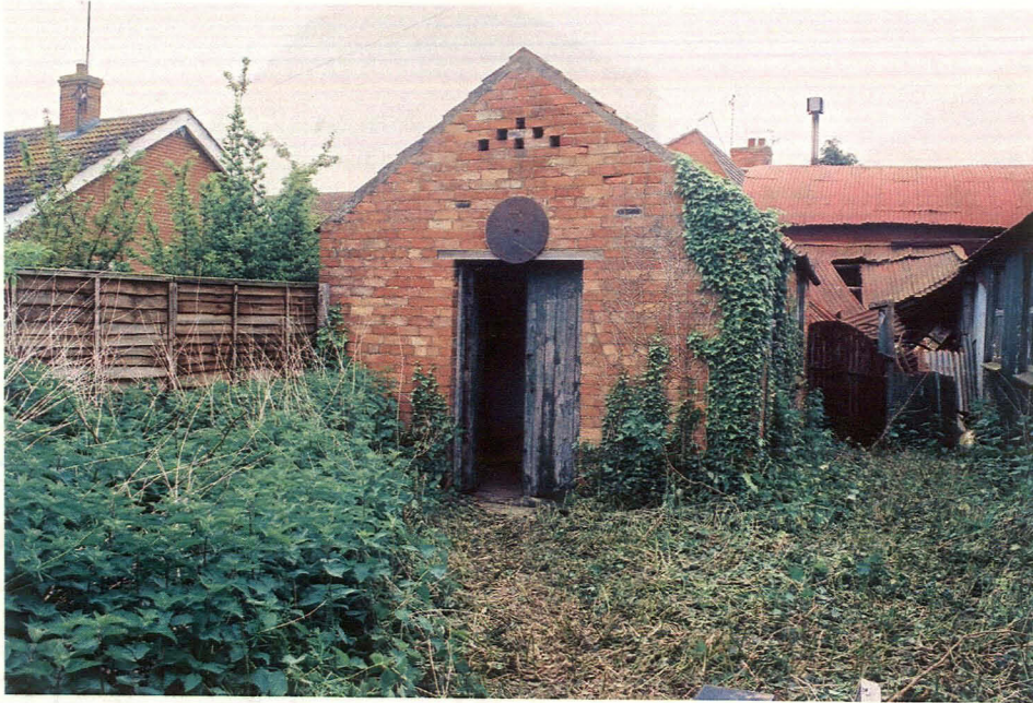
Plate 1 WSW elevation of recorded structure, looking ENE
