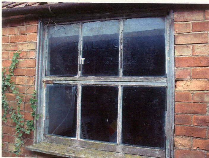
Plate 7 Detail of wooden framed windows, looking SSE
