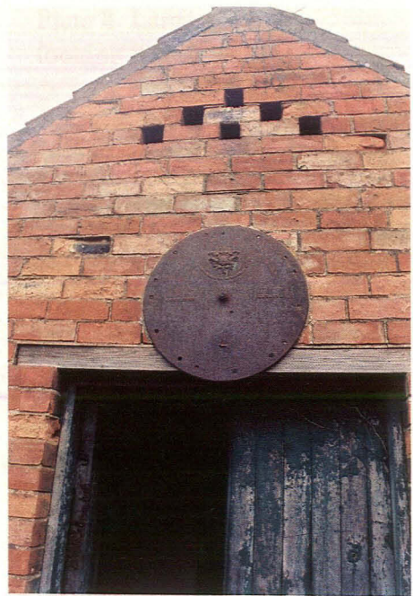
Plate 5 Detail of ventilation gaps and Tie Bar Plate, looking ENE
