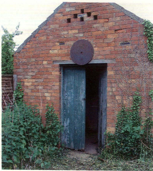
Plate 4 WSW elevation showing wooden door, ventilation gaps and Tie Bar Plate, looking ENE
