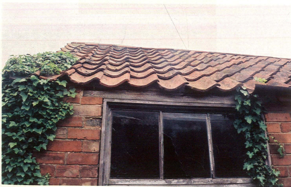
Plate 3 Detail of pantile roof, looking NNW
