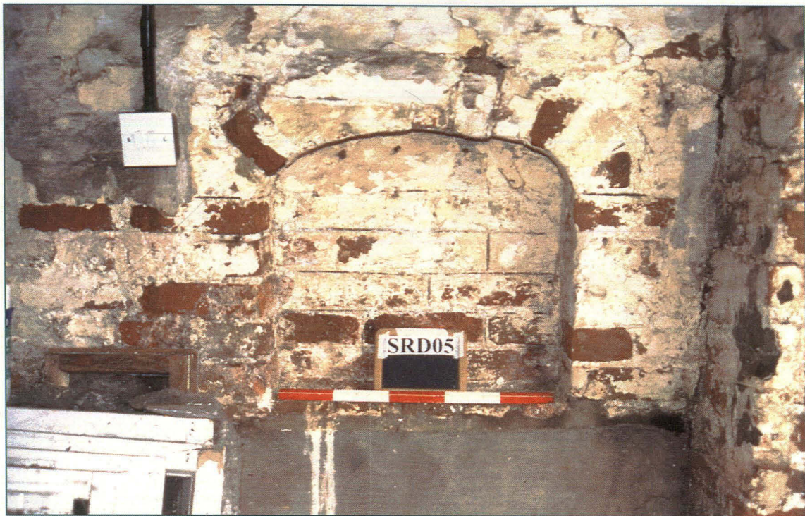
Pl. 9: Arched recess in north wall of Room C. Looking north.
