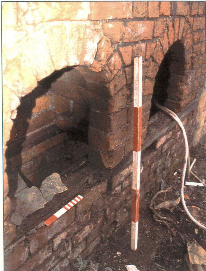
Pl. 19: Detailed view of arches. Note the interior corbelling of the structures and the gap allowing access between the two arches. Looking north-west
