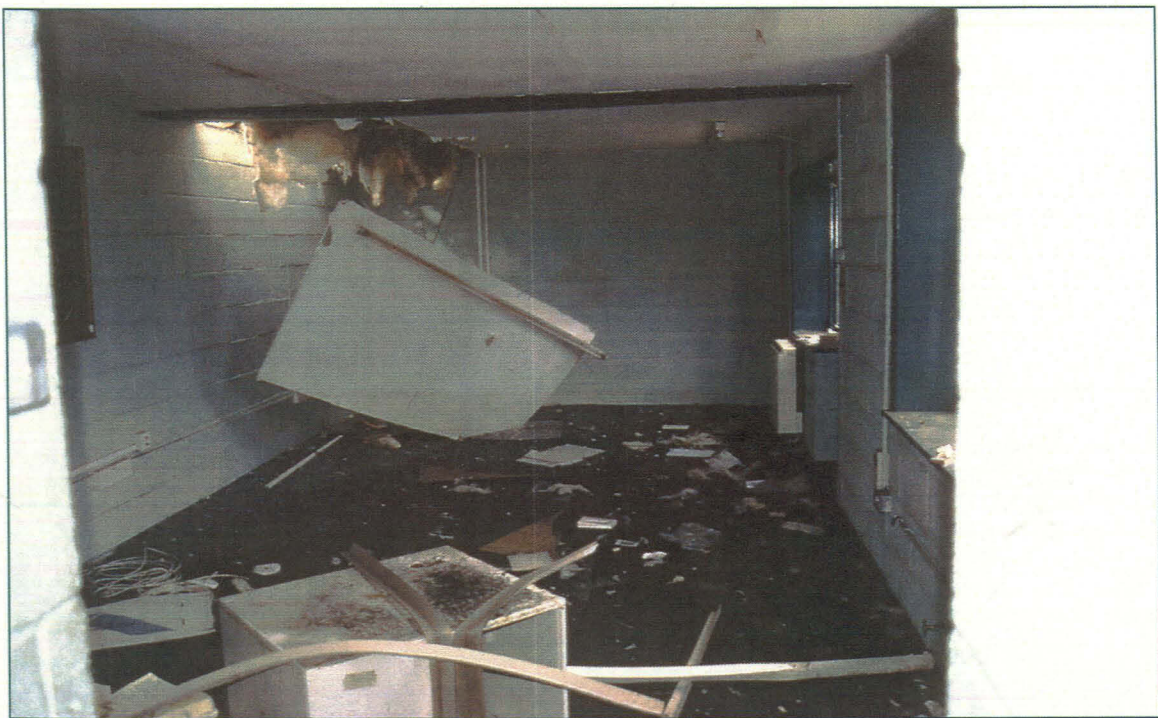
Pl. 12: Room E, showing breeze block rebuilding and suspended ceiling. Looking north.
