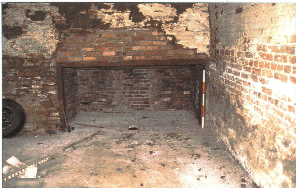
Pl. 10: Possible loading bay in west wall of Room D, looking west
