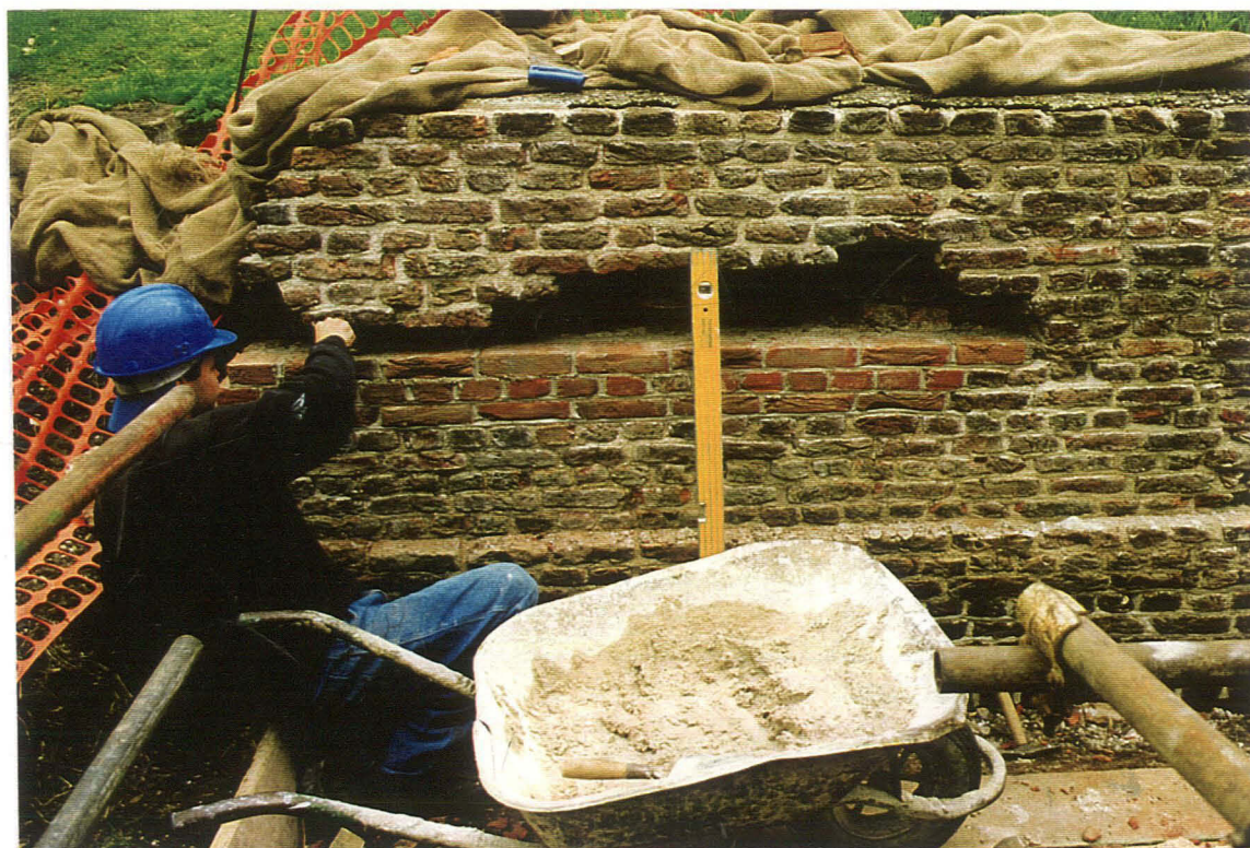
Pl. 7 Elevation A , east half, new brickwork
