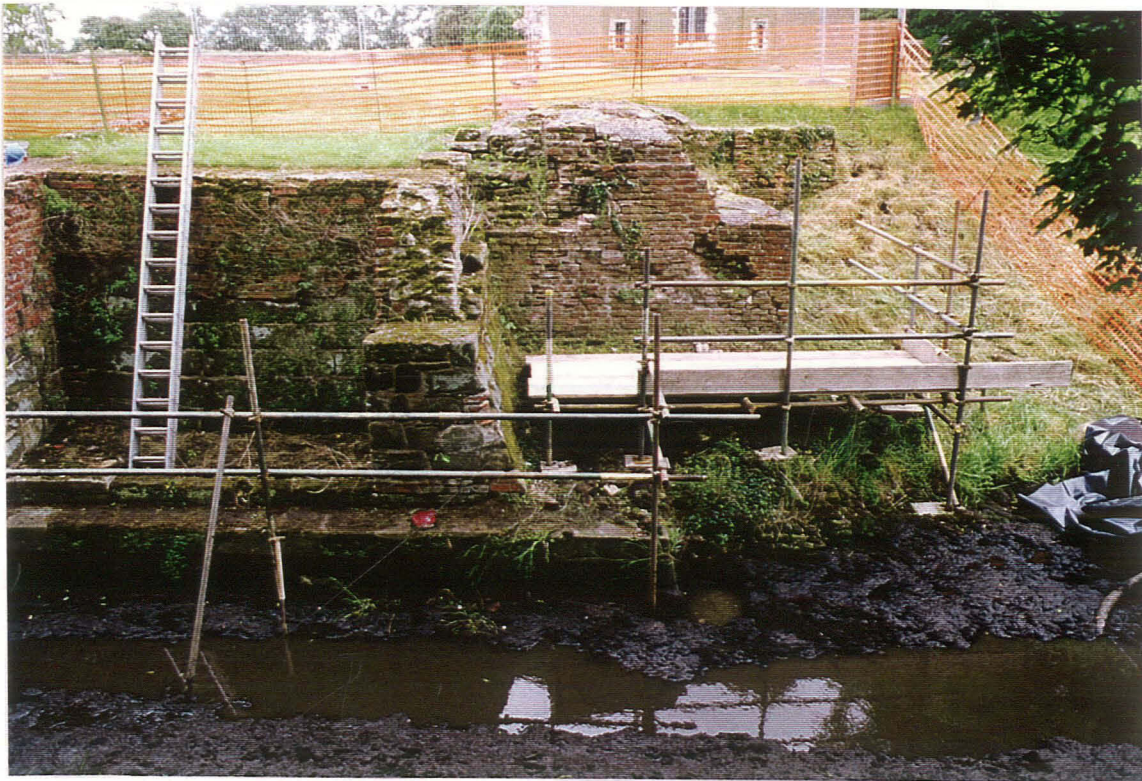
Pl. 10 General view of elevations E-K prior to cleaning
