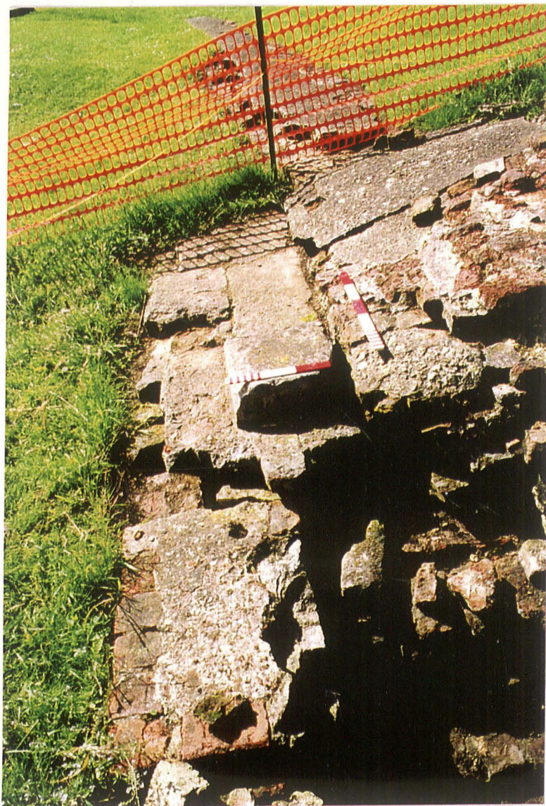
Pl. 32 Junction of walls extending from elevations F and K showing straight joint (X), with wall Y in background, looking south. Scales 0.50m and 0.30m
