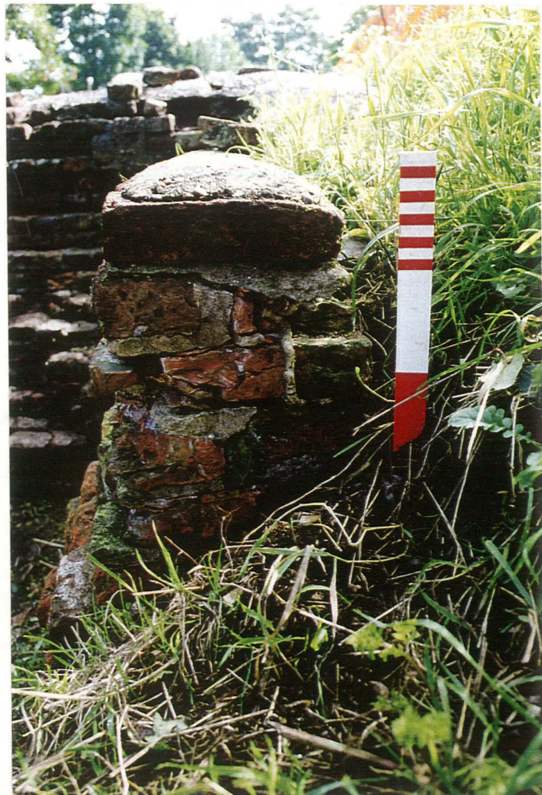
Pl. 31 Side view of Elevation K, looking east. Scale 0.30m
