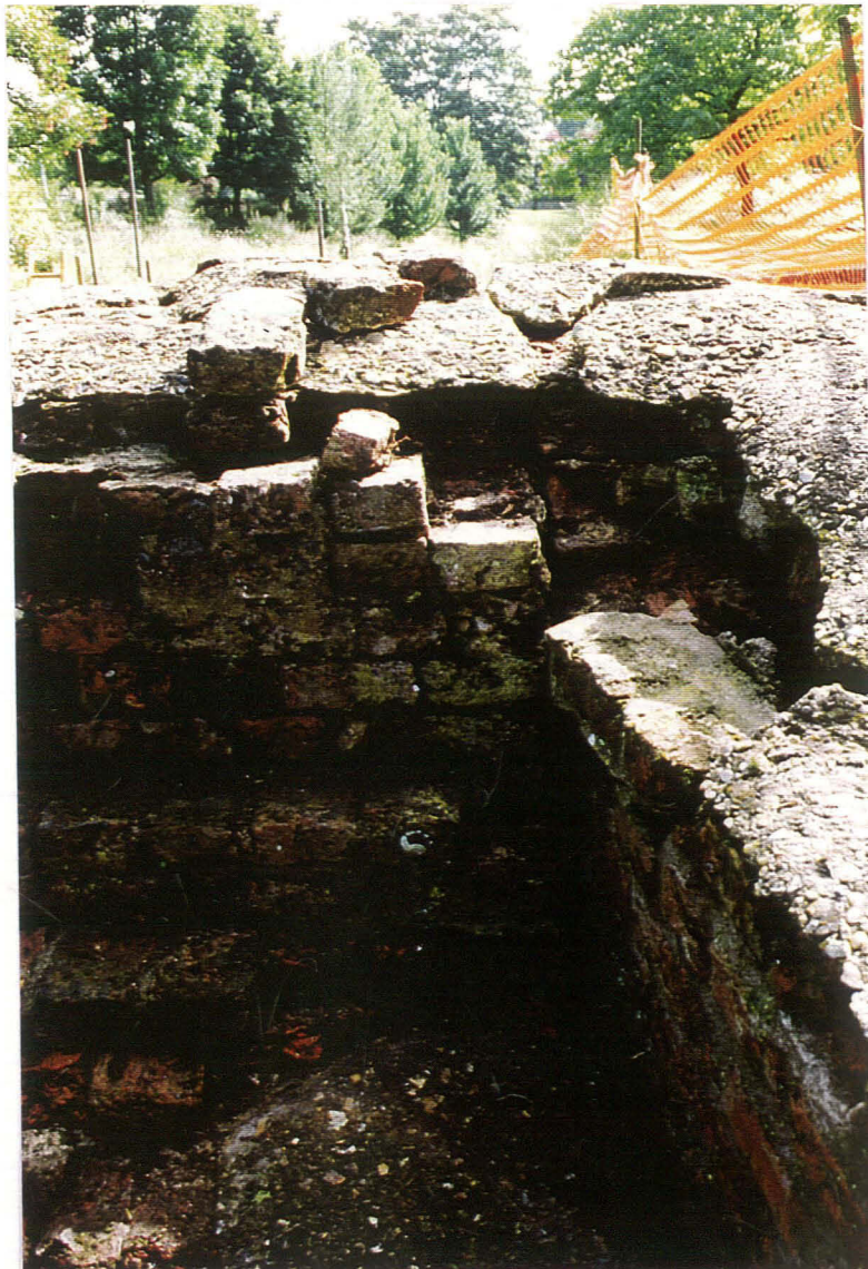
Pl. 29 Elevation J at junction with Elevation K, showing straight joint
