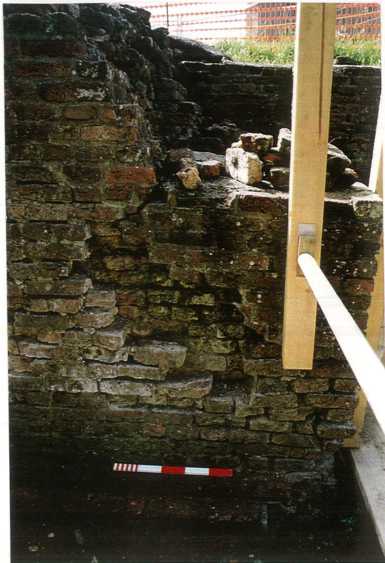
Pl. 24 Elevation I, west half, after cleaning. Scale 0.50m
