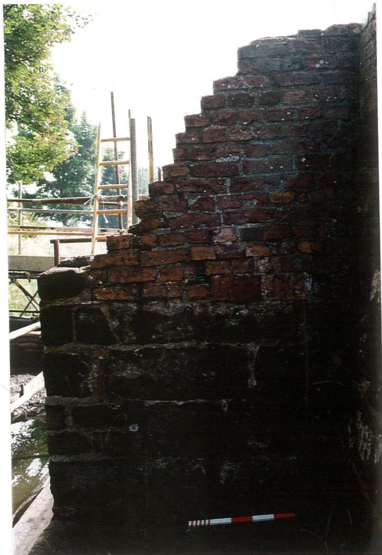
Pl. 15 Elevation D after cleaning. Scale 0.50m
