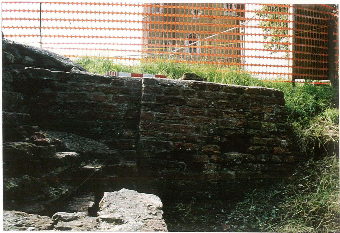
Pl. 30 Elevation K after cleaning, showing straight joint. Scale 0.50m
