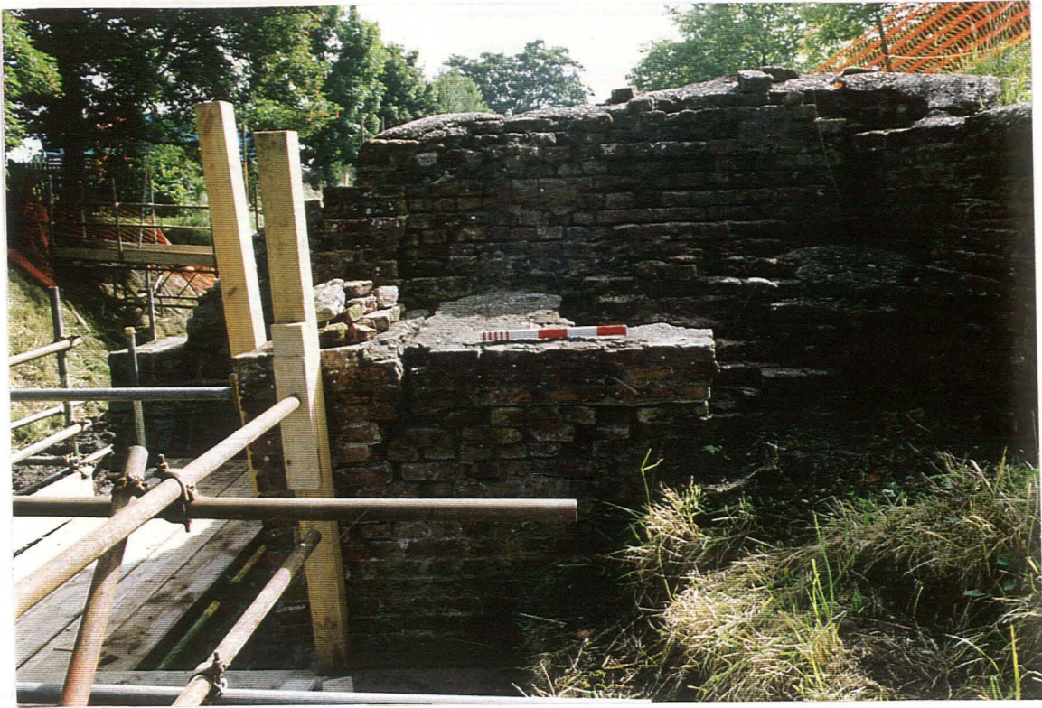
Pl. 28 Elevation J after cleaning. Scale 0.50m
