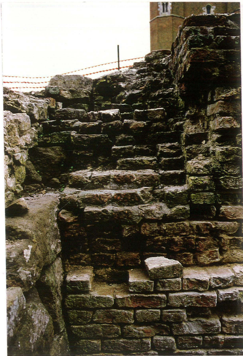
Pl. 22 Elevation I at junction with Elevation H, after raking out
