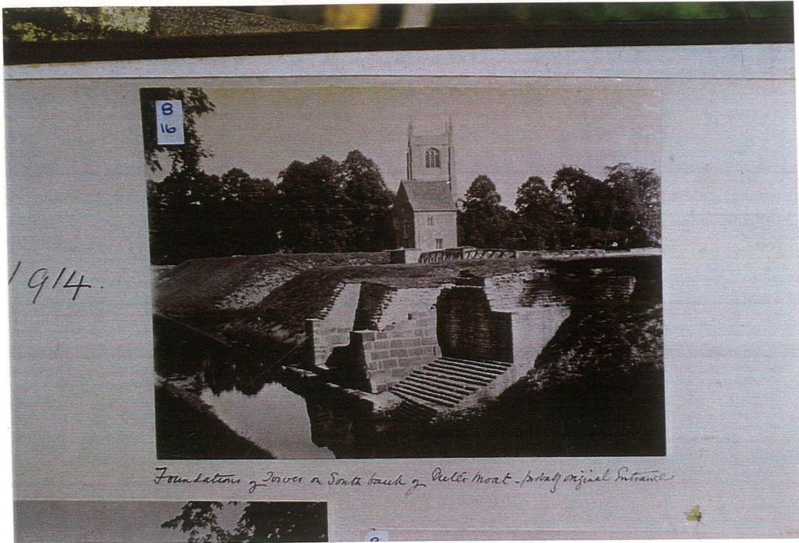
Pl. 1 General view of gatehouse after repairs in 1914. Copy of photo in album held at the Castle.
