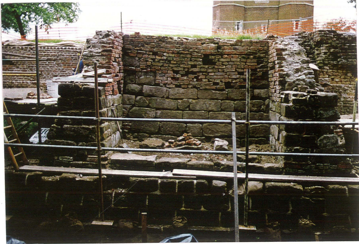
Pl. 14 Elevations C, E, G after raking out
