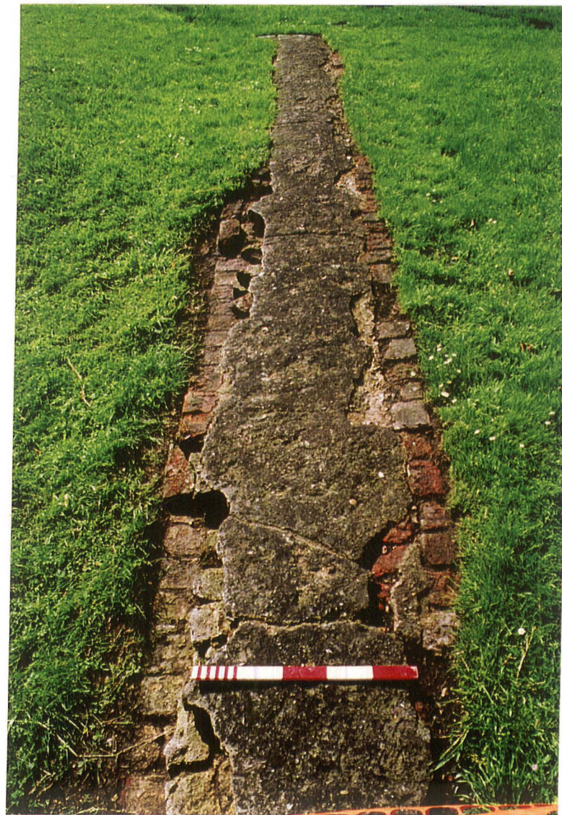
Pl. 32 Junction of walls extending from elevations F and K showing straight joint (X), with wall Y in background, looking south. Scales 0.50m and 0.30m
