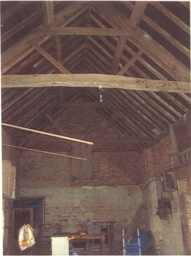
Plate 13 - Interior view of the barn showing doorways to the stable and granary
