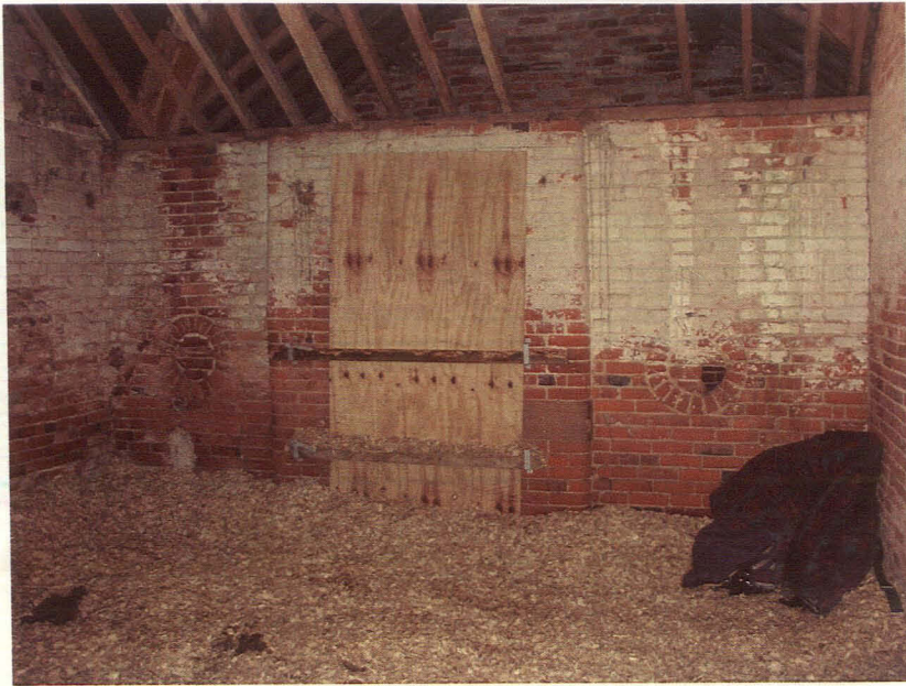
Plate 16 - View of the interior of the east room of the north range, showing the circular brick recesses
