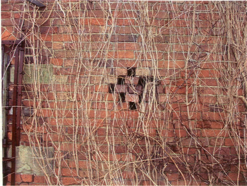
Plate 4 - View showing honey-combed brickwork ventilation
