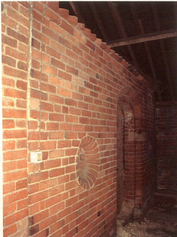
Plate 5 - View of the north range at the eastern end showing decorative brickwork and straight join to barn
