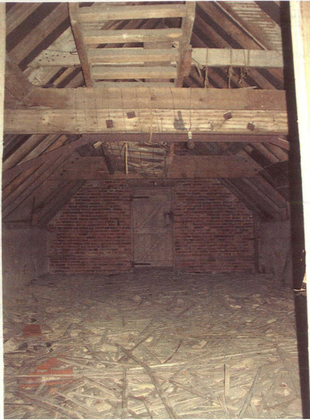
Plate 14 - Interior view of the first floor granary looking east
