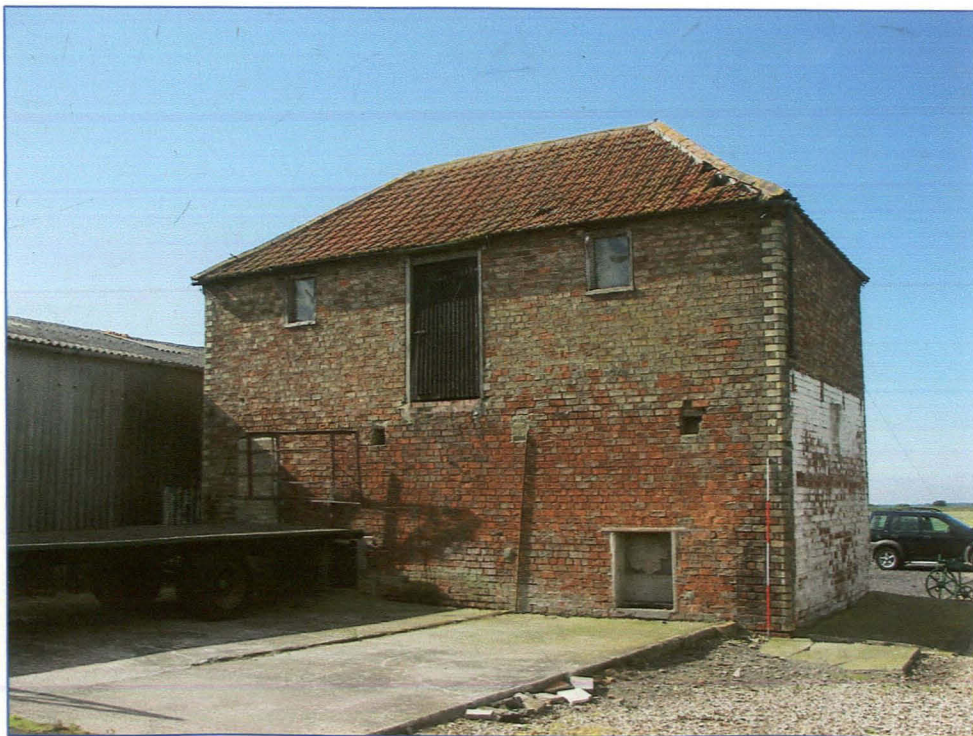
Plate 6 ( Shot 11): The north-east facing elevation viewed looking south. Note the concrete apron for the pig sties formerly accessed through the small openings in the barn wall.
